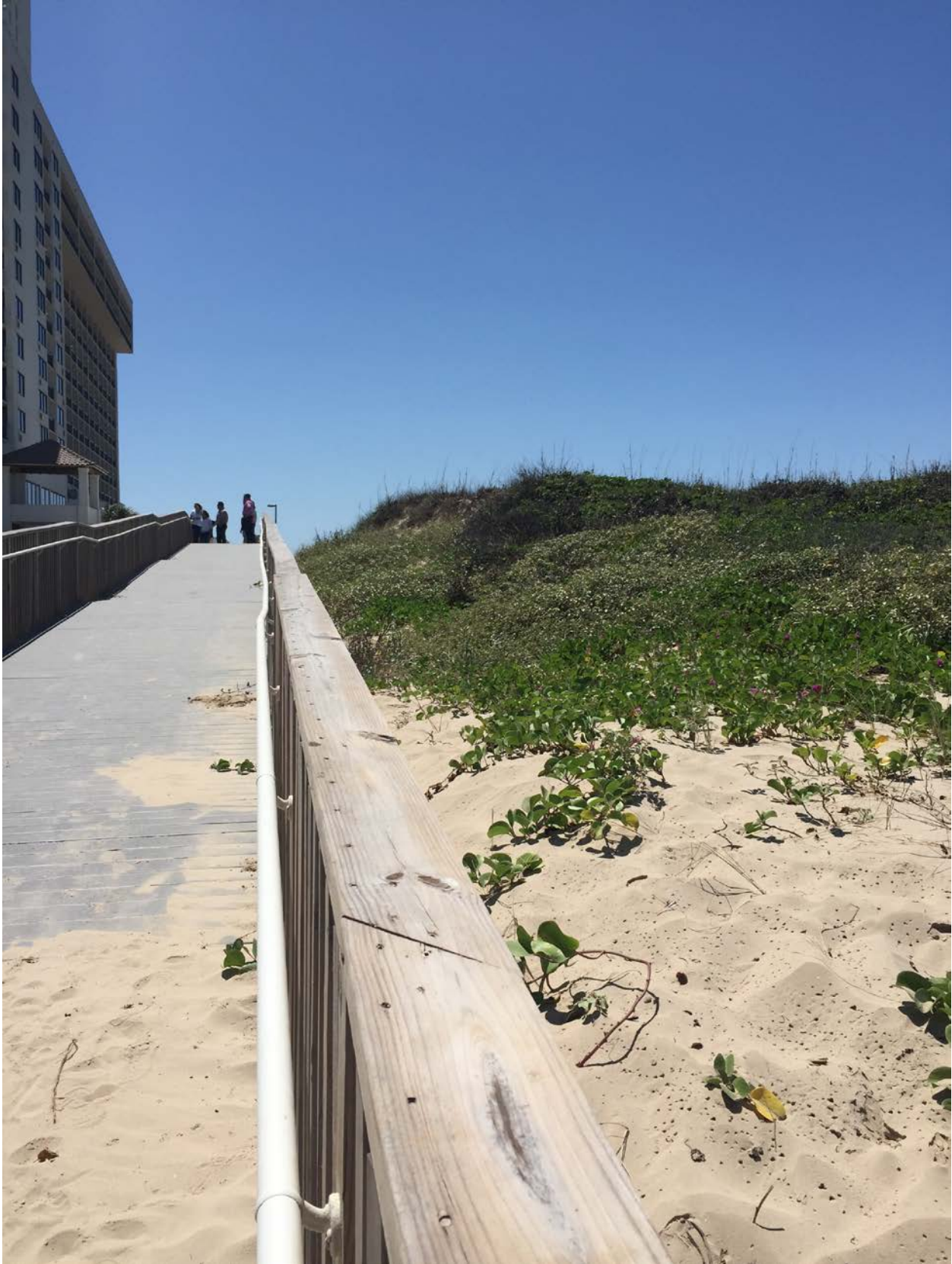
Figure 4. Photo of constructed dune walkover and mitigated dune
