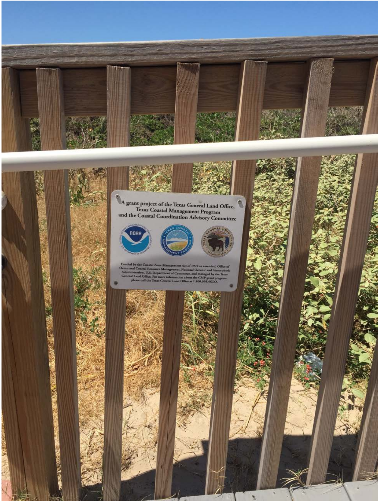
Figure 5. Photo of installed CMP signage
