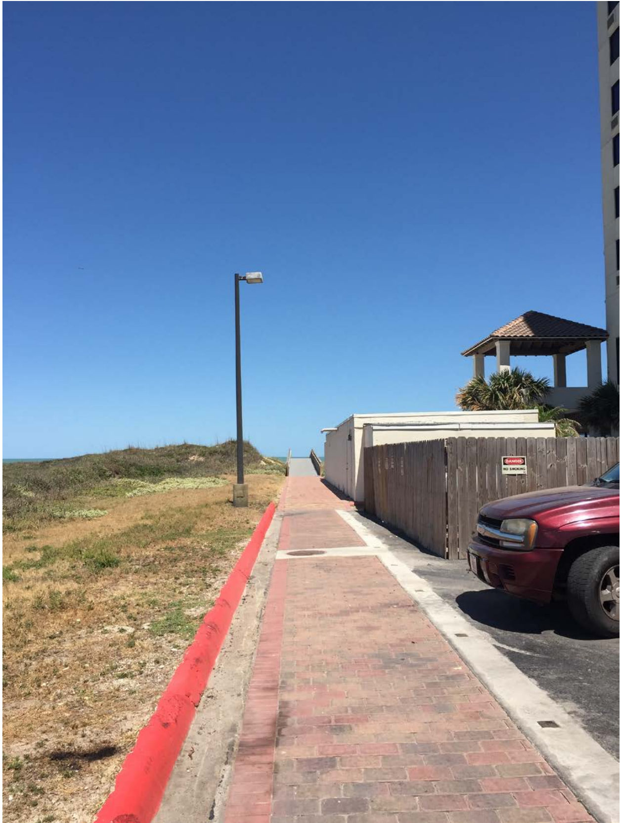
Figure 1. Photo of beach access walkway after construction
