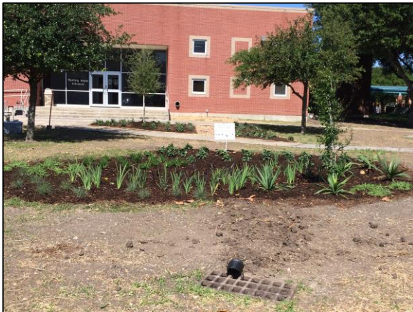
Rain garden site after installation
