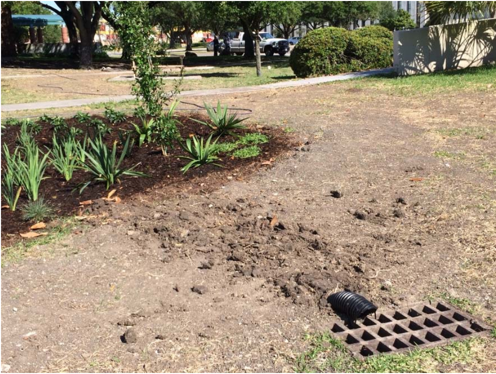
The perforated underdrain pipe runs along the bottom of the rain garden the connects to the storm drain system
