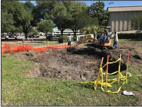
City of Pasadena workers digging the rain garden
