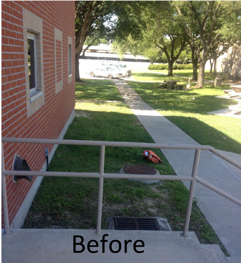
The pipe on the left is the water source for the rain garden.
