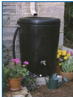
Rainwater harvesting system
