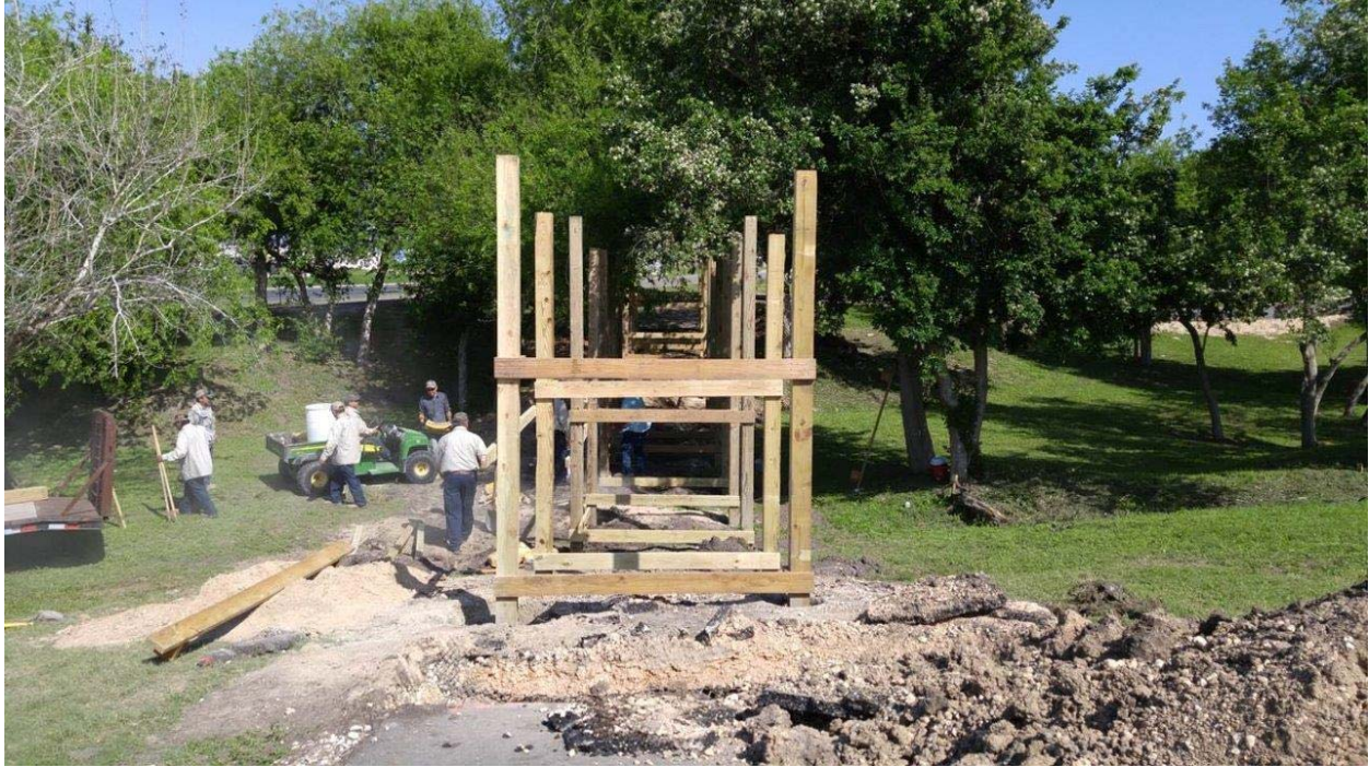
Figure 10. Nature bridge during construction
