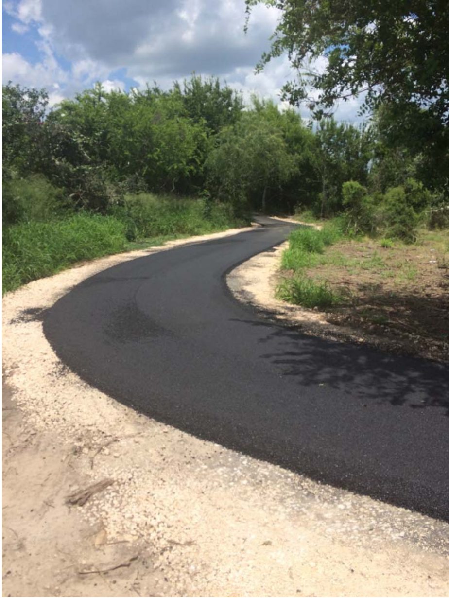
Figure 16. Nature trail after construction
