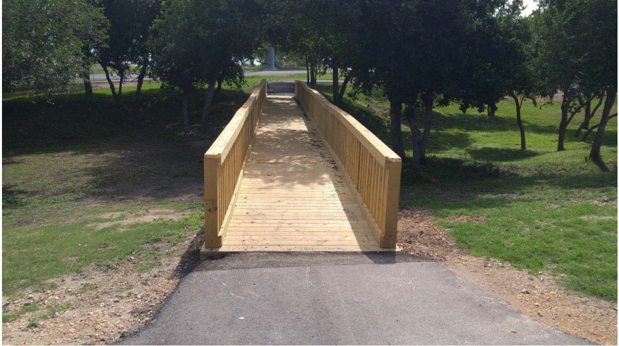
Figure 18. Nature bridge after construction
