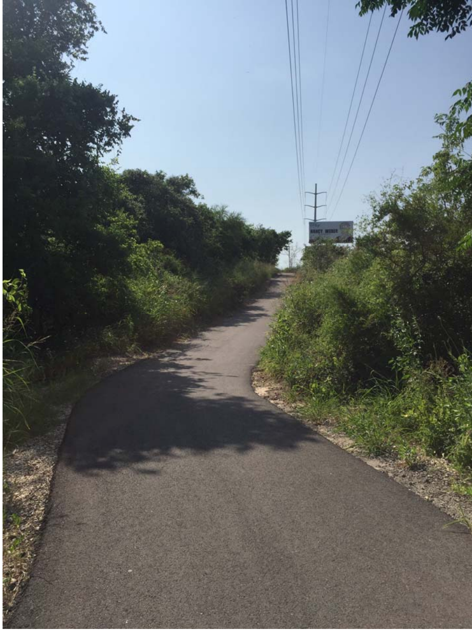
Figure 15. Nature trail after construction
