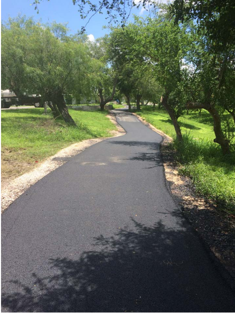
Figure 17. Nature trail after construction
