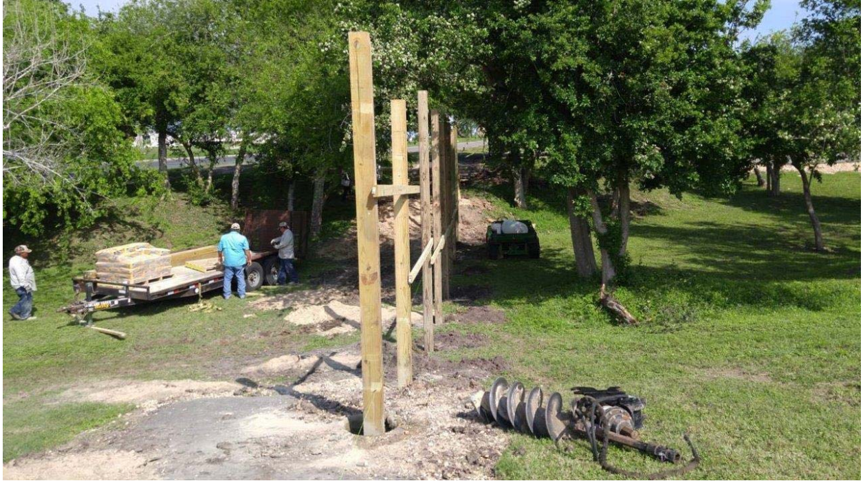
Figure 9. Nature bridge during construction
