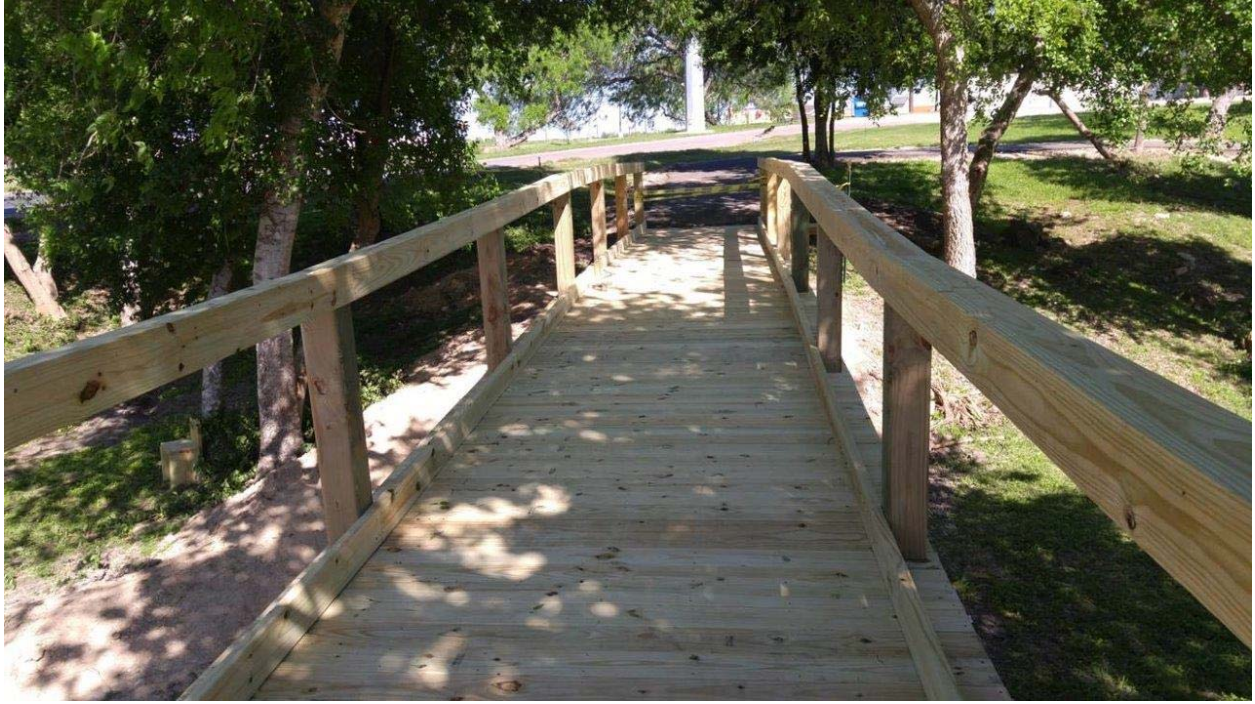
Figure 13. Nature bridge during construction
