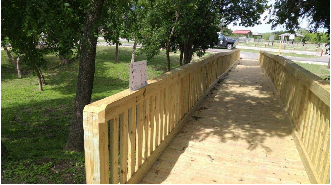
Figure 19. Nature bridge after construction
