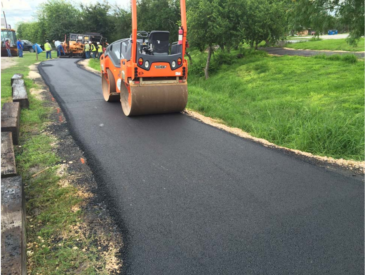
Figure 7. Nature trail during construction
