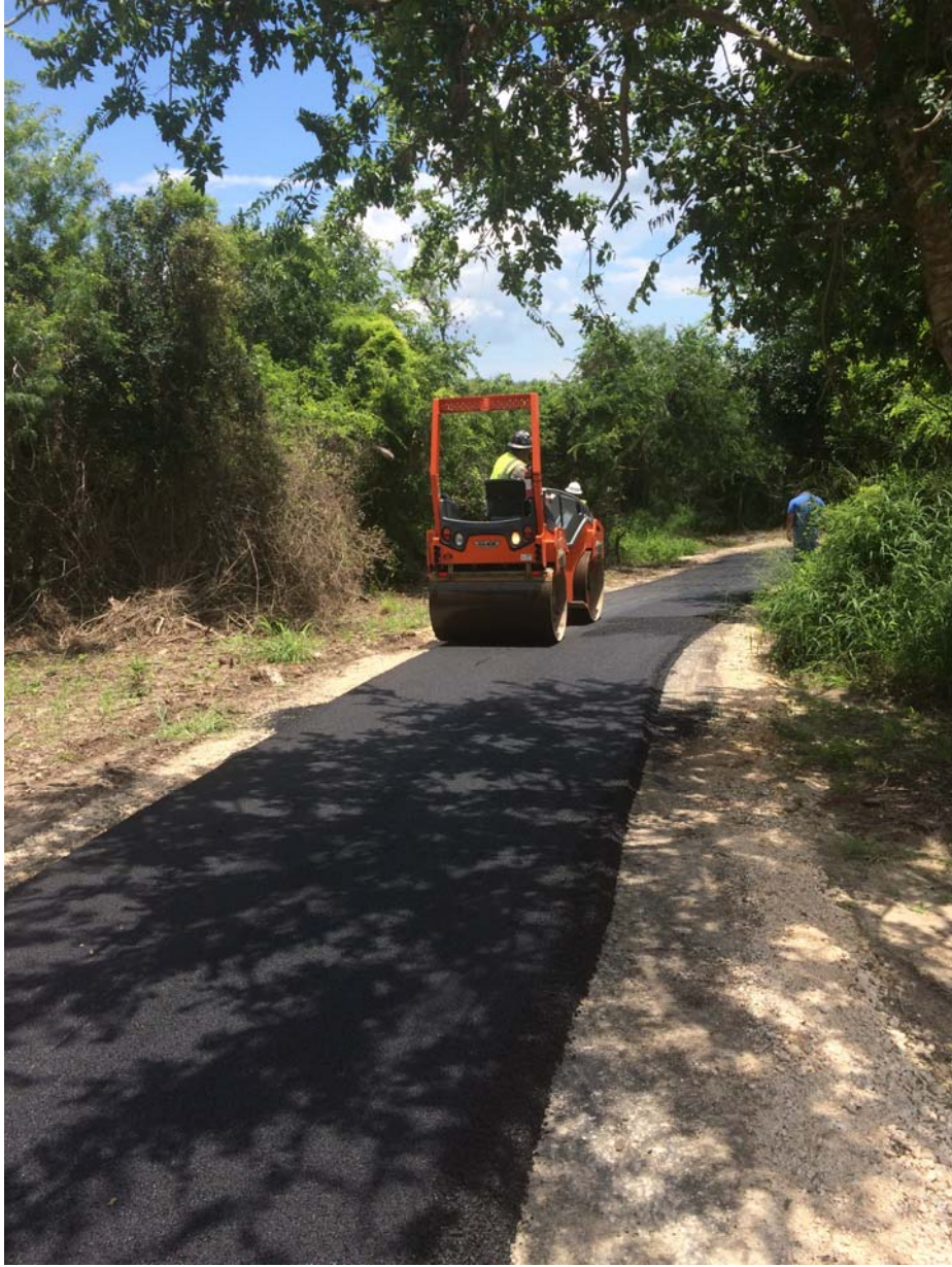
Figure 8. Nature trail during construction
