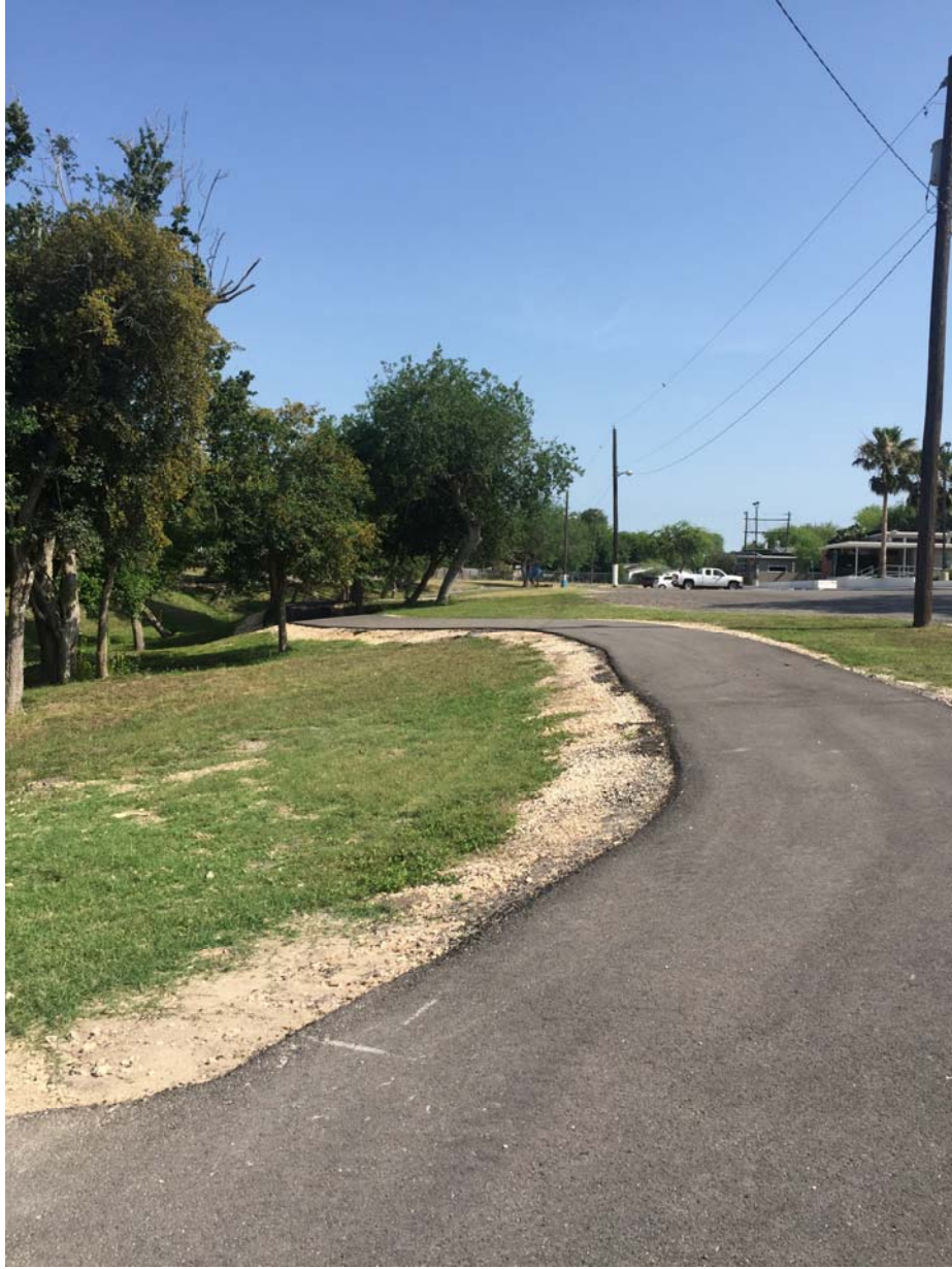
Figure 14. Nature trail after construction
