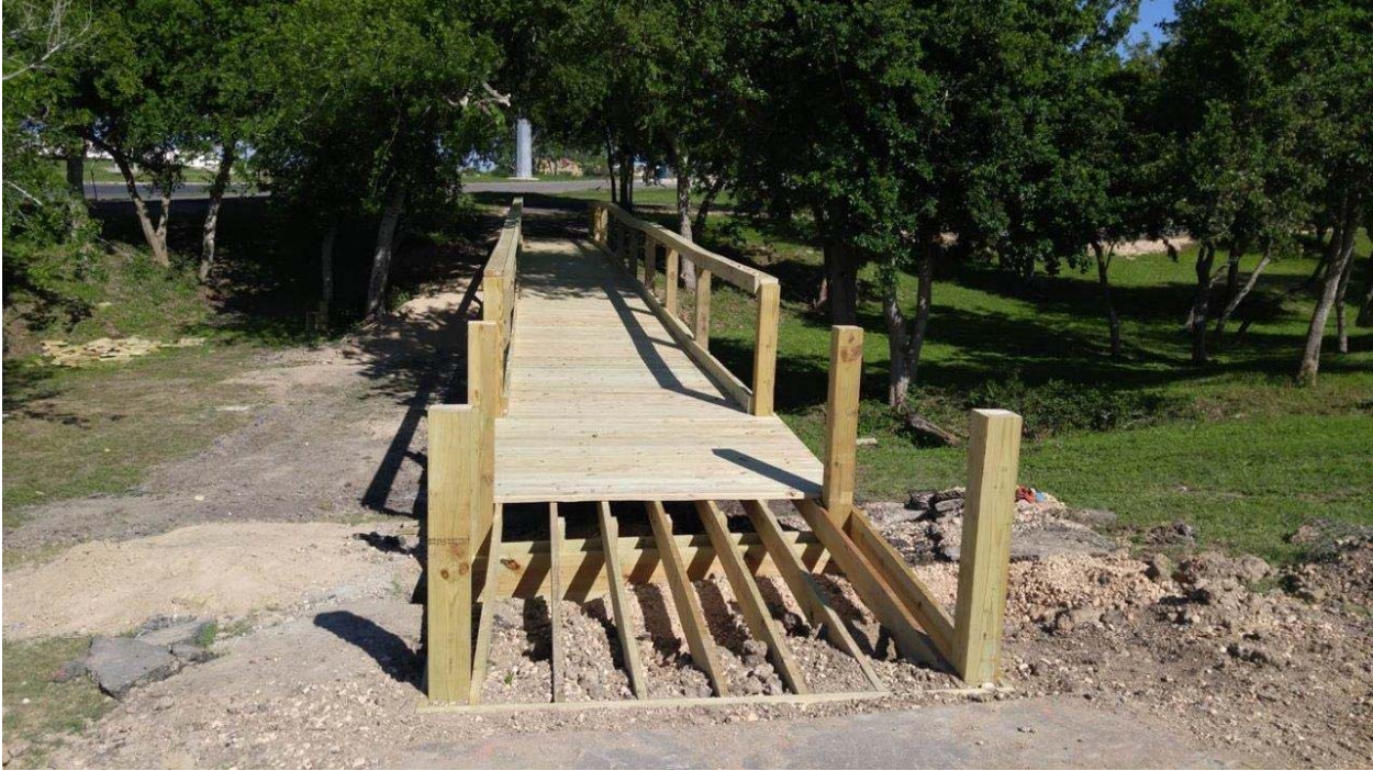
Figure 12. Nature bridge during construction
