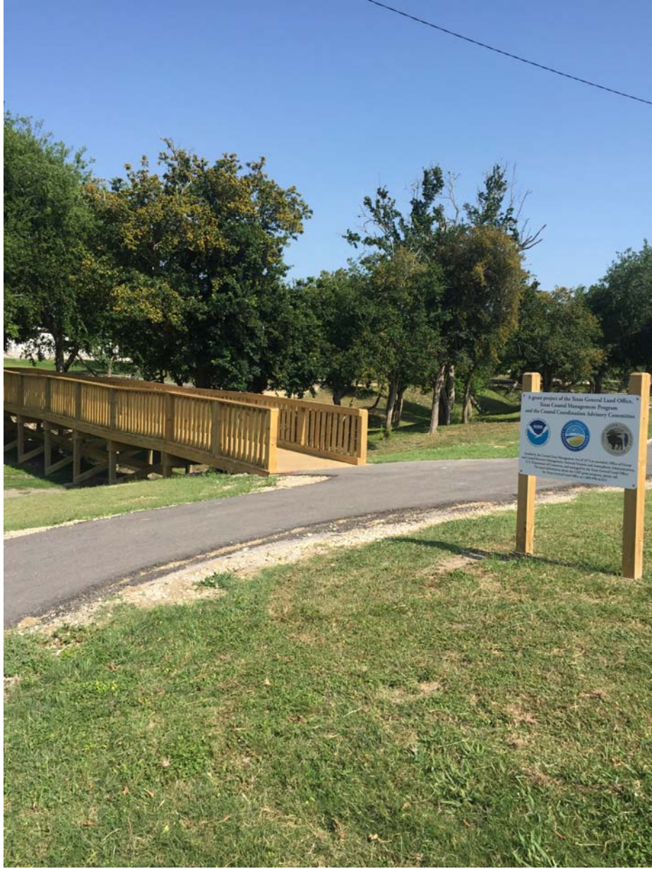
Figure 23. Installed CMP signage
