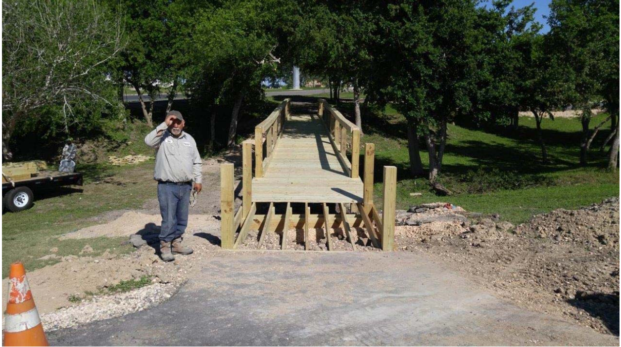
Figure 11. Nature bridge during construction
