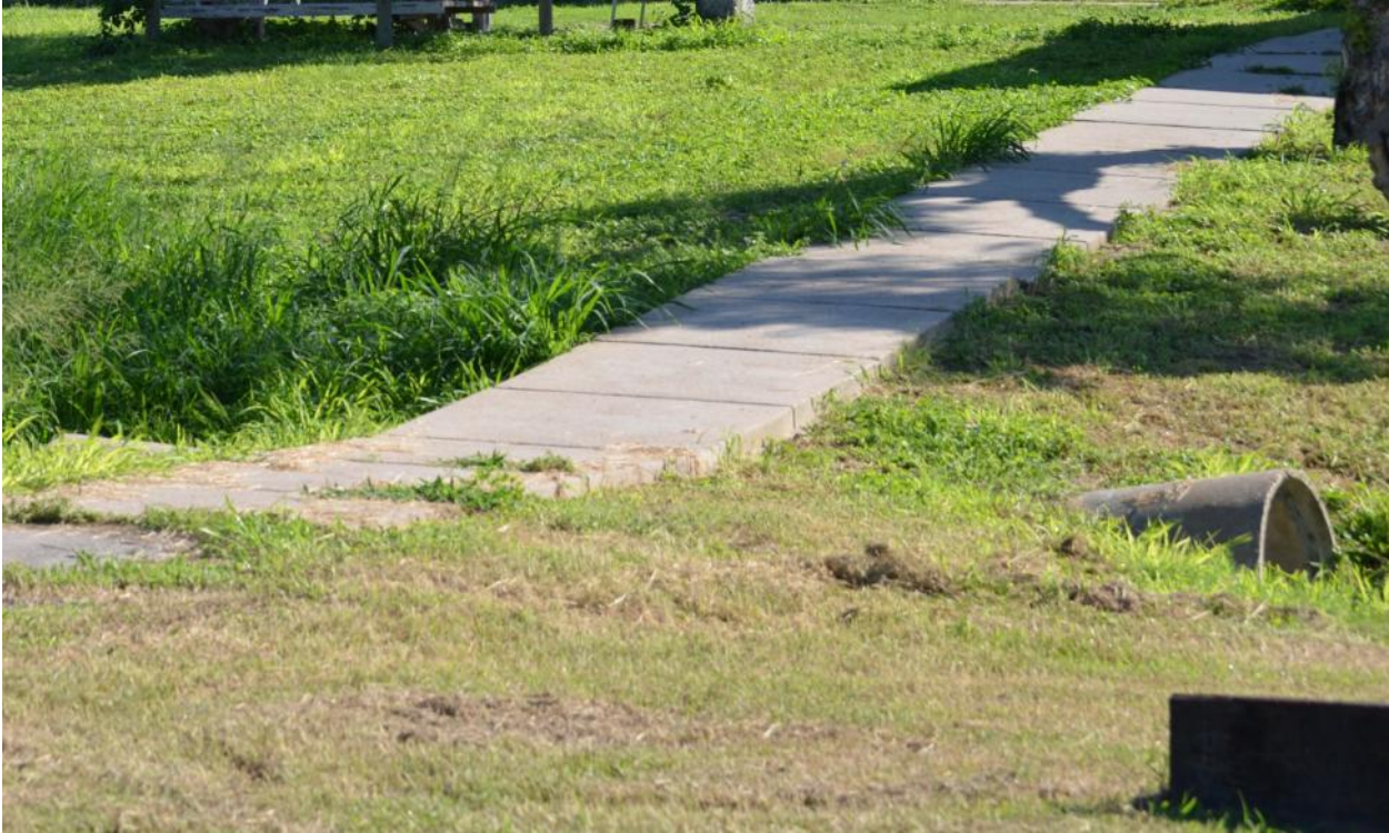
Figure 4. Sidewalk crossing (removed and replaced by wooden foot bridge)
