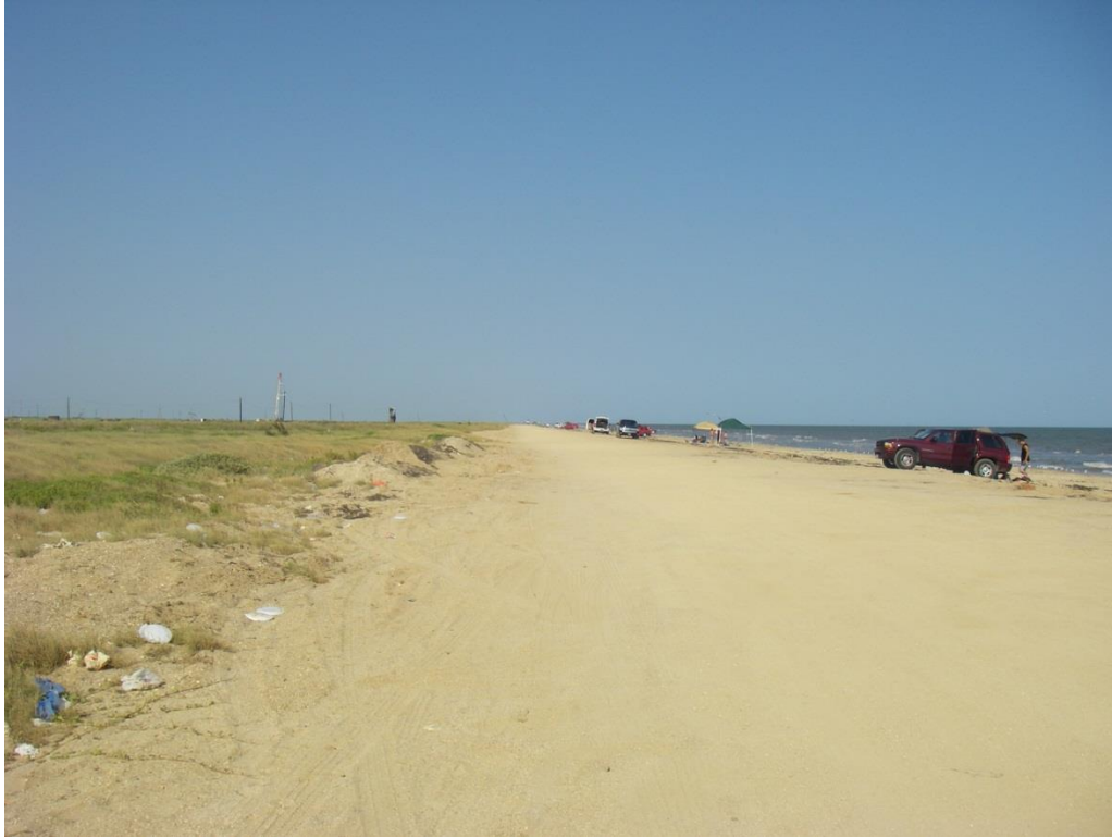
Figure 5.8 End of Highway 87 at High Island, looking north (2011).
