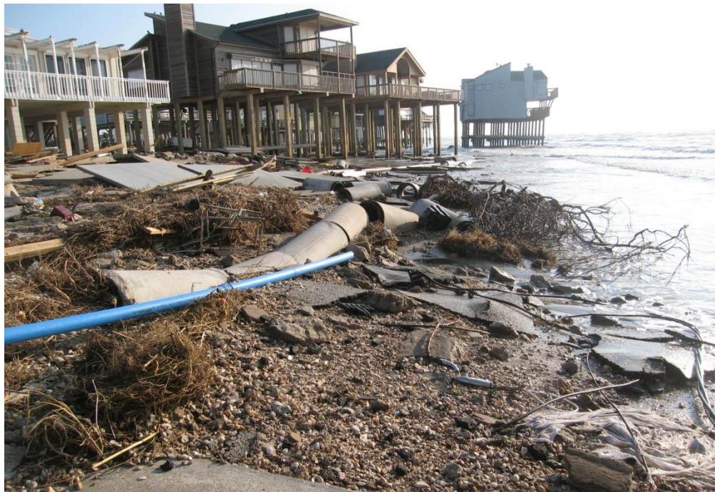
Figure 3.11 Damage in Spanish Grant on West Galveston Island.
