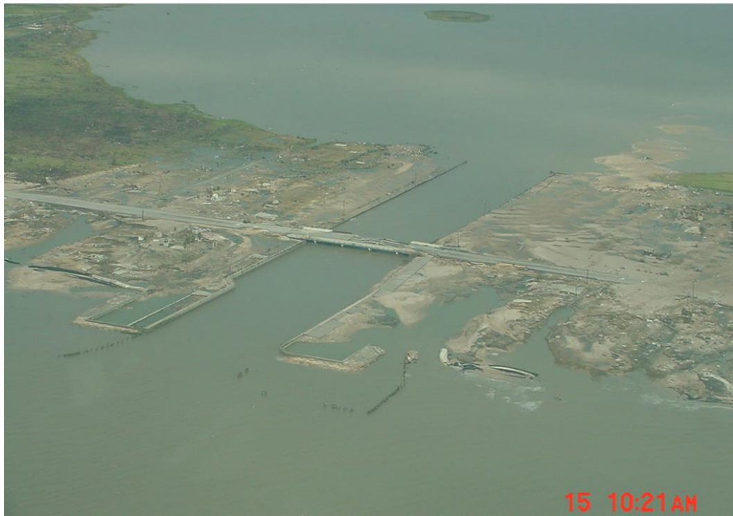
Figure 3.5 Aerial Photograph of damage at Rollover Pass.
