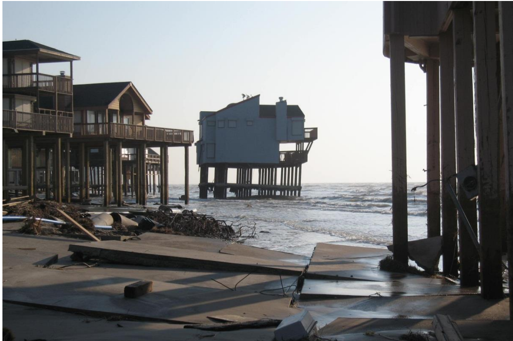
Figure 3.12 Damage in Spanish Grant on West Galveston Island.
