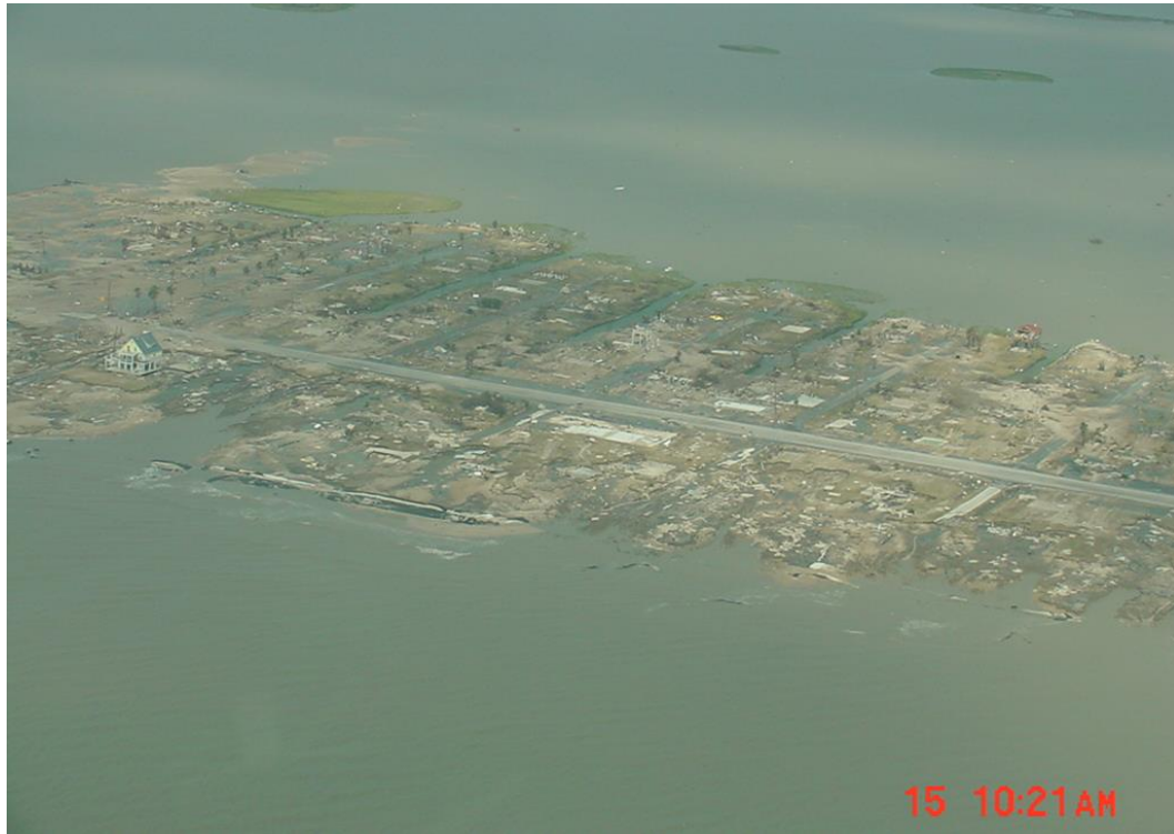
Figure 3.4 Aerial photo of Bolivar Peninsula showing damage to geotextile tubes.
