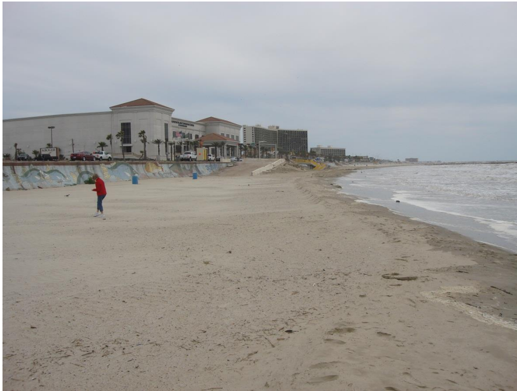
Figure 5.16 Area fronting Galveston Seawall and Convention after beach nourishment.
