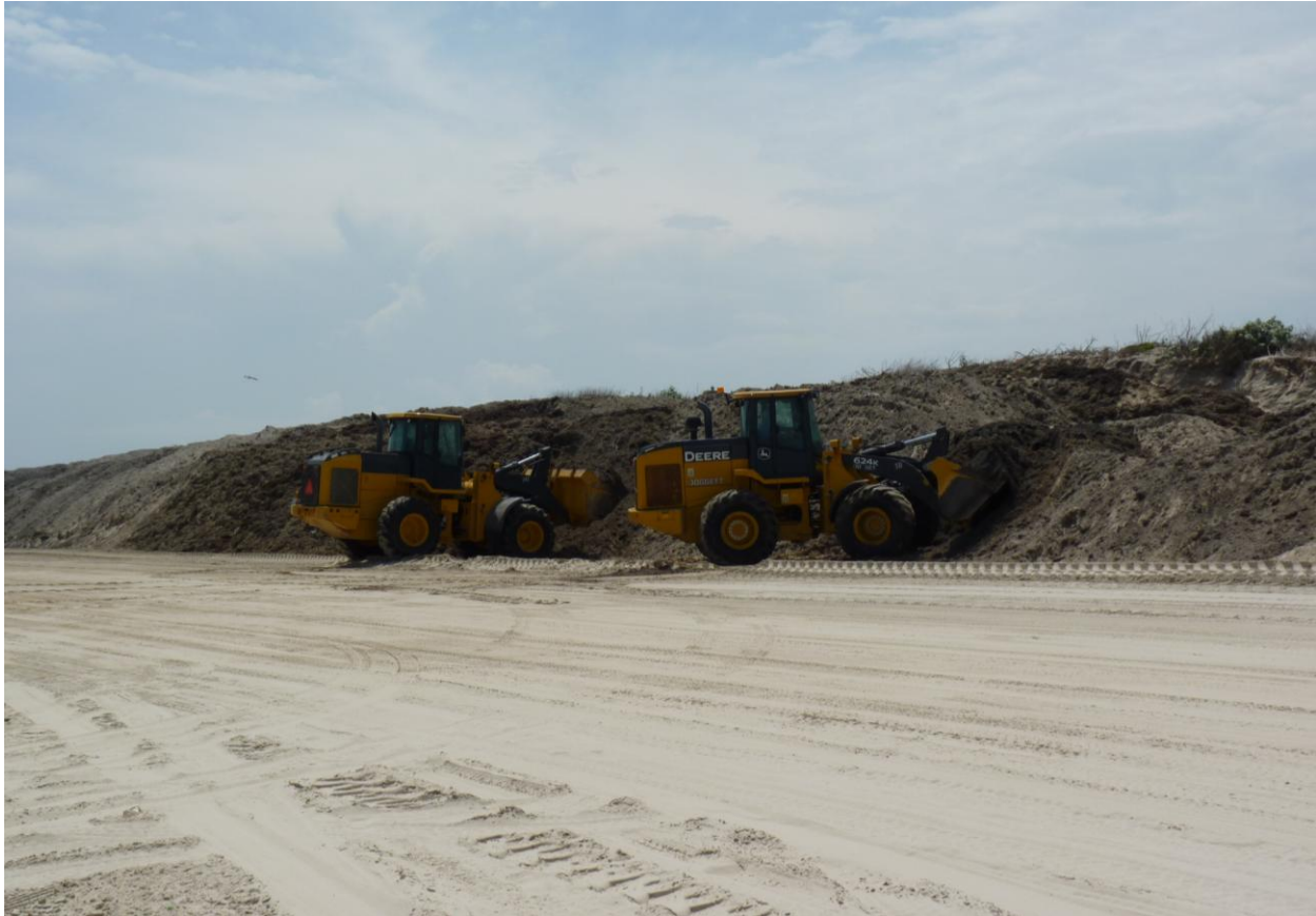
Figure 16. Beach maintenance crews “front-notching” dunes that were created from scraped Sargassam and sand and placed along the beach roadway. After the Sargassam disintegrates, the sand is placed back onto the beach. (July 2014, view to the west)
