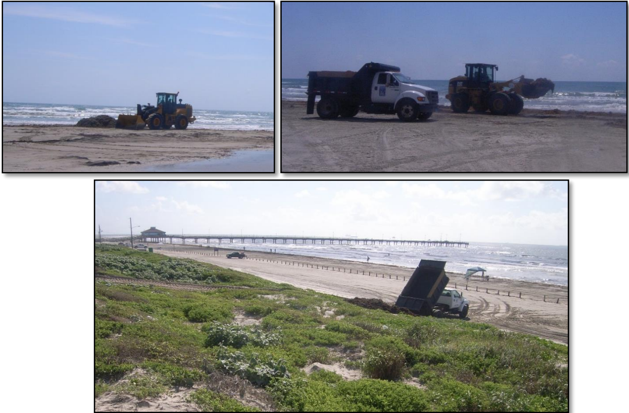
FIGURE 3. REMOVAL OF SARGASSUM FROM THE BEACH (TOP) AND DEPOSITION AT DUNE TOE (BOTTOM) IN CITY OF PORT ARANSAS. SARGASSUM REMOVAL TECHNIQUES AND EQUIPMENT VARY AMONG JURISDICTIONS.
