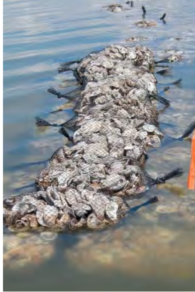
Photo 1: Recycled oysters are placed in mesh bags and stacked to create new habitat and protect the shore from erosion photo courtesy of Galveston Bay Foundation
