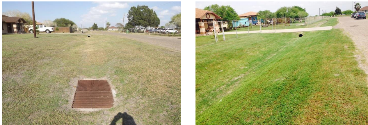
Figure 2. View of the bioretention cell areas before construction.
