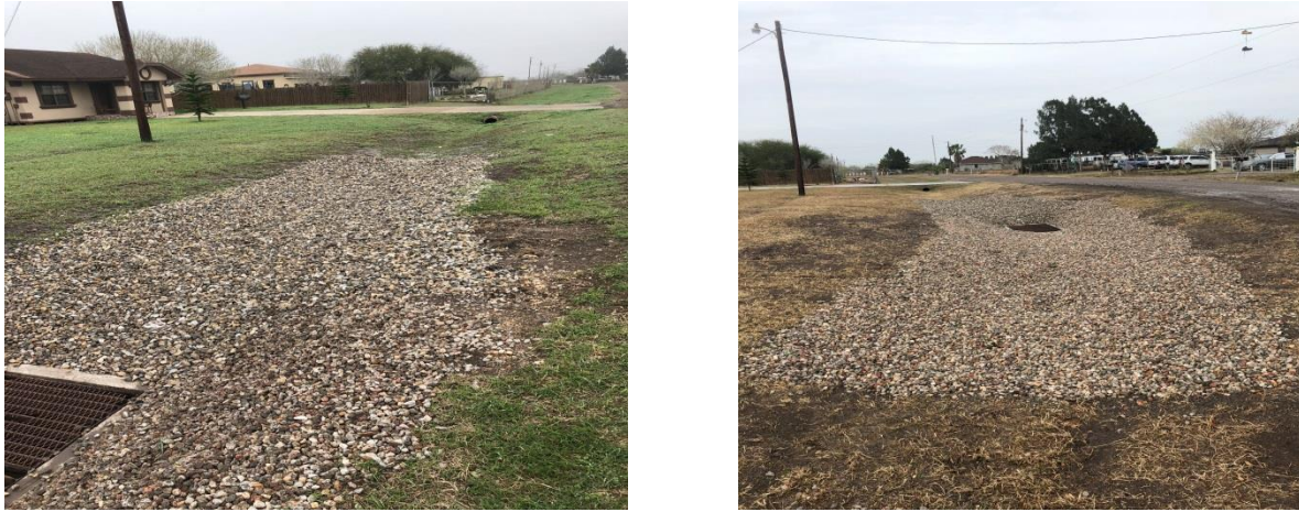
Figure 3. View of the La Esquina Colonia bioretention cells after construction.
