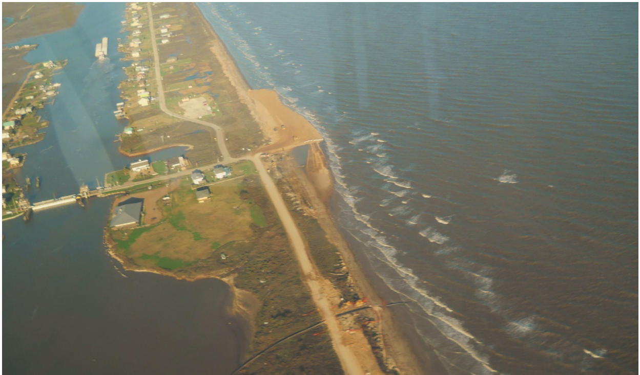
Figure 3.8 Sargent Beach during Construction (2/8/13; Photo provided by Texas GLO)
