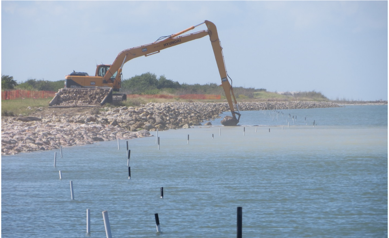
Figure 4.3 Revetment Reconstruction (October 28, 2013)
