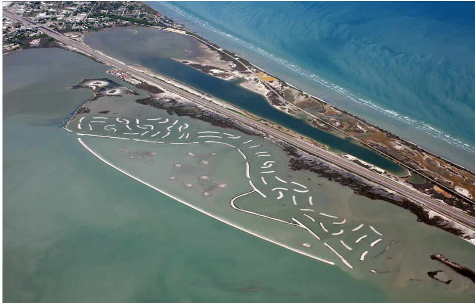
Figure 4.7 Nueces Bay Portland Causeway Marsh Restoration Phase II Post-Construction (Photo provided by the GLO; photo dated March 30, 2014)
