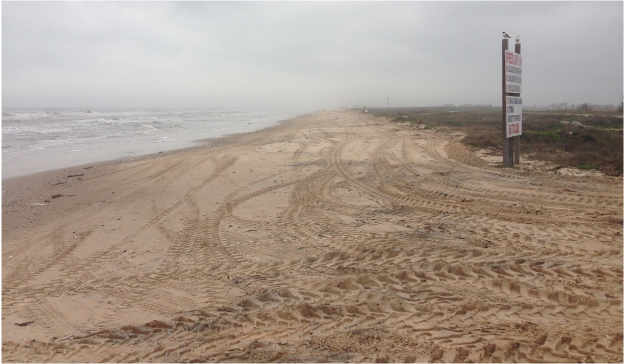
Figure 3.10 Westward View of Sargent Beach from FM 457 Two Years Post-Construction (3/4/15)
