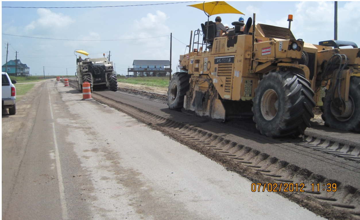
Figure 3.5 CR 257 Road Repairs during Construction (July 2, 2012; photo provided by GLO)
