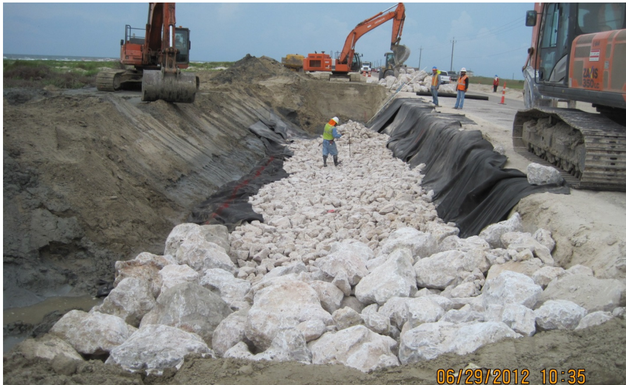
Figure 3.4 CR 257 Rock Revetment during Construction (June 29, 2012; photo provided by GLO)
