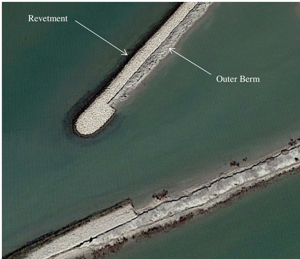
Figure 4.8 Detail of Rock Revetment at Southwest End of Outer Berm (Aerial Source: Google Earth)
