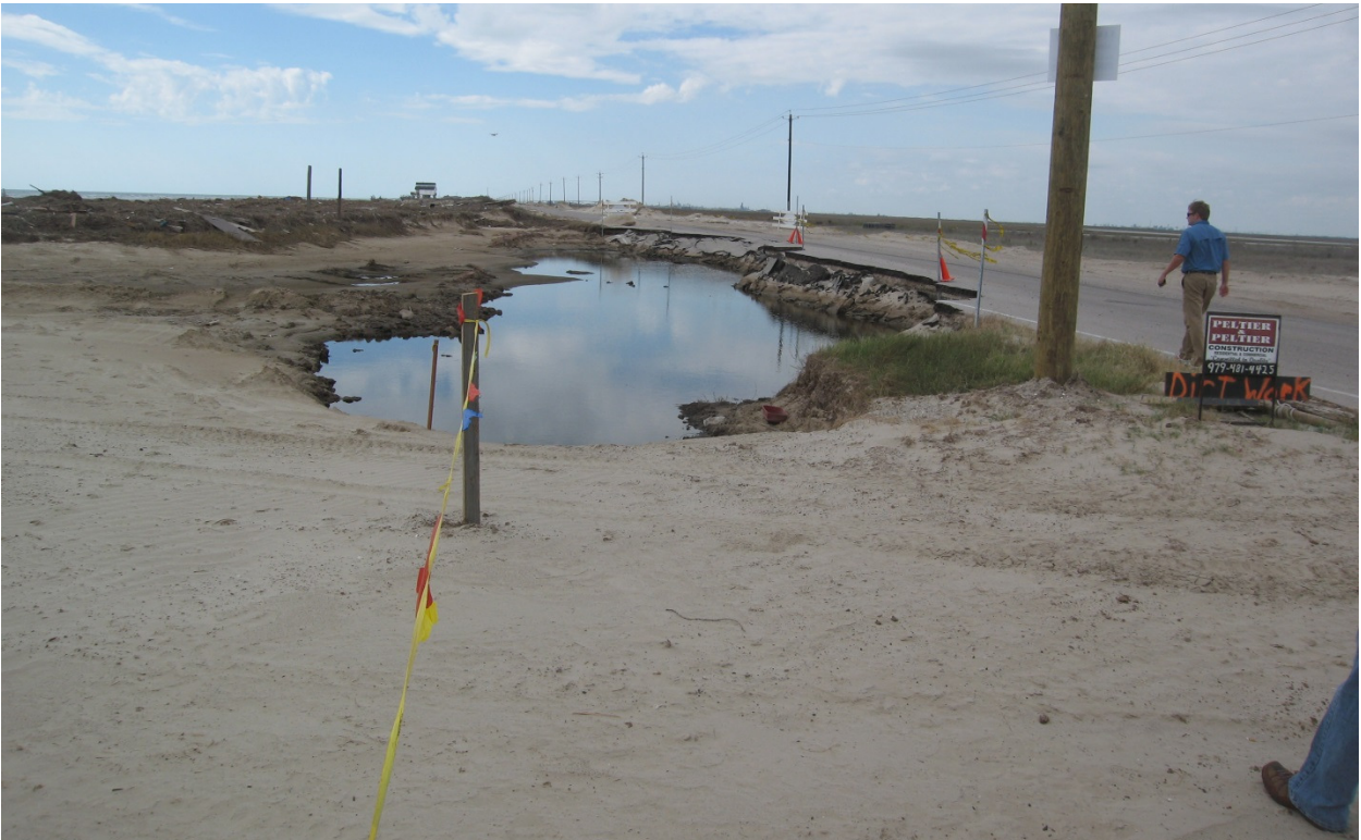
Figure 3.3 CR 257 Post-Hurricane Ike (November 4, 2008; photo provided by GLO)
