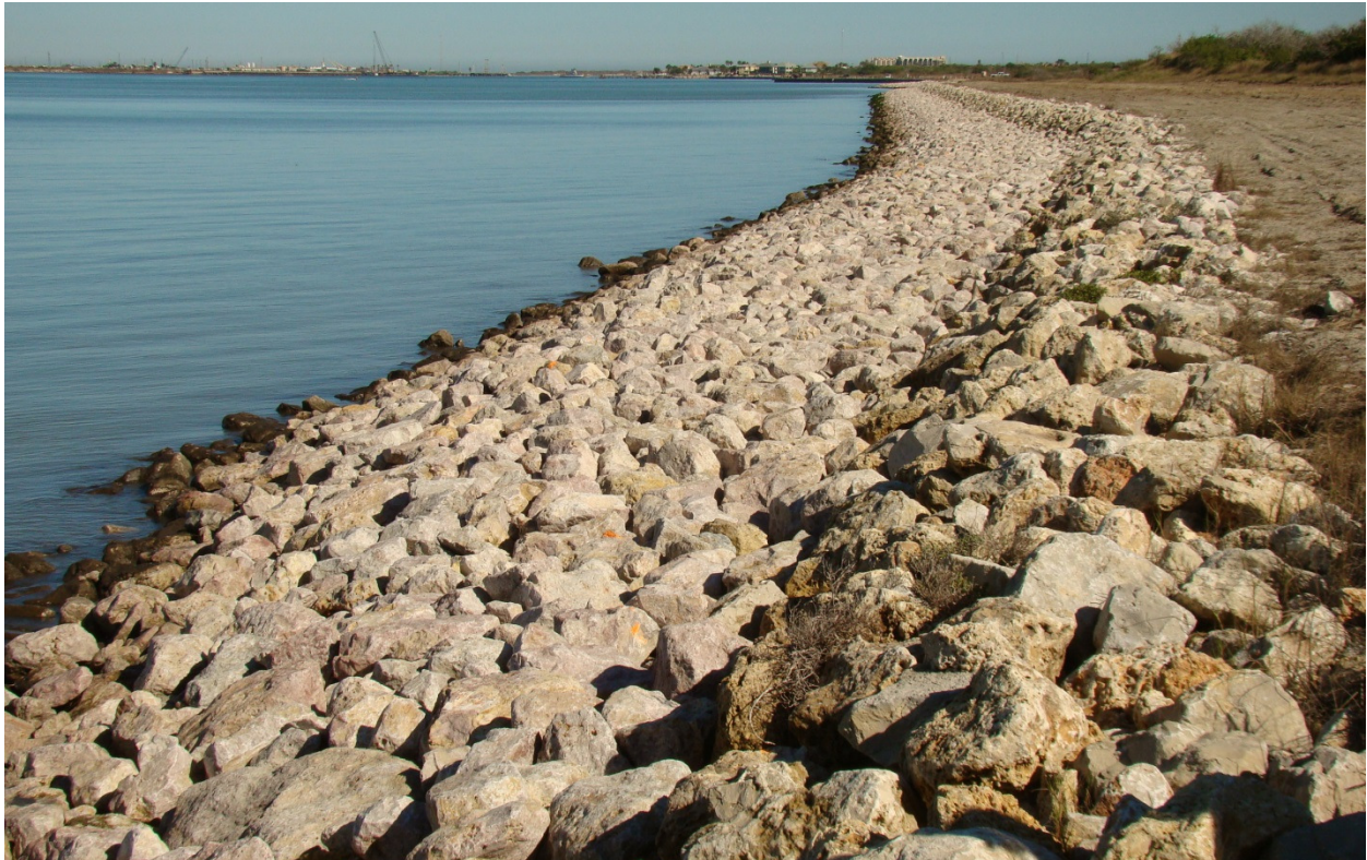
Figure 4.4 Post-construction Conditions (12/16/13; photo provided by GLO)
