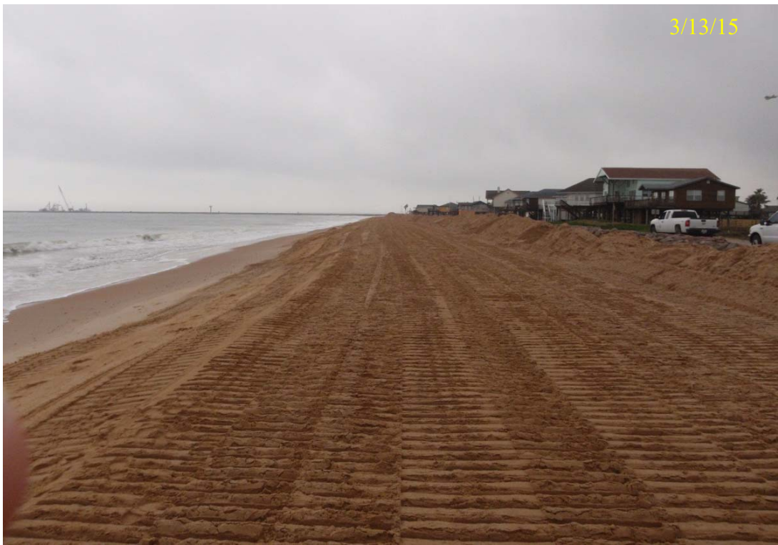
Figure 3.3.3 Westward View of Project #1570 Pre- and Post-construction (provided by GLO)
