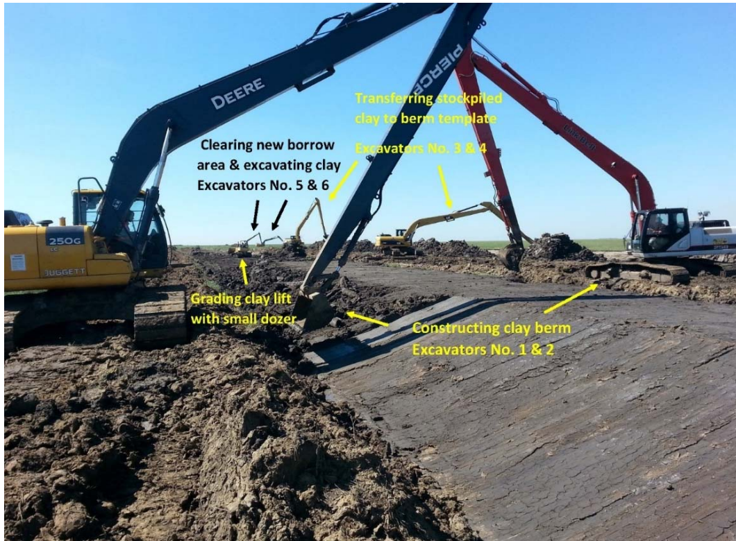
Figure 4.1.2 McFaddin NWR overwash protection berm under construction (Photo from GLO)
