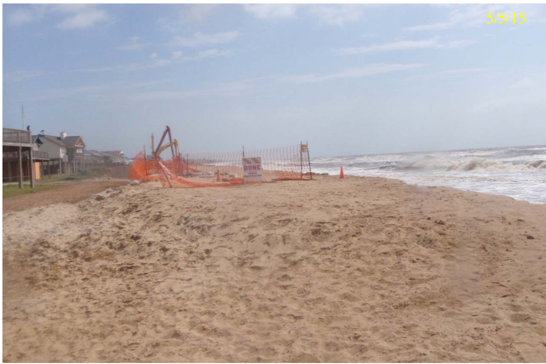
Figure 3.3.5 Westward Terminus of Revetment During Construction (provided by GLO)
