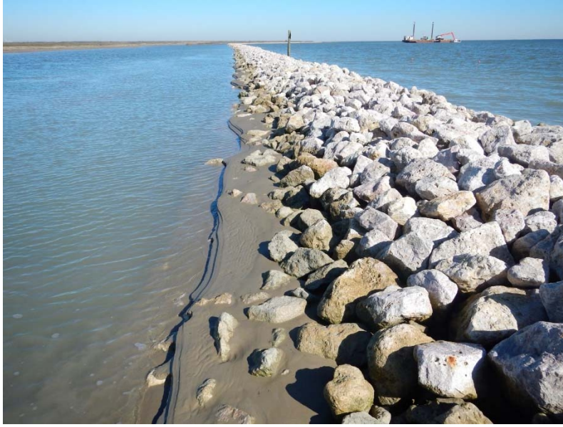
Figure 4.6.2 Oyster Lake Habitat Restoration Rock Breakwater
