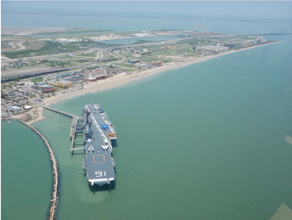
Figure 3.2.7 Post-construction Aerial (Photo provided by GLO)
