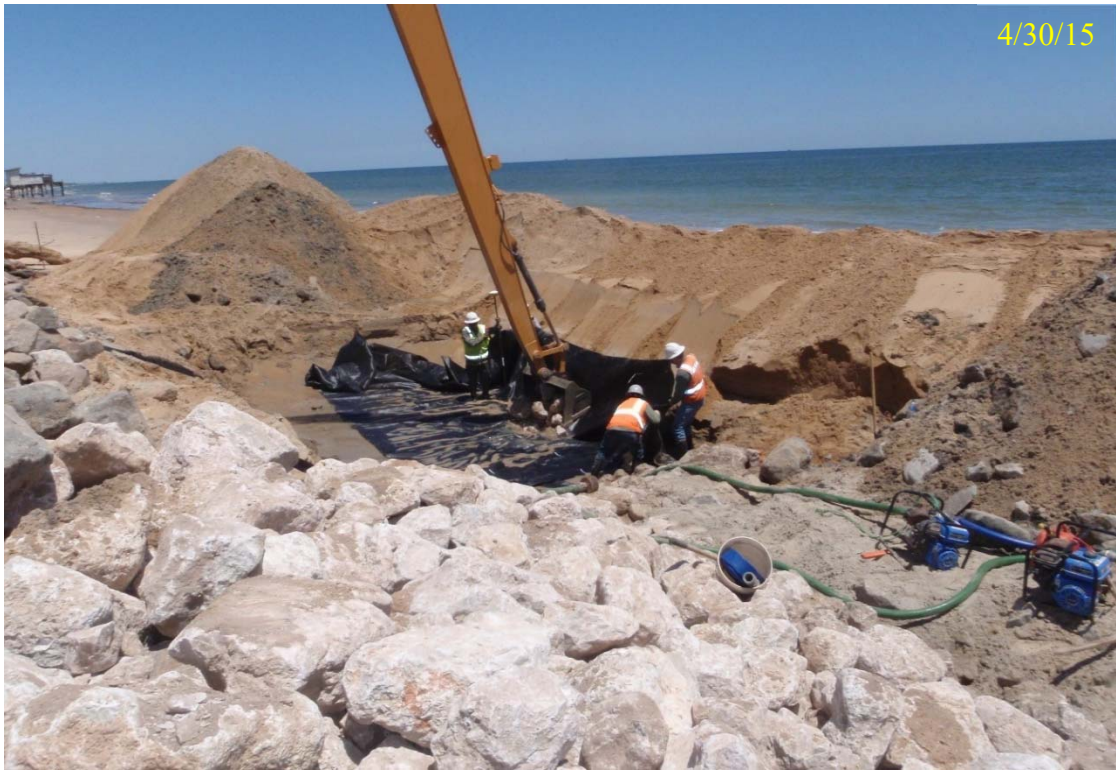
Figure 3.3.4 Surfside Revetment Project#1573 During Construction (provided by GLO)
