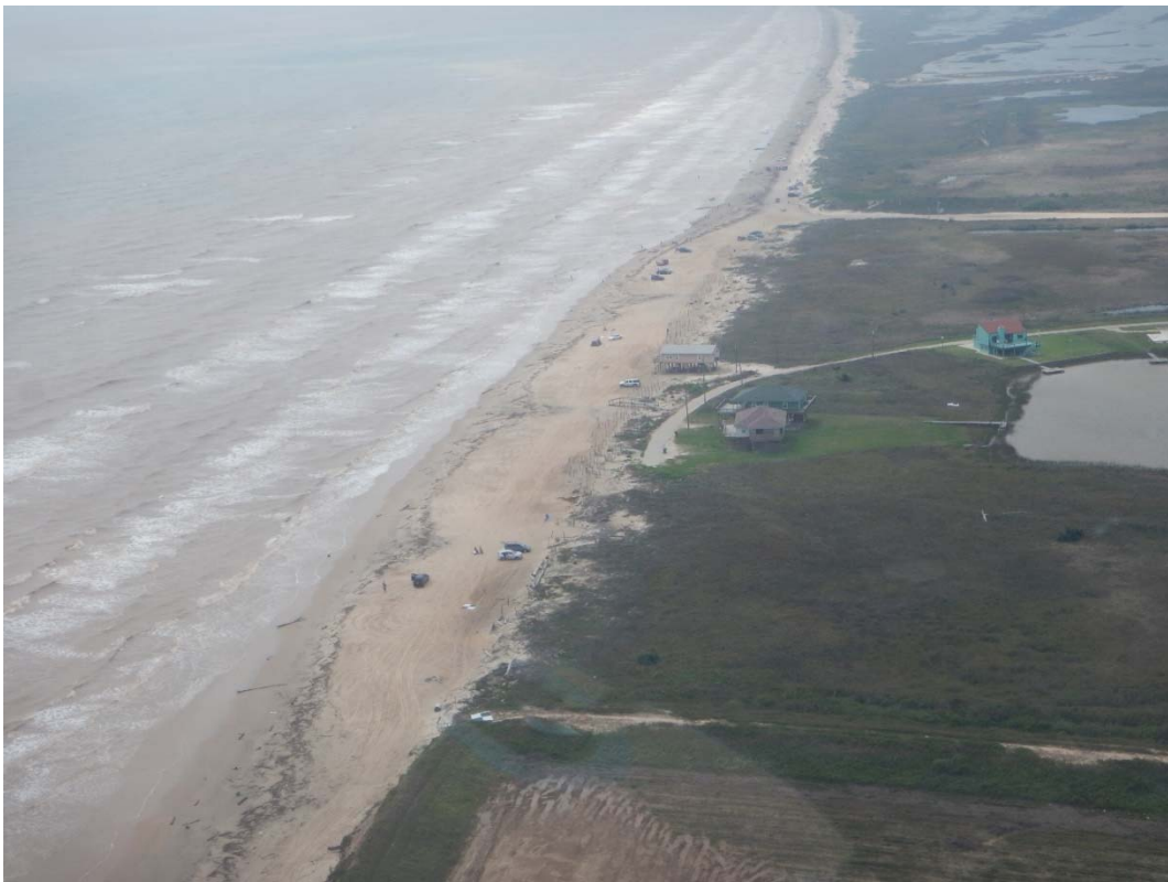
Figure 3.4.5 Bryan Beach Post-Construction (3/14/16; Photo provided by GLO)
