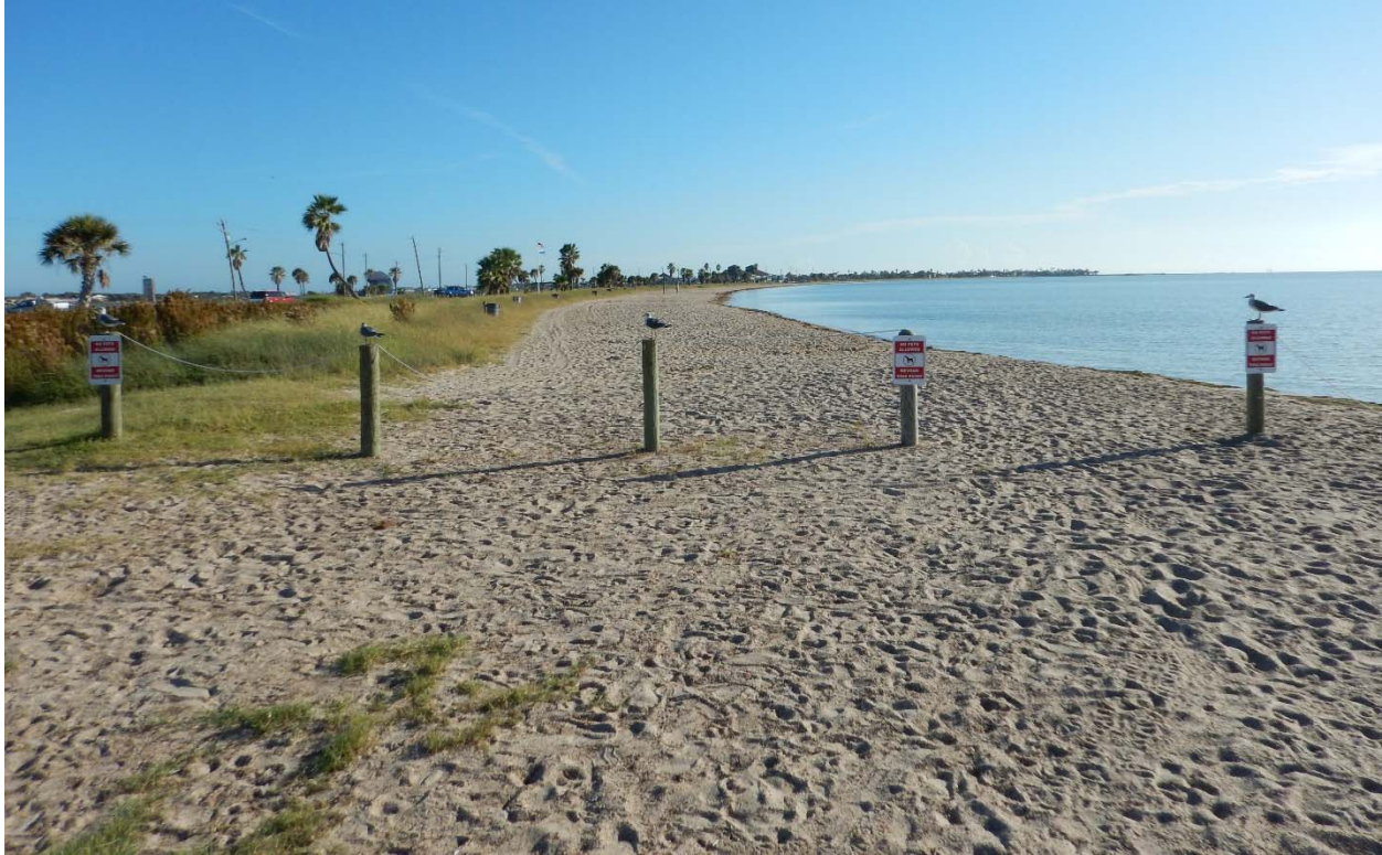
Figure 3.5.6 West End of Rockport Beach Project #1603 Post-construction (10/20/16)
