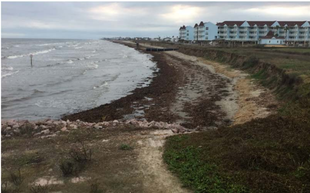
Figure 3.1.5 End of seawall project area 22 months after construction (1/19/17)
