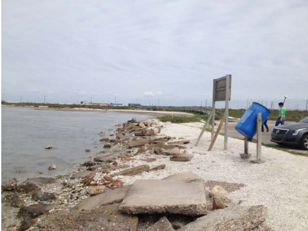
Figure 4.3.2 Pre-Construction Shoreline of Indian Point (Photo provide by GLO)
