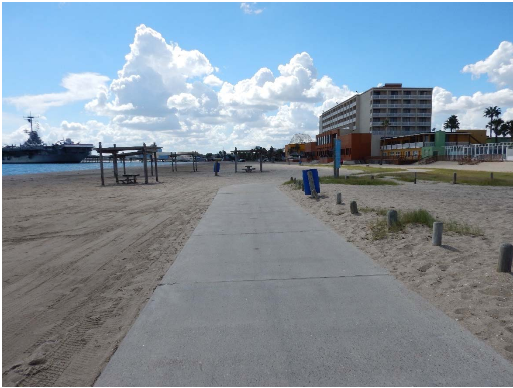
Figure 3.2.9 Southwestward View from Station 13+50, Post-Construction (10/20/2016)
