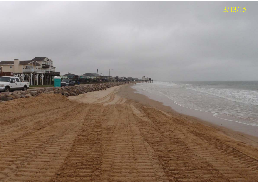
Figure 3.3.2 Eastward View of Project #1570 Pre-and Post-construction (provided by GLO)
