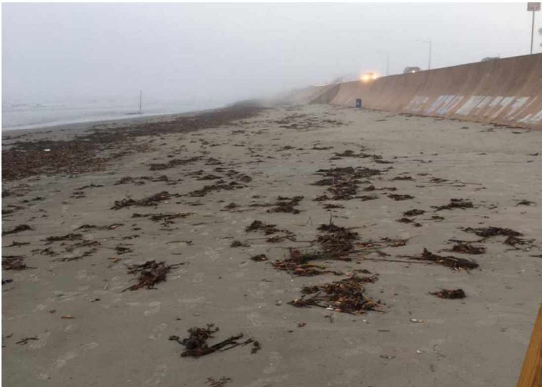
Figure 3.7.6 Galveston Seawall Beach Nourishment 14 months after completion (77 th St)
