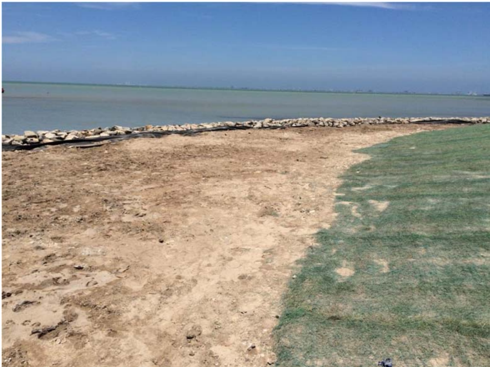
Figure 4.4.3 CEPRA Project #1576 during Construction (provided by GLO)
