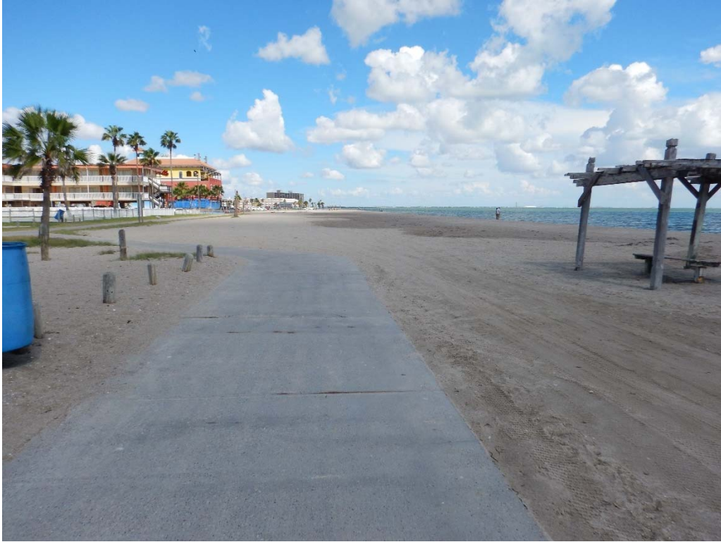
Figure 3.2.8 Northeastward View from Station 13+50, Post-Construction (10/20/2016)
