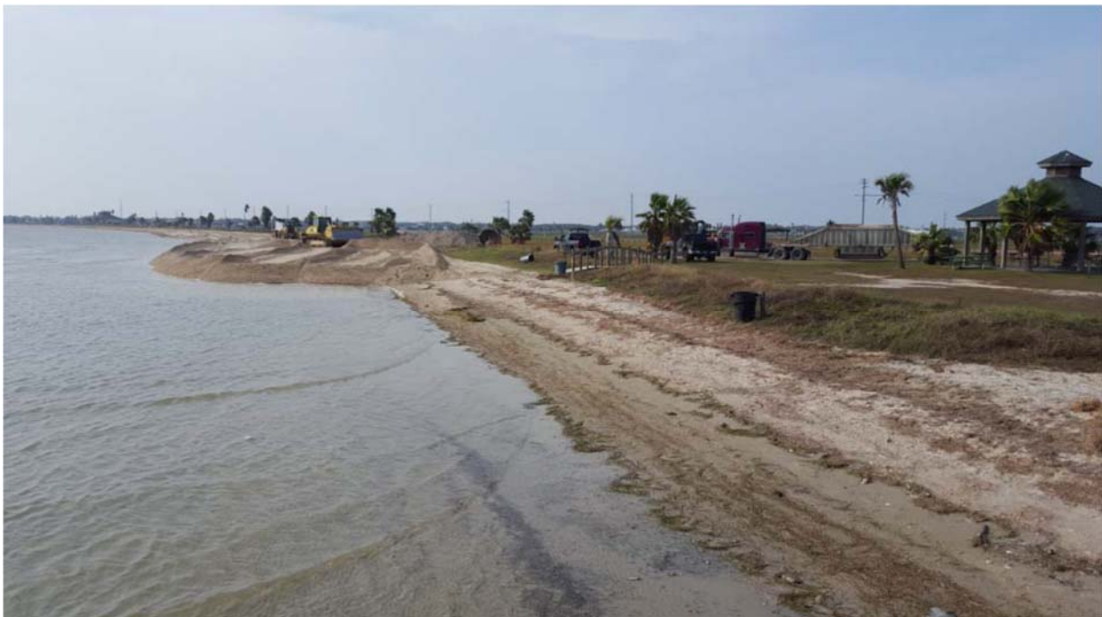
Figure 3.5.3 Rockport Beach #1603 During Construction Near East End (12/11/15; provided by GLO)
