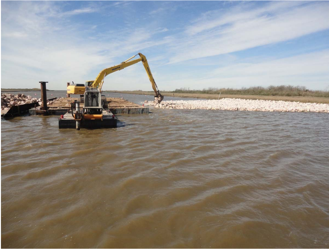
Figure 4.5.2 Keith Lake Fish Pass Baffle Under Construction (Photo provide by GLO)
