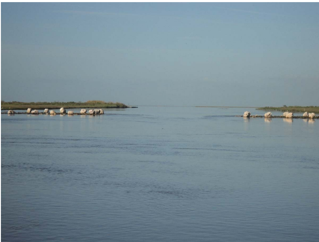
Figure 4.5.3 Completed Keith Lake Fish Pass Baffle (Photo provided by GLO)
