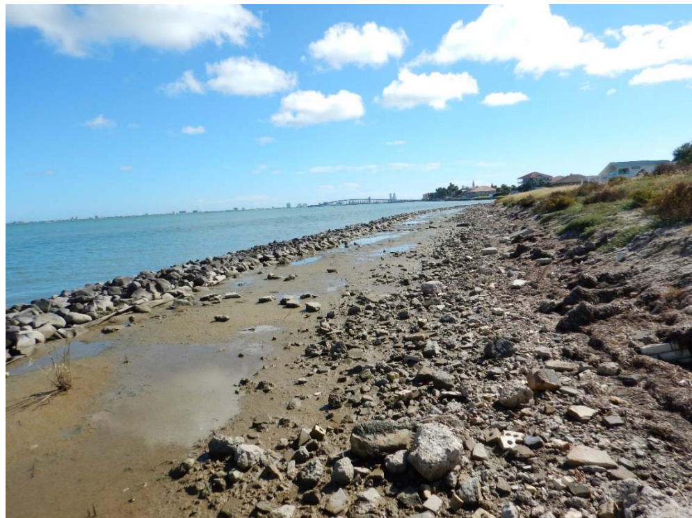
Figure 4.4.5 October 2016 Site Conditions
