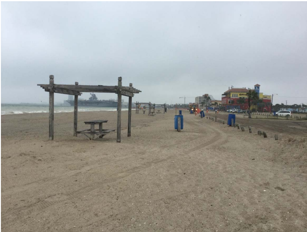
Figure 3.2.5 Southwestward View of North Beach During Construction (Photo provided by GLO)
