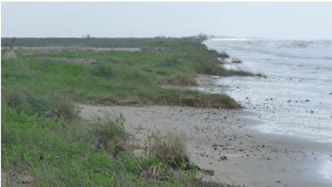
Figure 4.2.3 Project #1530 Pre-Construction Conditions, April 2017 (Source: GLO)
