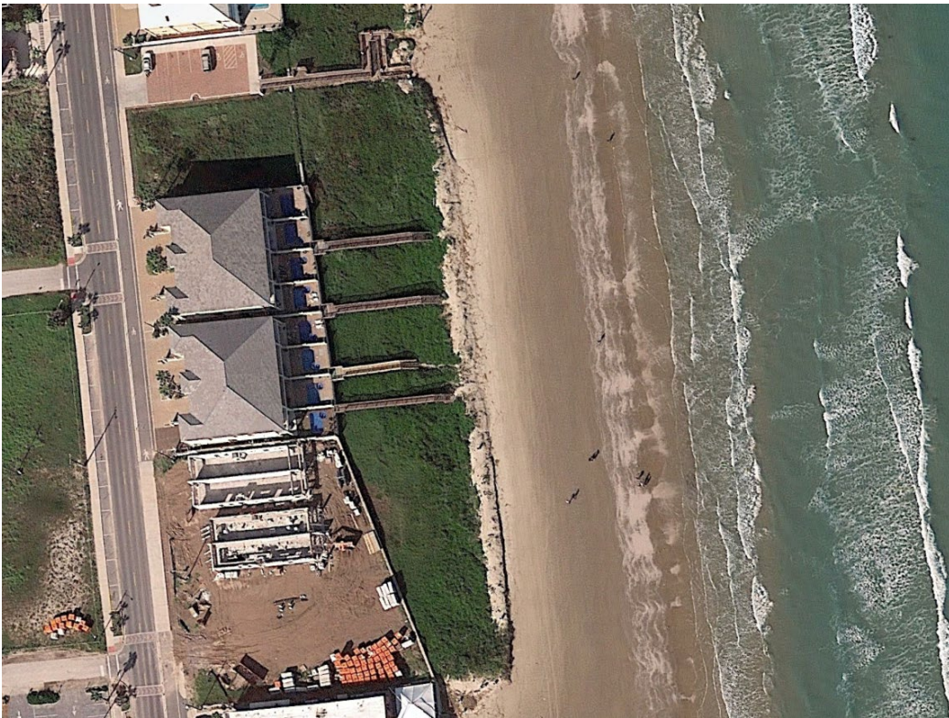
Figure 3.2.11 Project #1574 South End Post-Harvey, December 2017 (Source: Google Earth)
