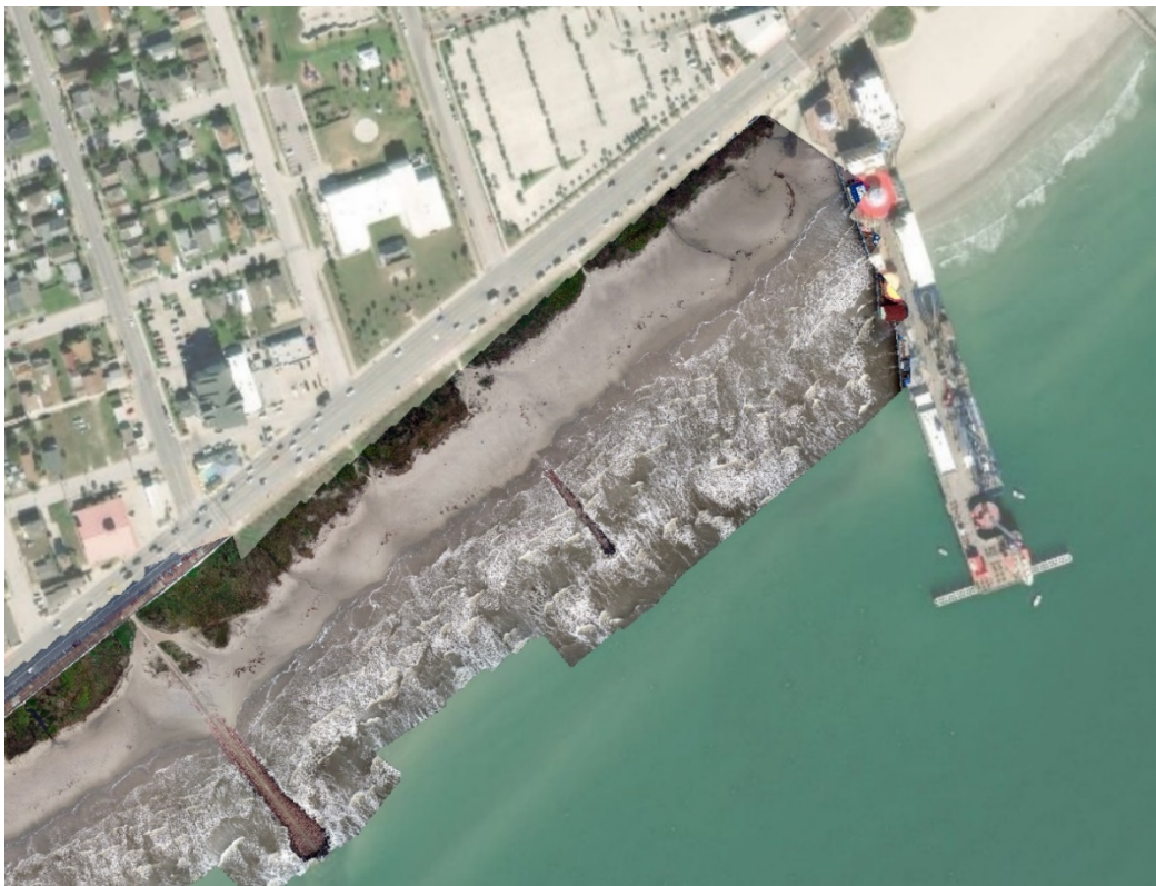
Figure 3.1.6 Project #1566 Conditions Two Years Post-construction (2/16/19)
