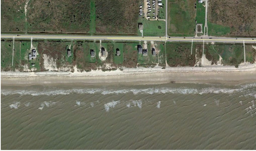
Figure 3.5.5 Project #1619 Aerial Imagery, February 2017 (Source: Google Earth)
