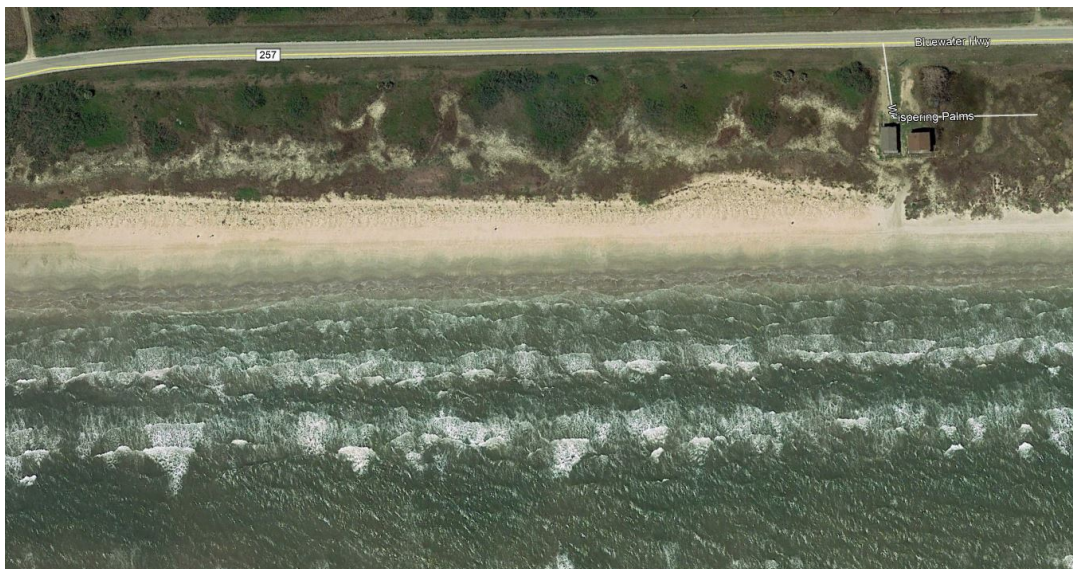
Figure 4.1.5 Project #1529 Post-Hurricane Harvey, March 2018 (Source: Google Earth)
