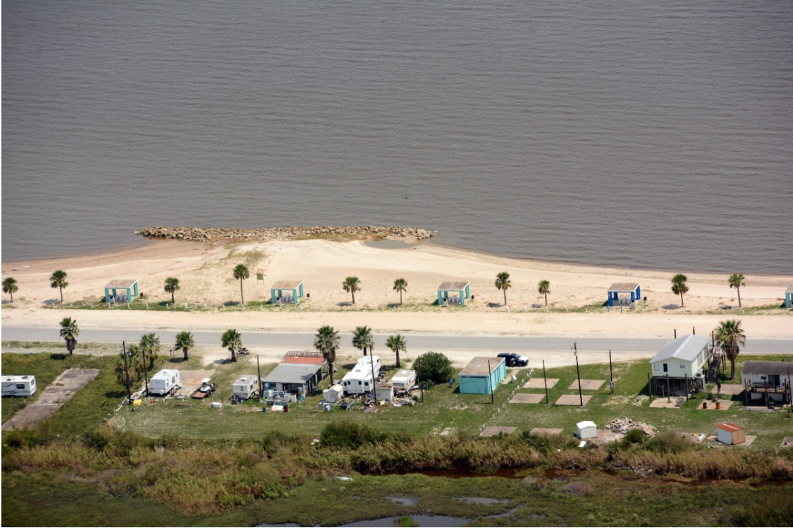
Figure 3.3.5 Project #1604 Conditions Post-Hurricane Harvey
