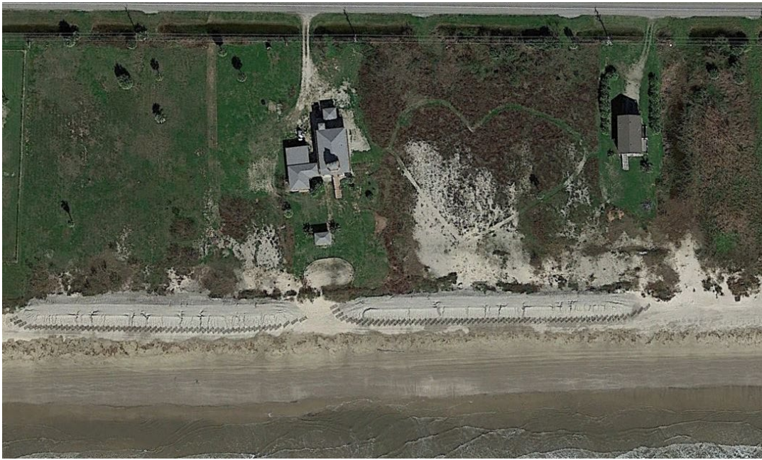
Figure 3.4.10 Project #1610 Post-Construction, February 2017 (Source: Google Earth)
