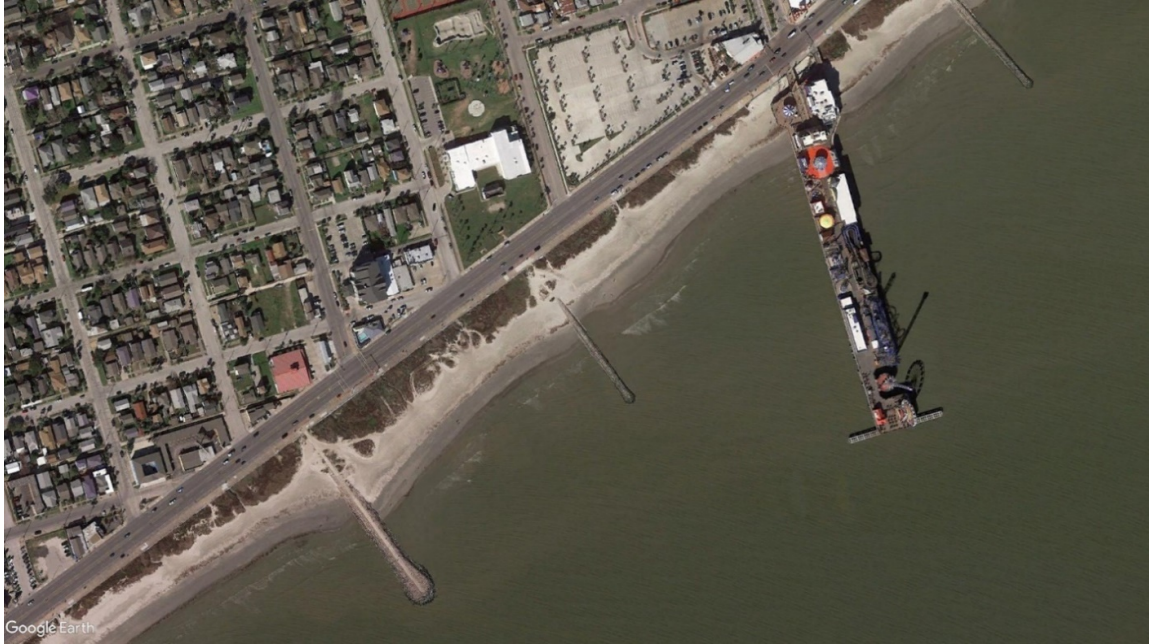
Figure 3.1.3 Project #1566 Pre-construction Conditions (Source: Google Earth, January 22,2017)
