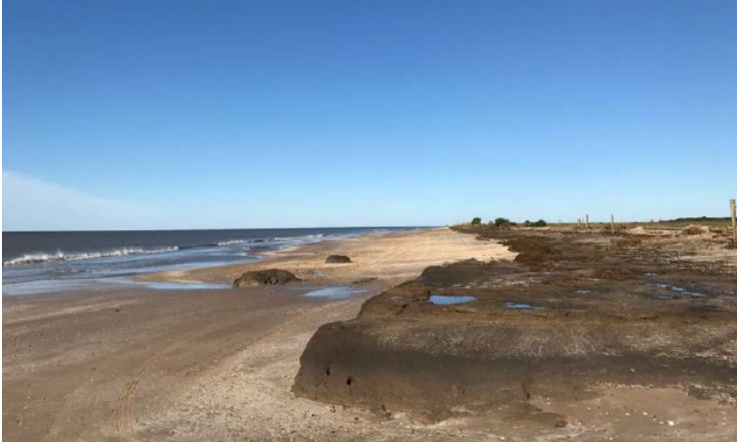
Figure 4.2.2 Project #1530 Pre-Construction Conditions, April 2017 (Source: GLO)
