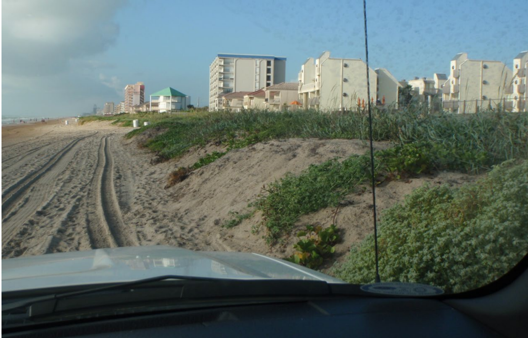
Figure 3.2.2 Project #1574 Pre-Construction, June 2015 (Source: Texas GLO)
