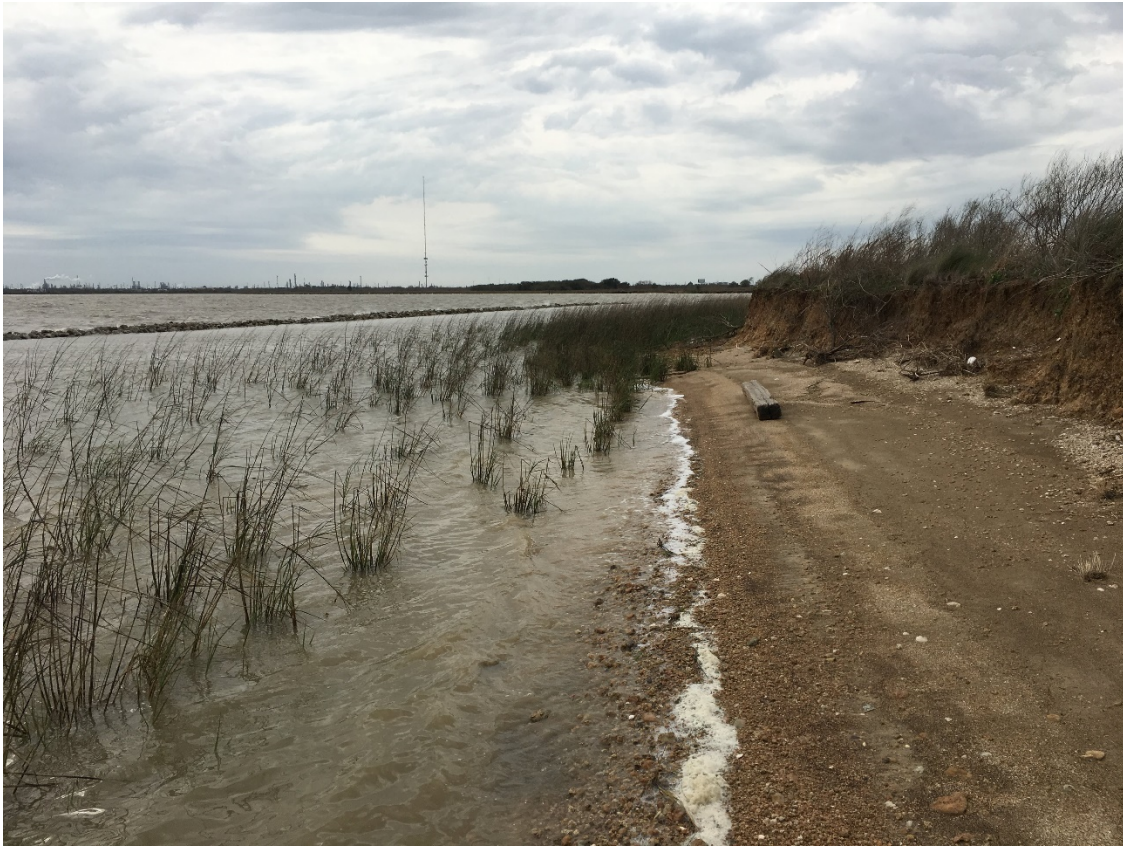
Figure 4.8.2 Project #1627 One Year Post-construction
