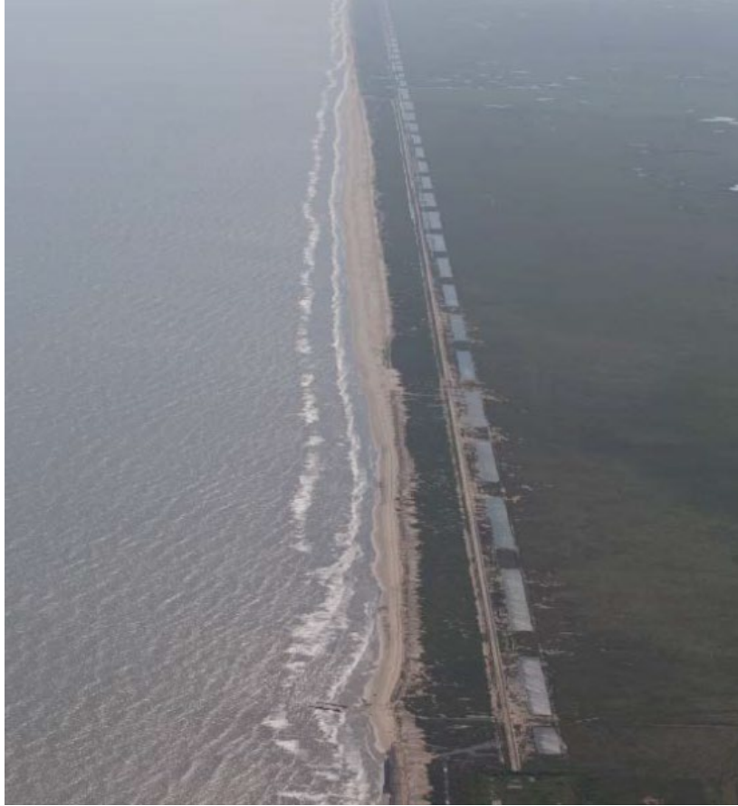
Figure 4.2.4 Project #1530 Post-Construction Aerial View (Source: GLO)
