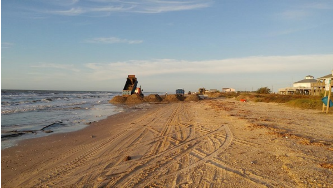
Figure 3.4.5 Project #1610 During Construction, November 2017 (Source: GLO)
