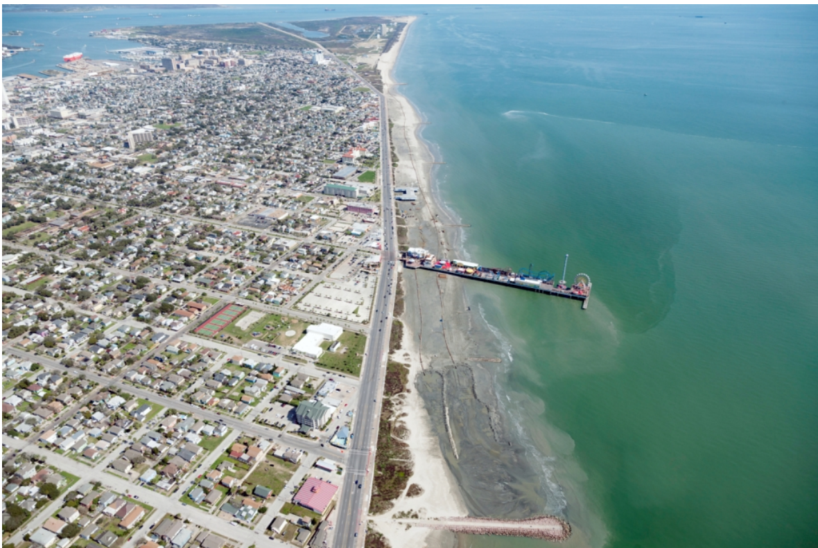
Figure 3.1.4 Project #1566 During Construction (Source: HDR, 2017)
