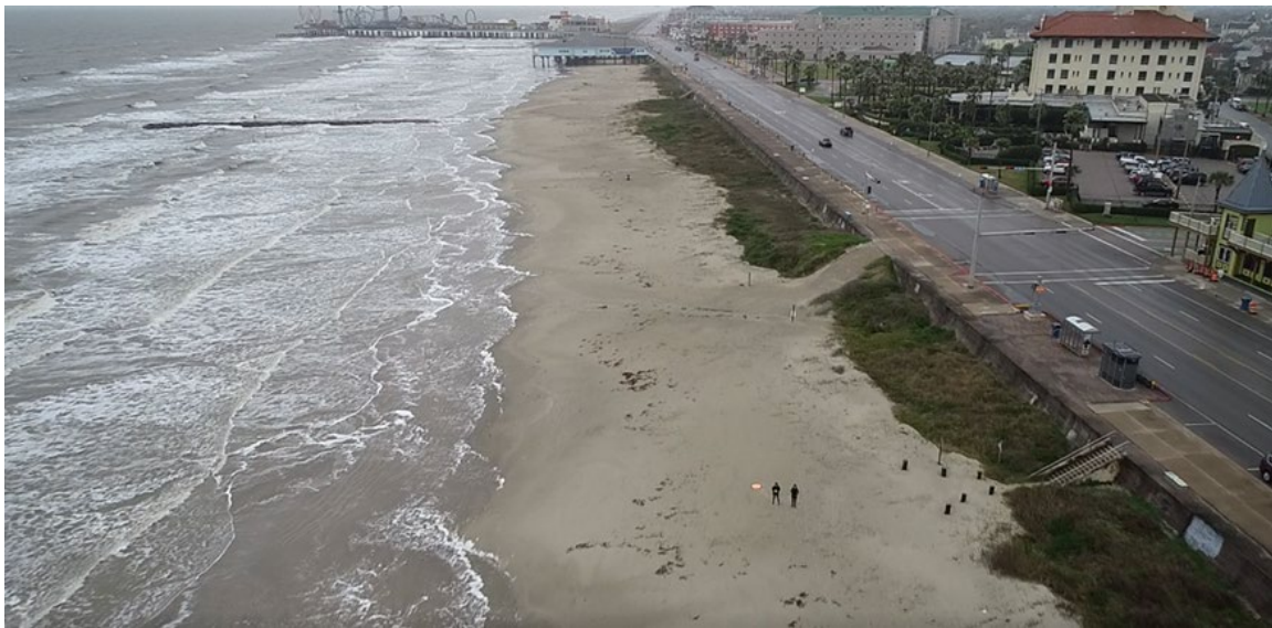
Figure 3.1.2 Project #1566 Two Years Post-construction, 18 th Street Looking Southwest (2/26/19)
