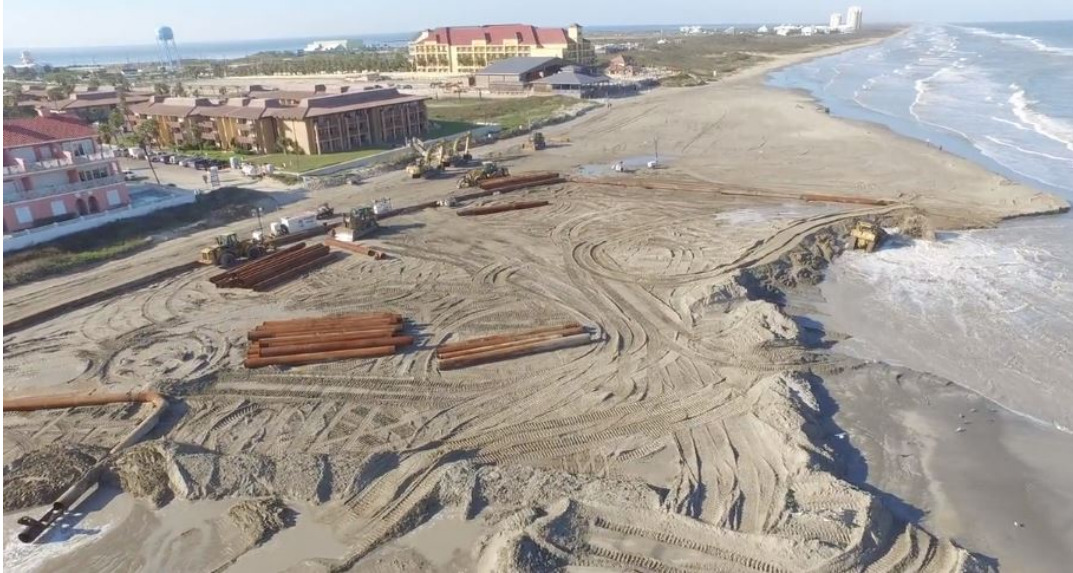
Figure 3.2.4 Project #1574 During Construction, December 2015 (Source: Texas GLO)
