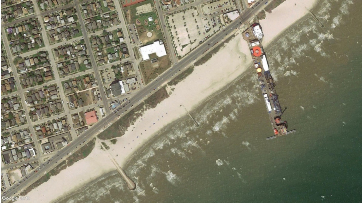
Figure 3.1.5 Project #1566 Post-construction (Source: Google Earth, 3/21/18)
