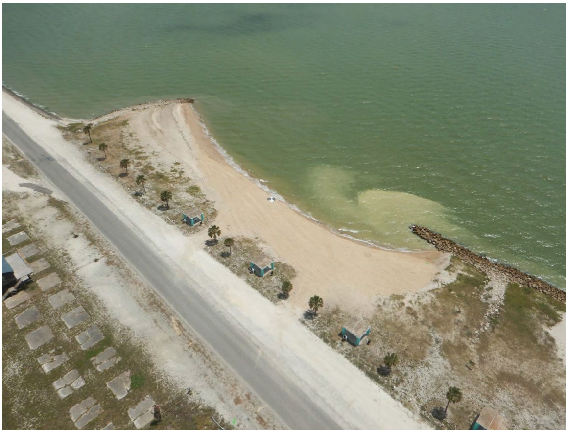
Figure 3.3.4 Project #1604 Post-construction Conditions
