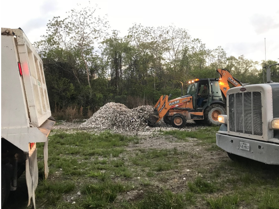
Contractors piling shell after loading shell for transport
