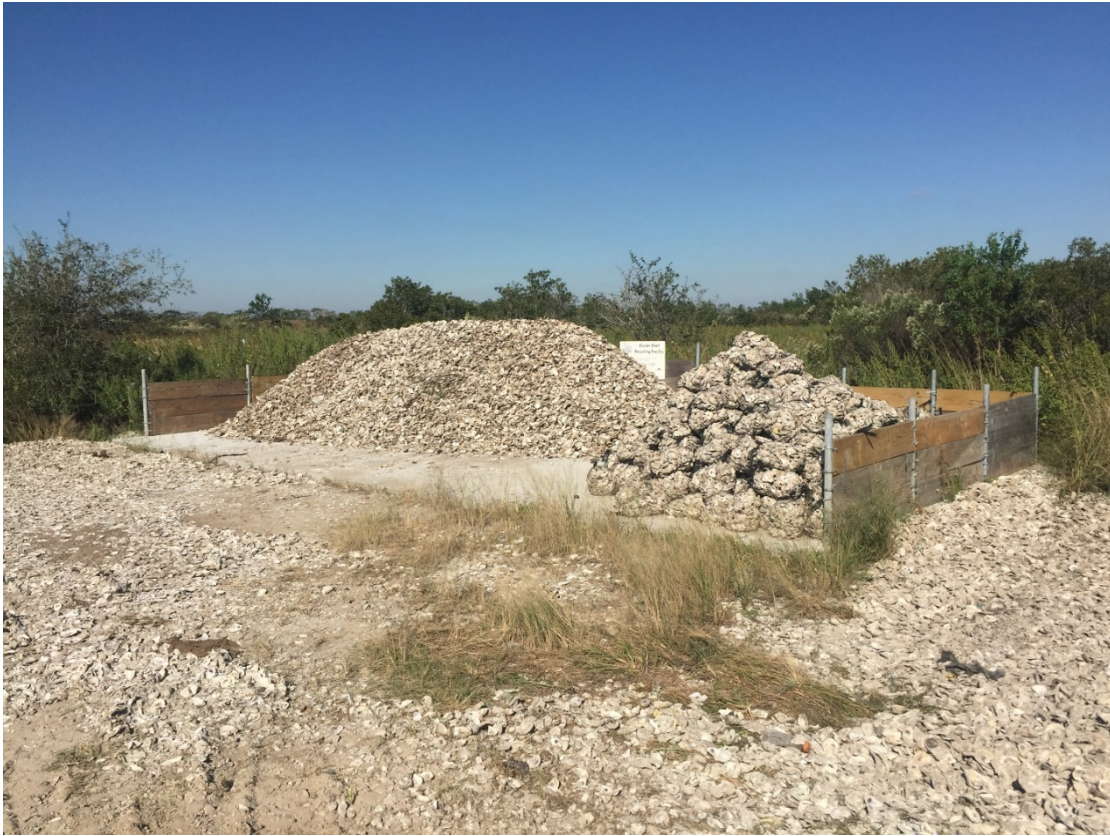
Cured and bagged oyster shell on cement curing pad
