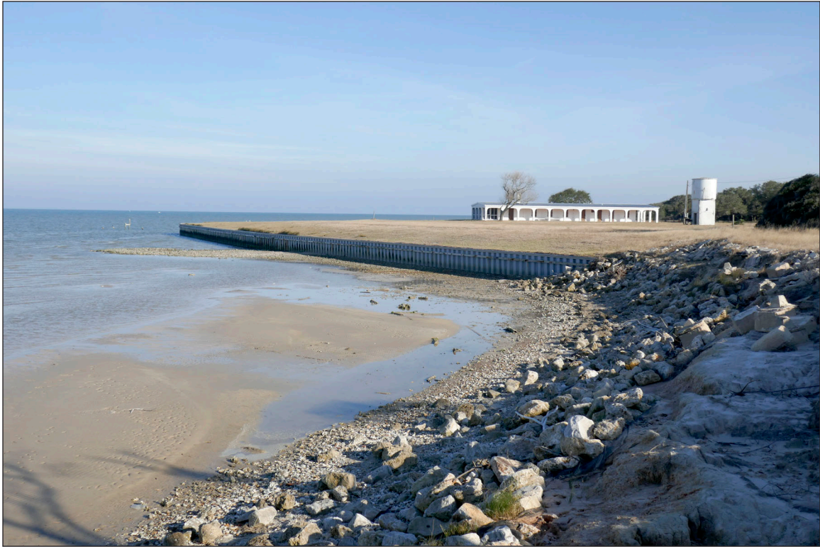
Figure 25. Bulkhead and riprap along the Matagorda Bay shoreline at the ranch house.
