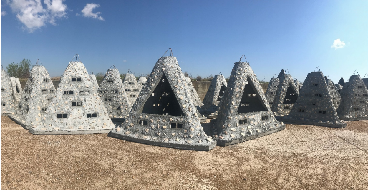
Figure 4. Mid relief pyramids completed and staged for moving to Port Isabel for deployment preparations.
