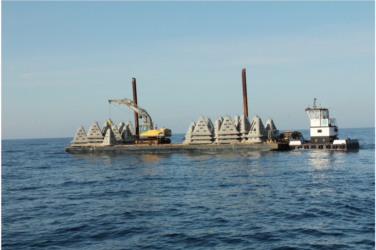
Figure 6. Deployment image of the mid relief pyramids being placed in the Rio Grande Valley Nearshore Reef Site (PS-1005) on 23 August 2018.
