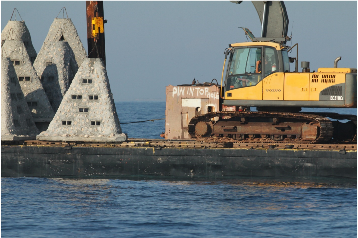
Figure 8. Close-Up Image of the deployment of the mid relief pyramids being placed in the Rio Grande Valley Nearshore Reef Site (PS-1005) on 23 August 2018.
