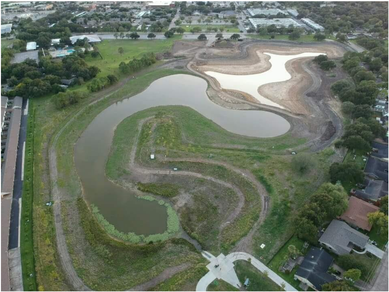
Figure 22. Phase 1 habitat island construction, land bridge still intact.
