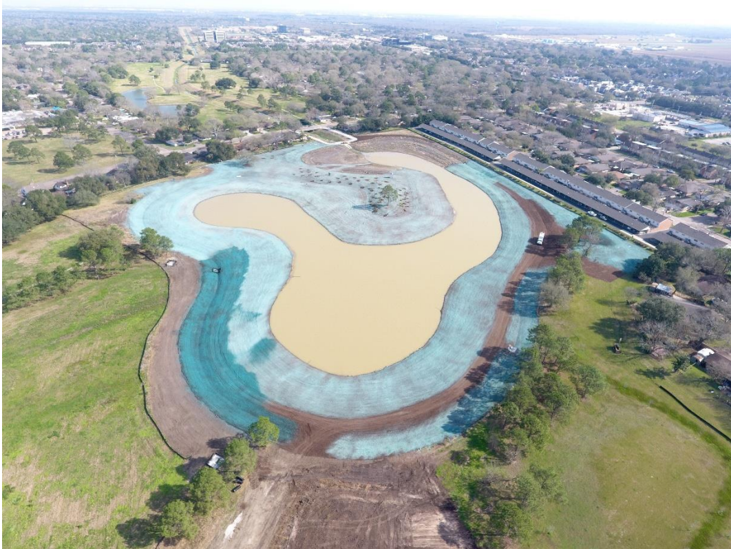
Figure 16. Hydroseeding Phase 1A.
