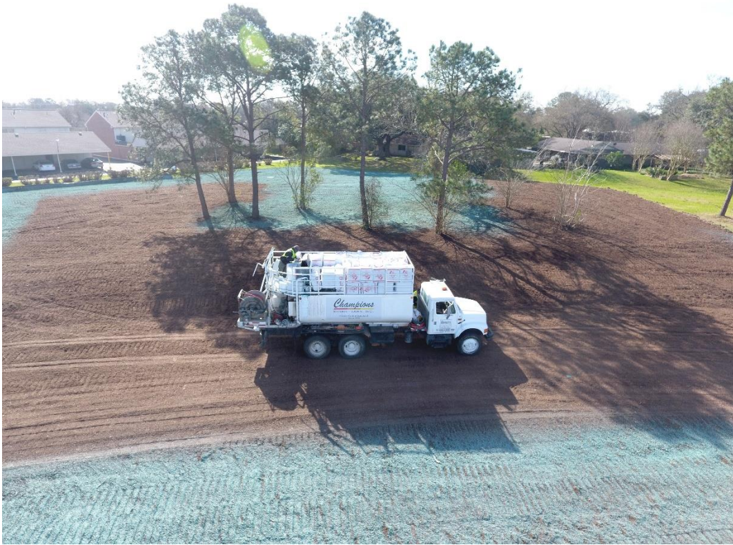
Figure 15. Hydroseeding Phase 1A.
