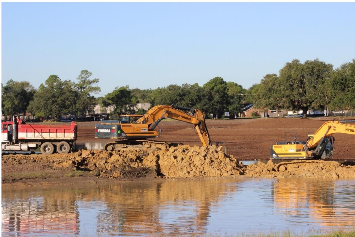
Figure 6. Phase I construction
