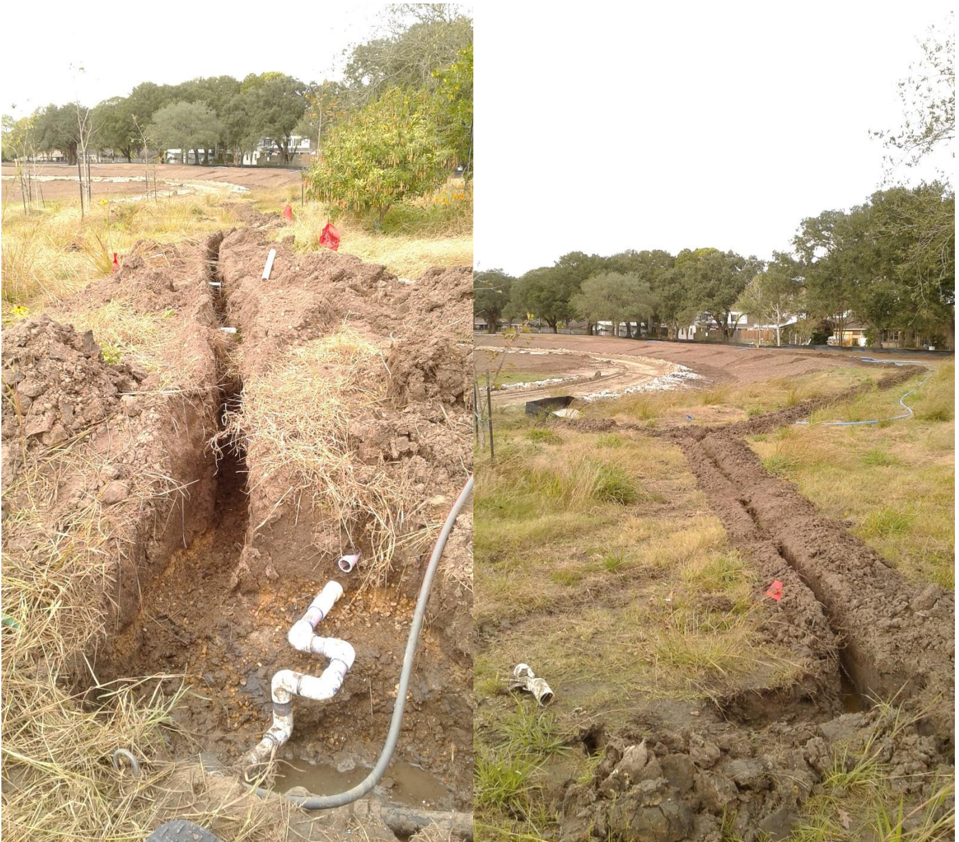
Figure 33. Trenches for irrigation lines to water trees and shrubs.
