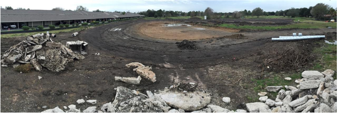
Figure 5. Phase IA excavation
