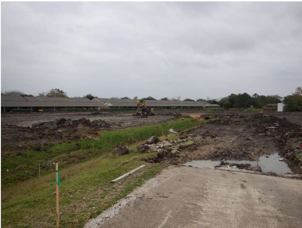
Figure 4. Phase 1A excavation
