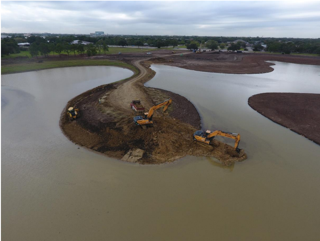
Figure 23. Removal of habitat island land bridge.
