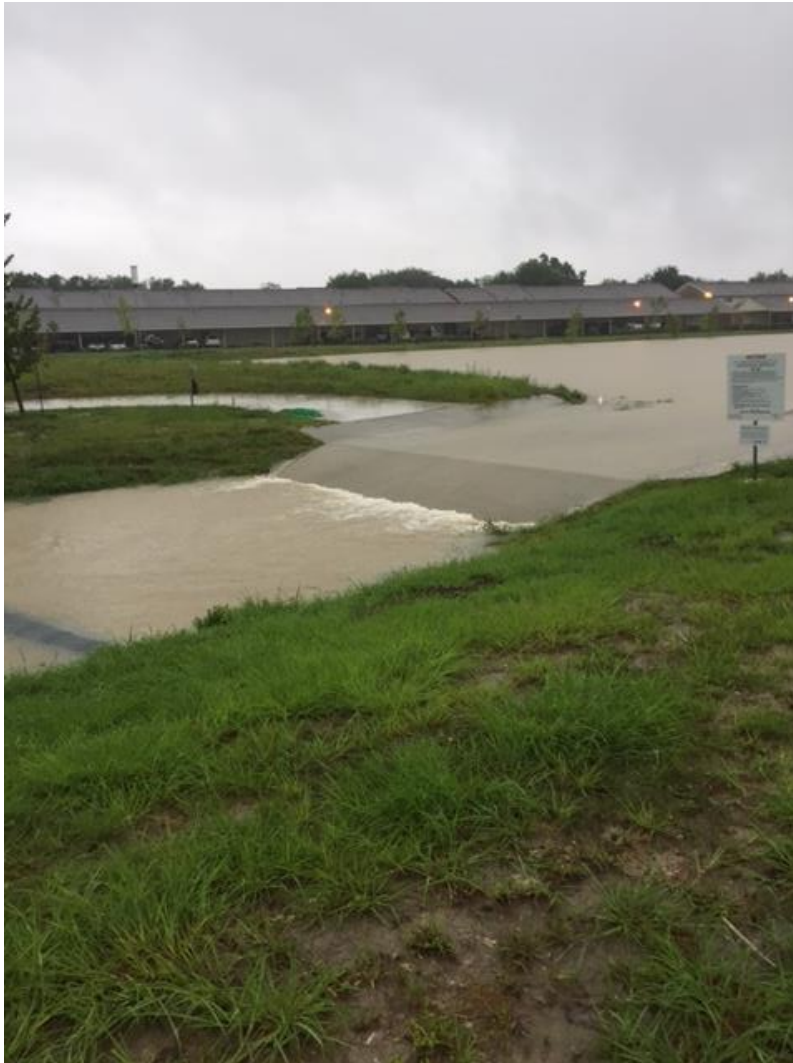
Figure 48. Phase 1A spillway during Hurricane Harvey.
