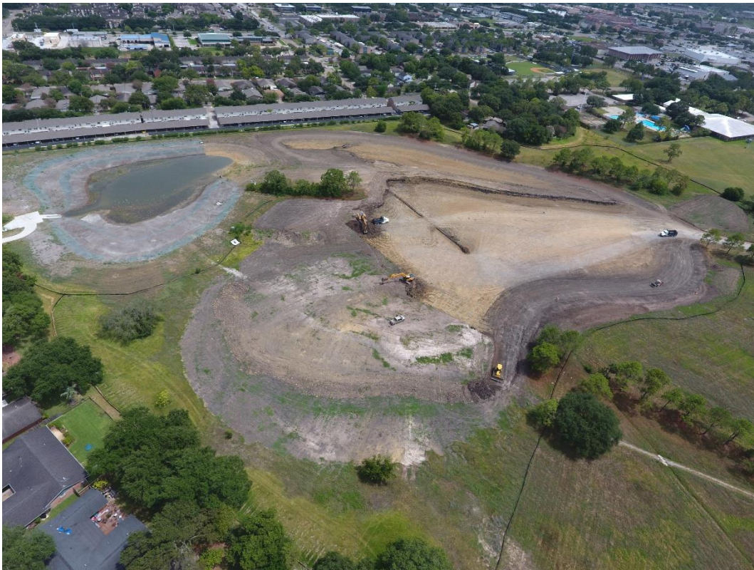
Figure 8. Phase 1B construction site.
