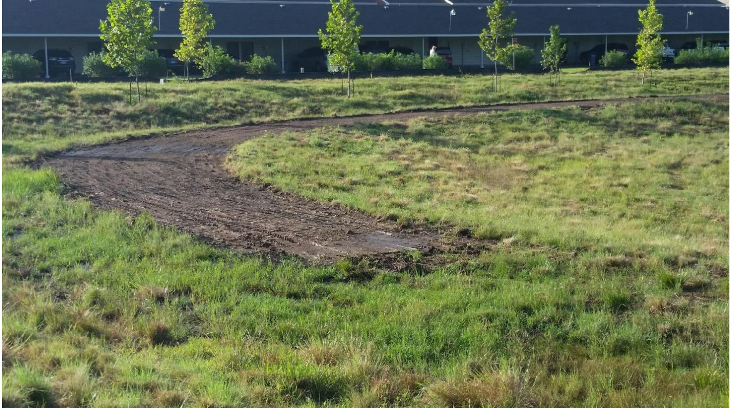
Figure 26. Initial Phase 1 trail construction.
