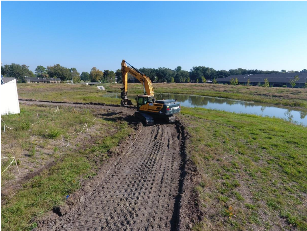
Figure 27. Trail construction around Phase 1A.
