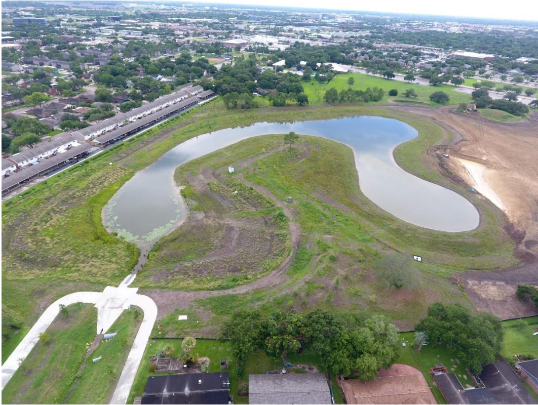
Figure 11. Phase 1A and 1B after seeding and during 1C construction.
