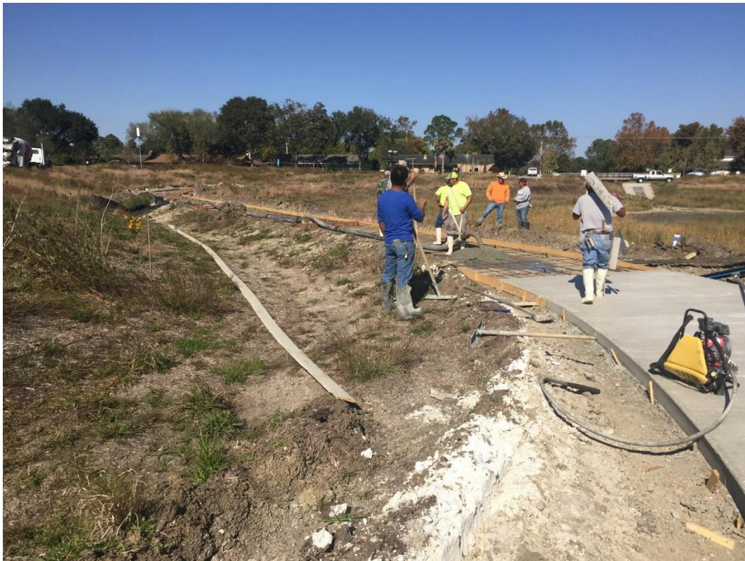
Figure 30. Trail construction, pouring concrete at Phase 1A.
