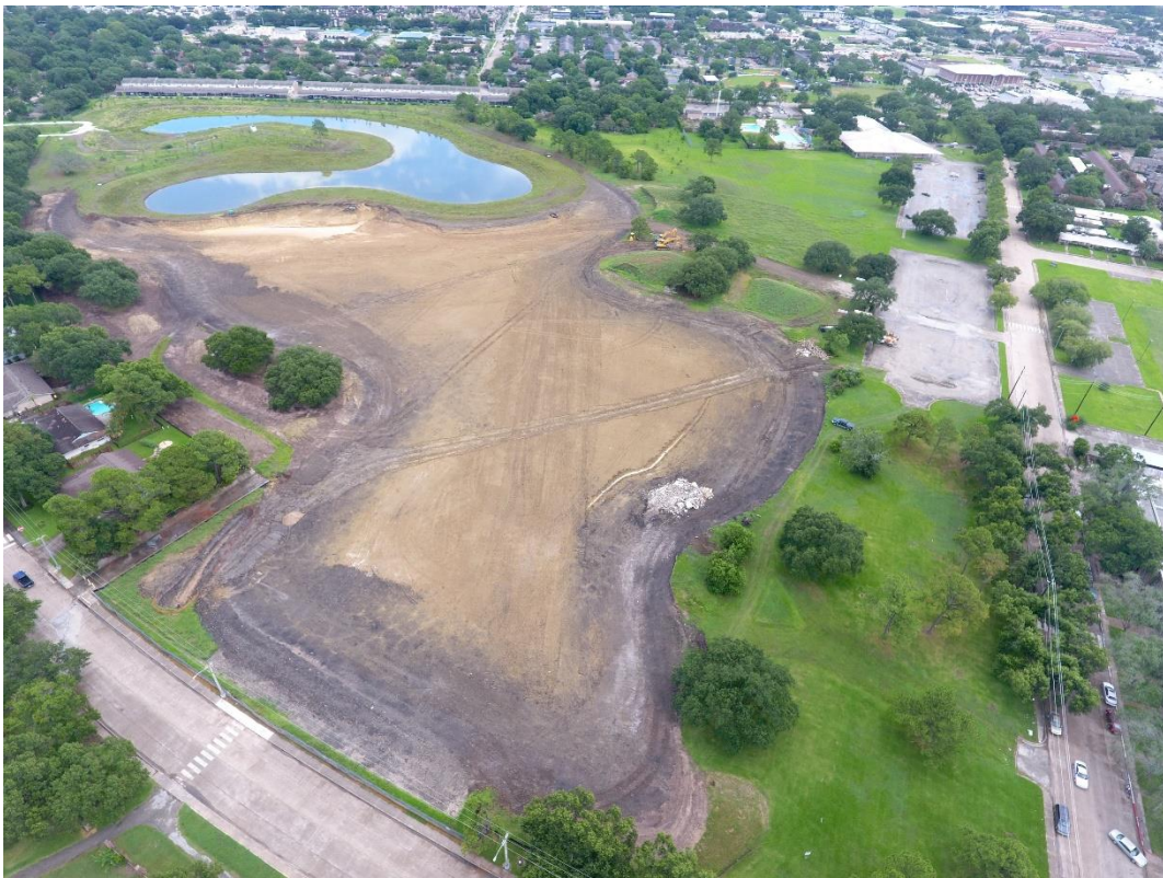
Figure 12. Phase 1C construction
