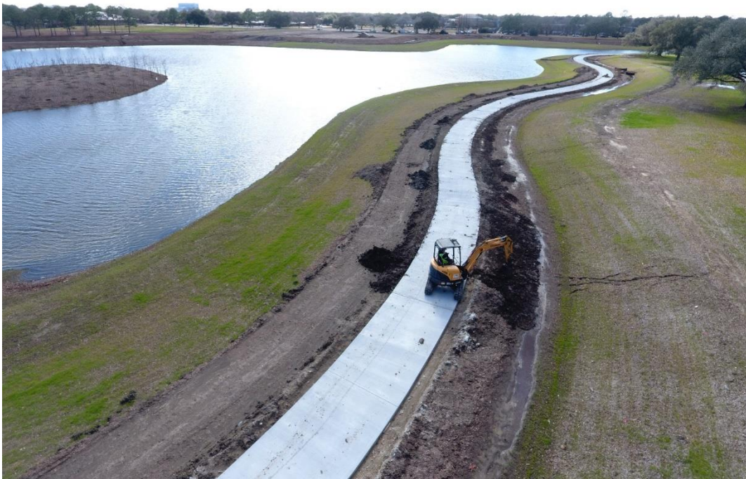
Figure 32. Trail construction Phase 1B.
