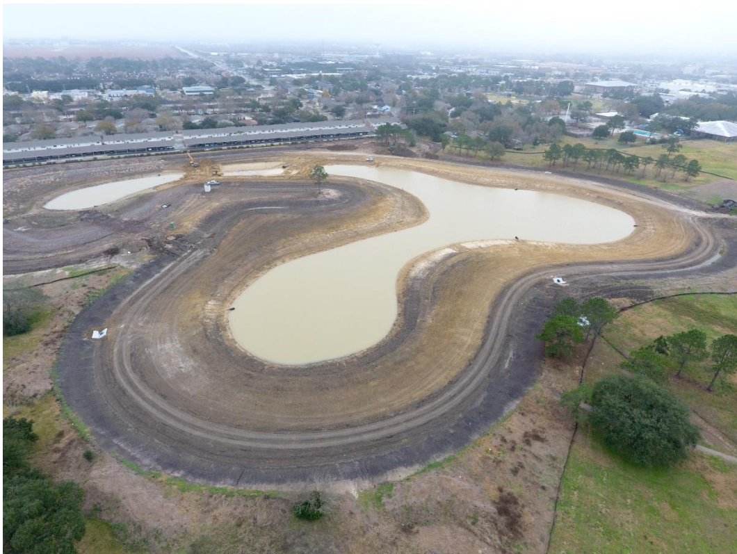
Figure 10. Phase 1A and 1B before 1C excavation.
