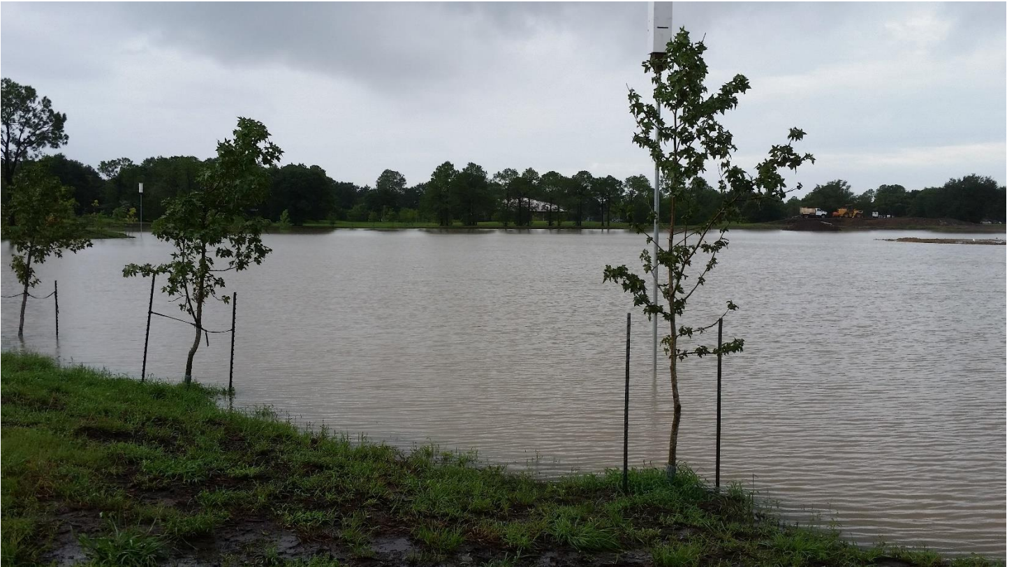
Figure 47. Phase 1 during Hurricane Harvey
