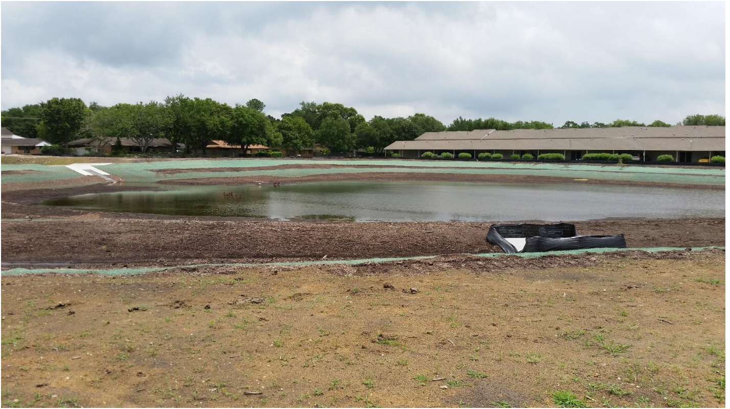
Figure 7. Construction of Phase 1A after seeding.
