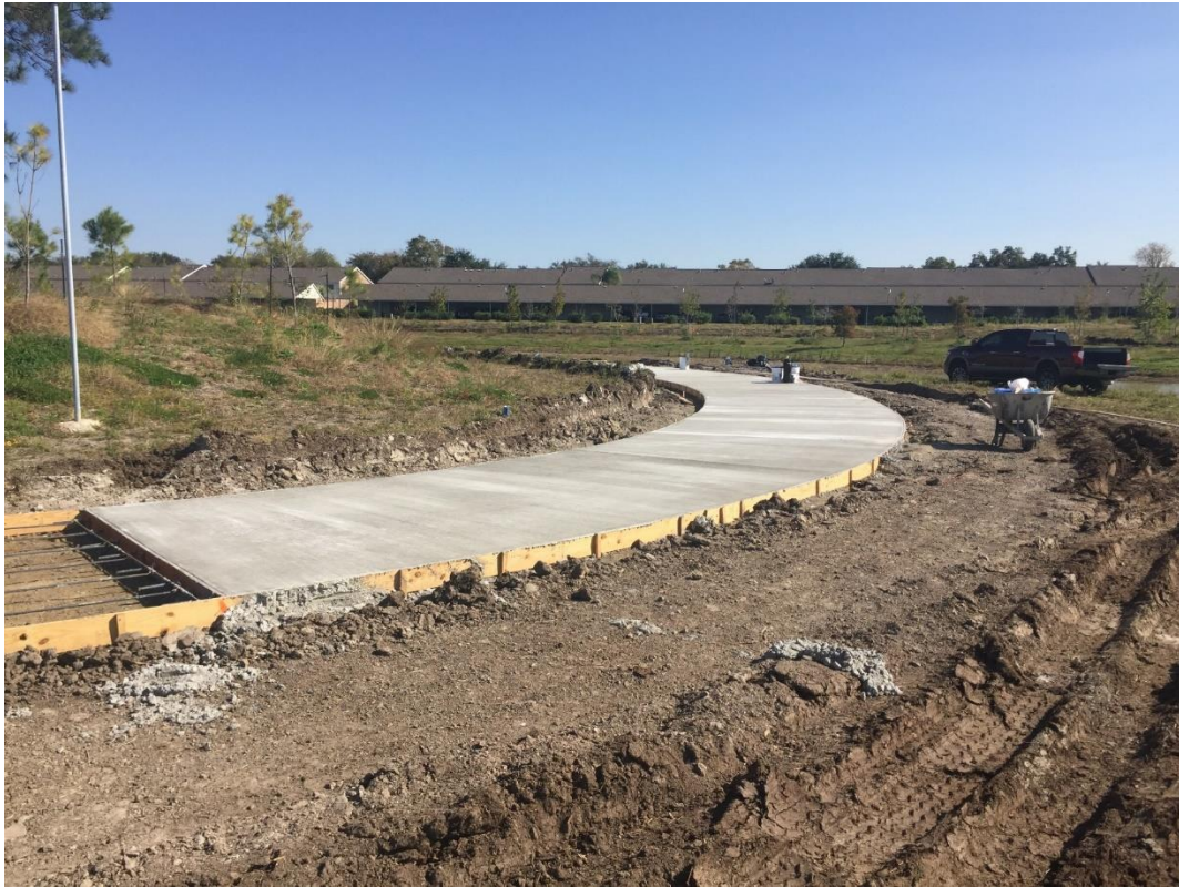
Figure 29. Trail construction with concrete poured.
