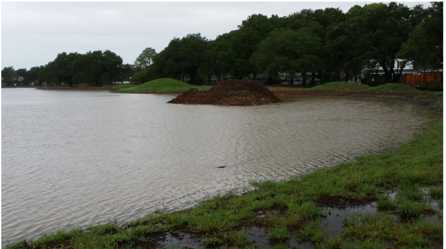
Figure 46. During Hurricane Harvey Phase 1 prevented approximately 150 homes from flooding.
