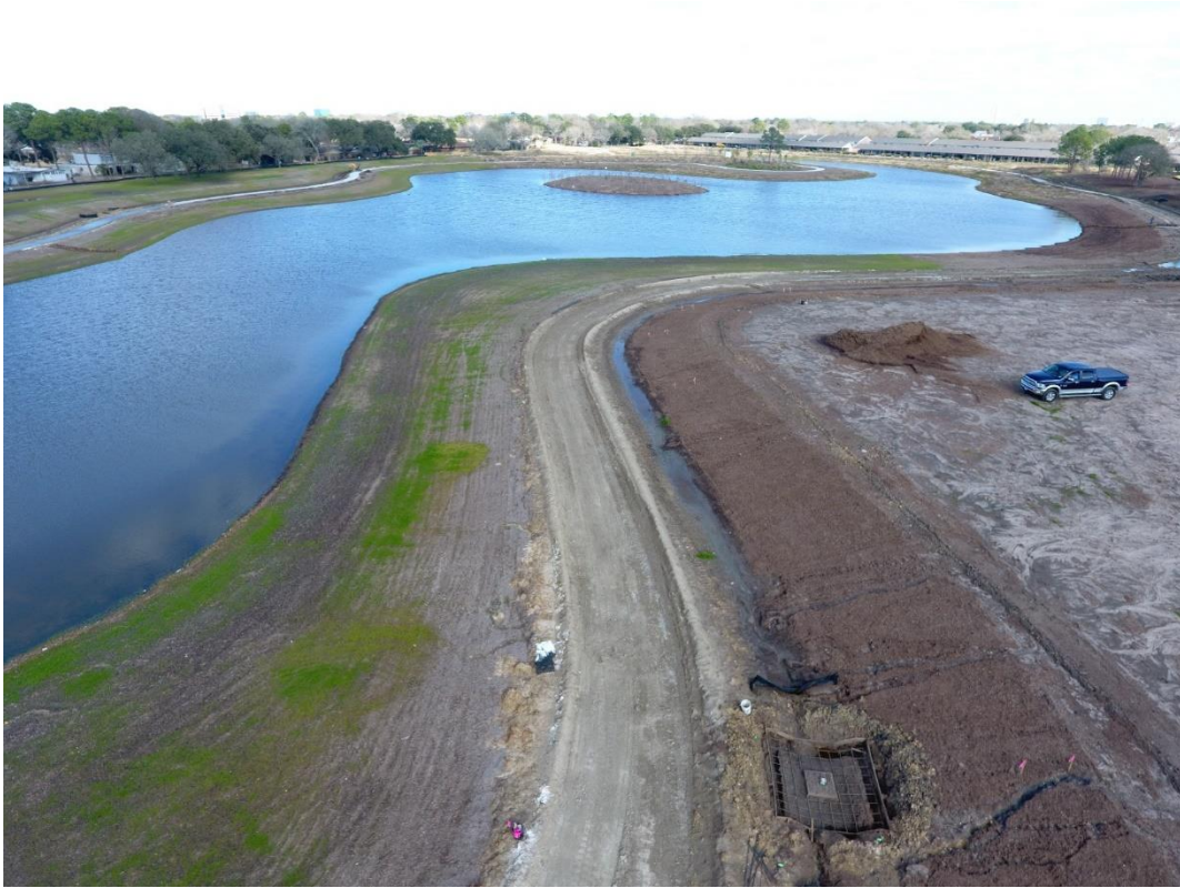
Figure 31. Trail construction phase 1C.
