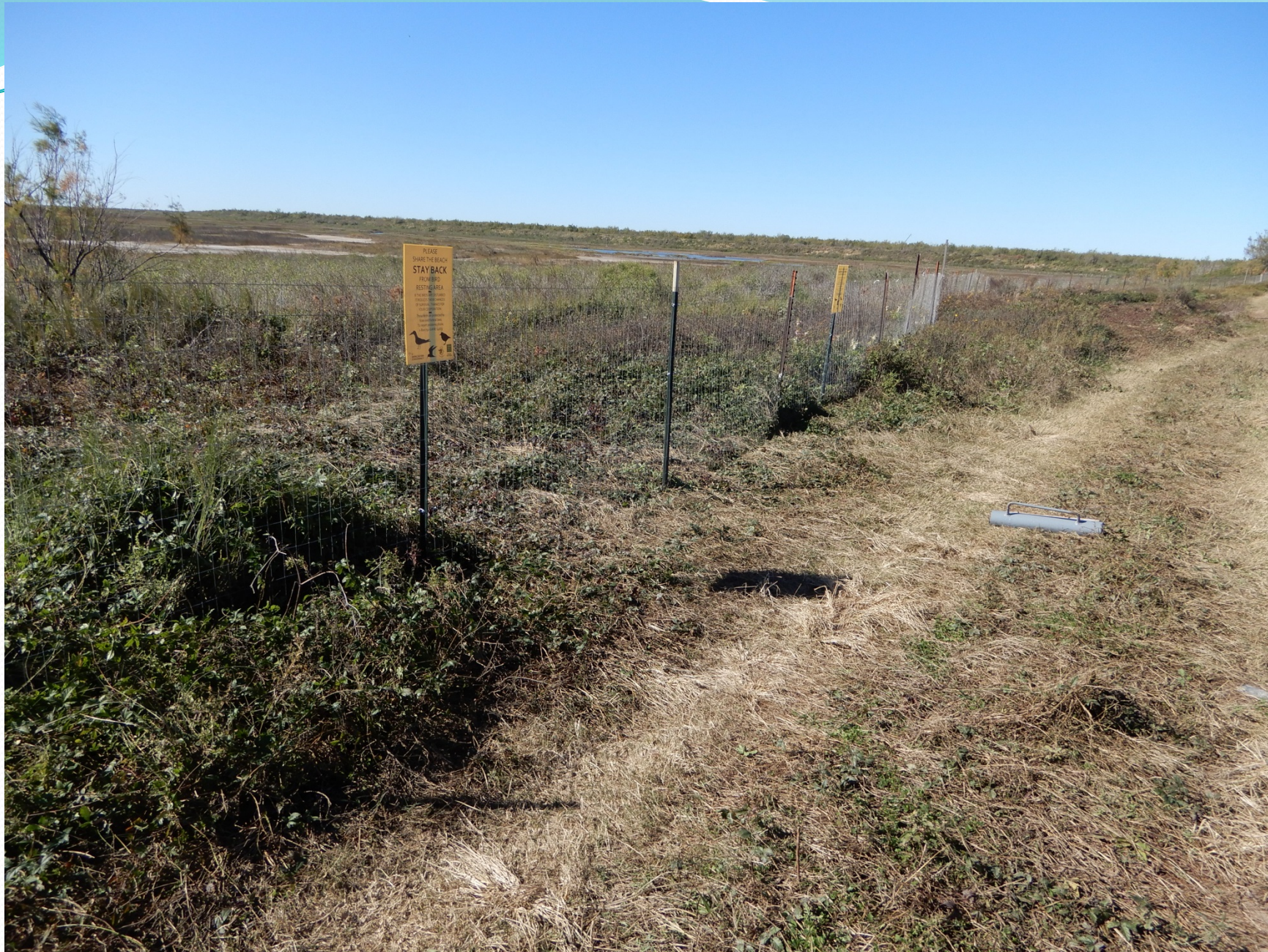
Big Flats fence repaired (Dec 21, 2018)
