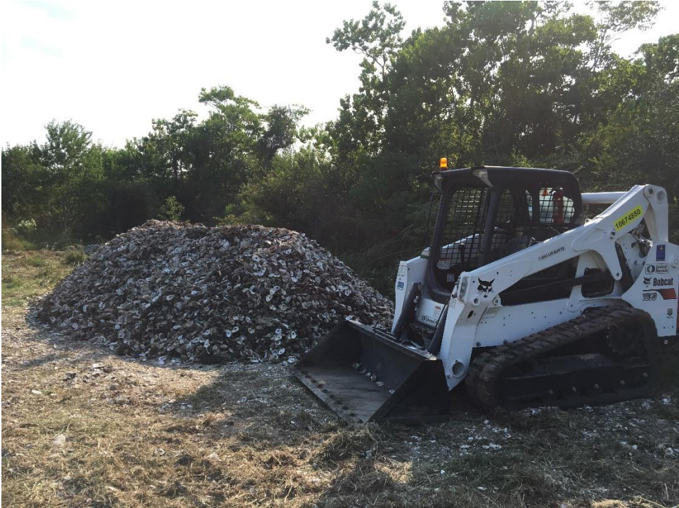
Shell turning and piling
