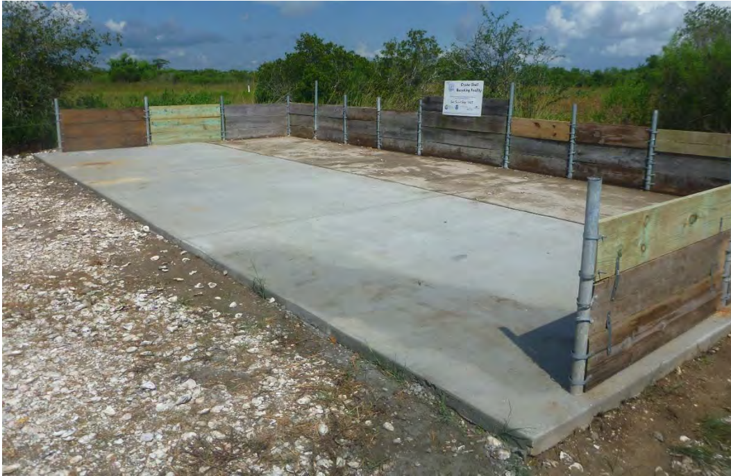
Figure 15. Cement pad at TX City Curing Site.
