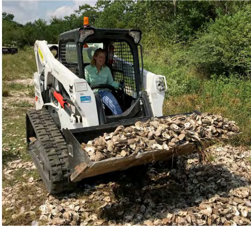
Figure 11. Piling recycled shell at Red Bluff Curing Site.
