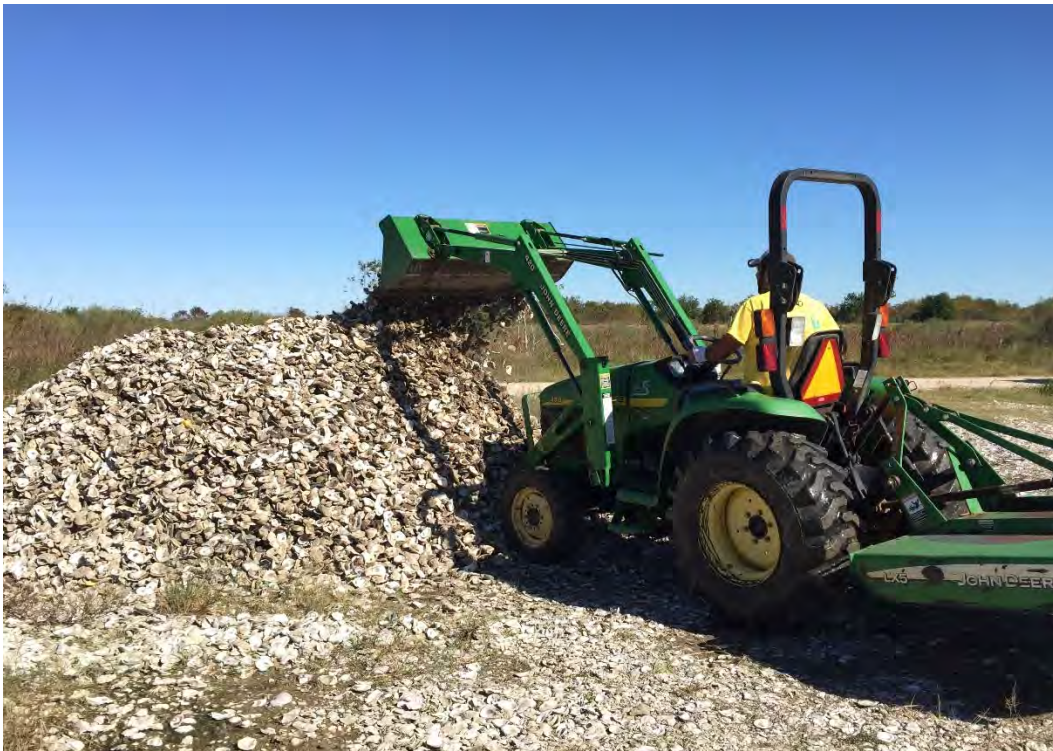
Figure 20. Piling recycled shell at TX City Curing Site.
