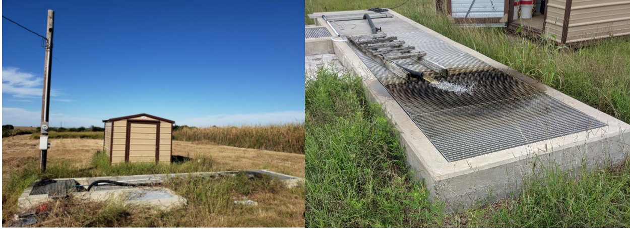
Figure 7. Photos of the Bayside WWTP effluent outfall.
