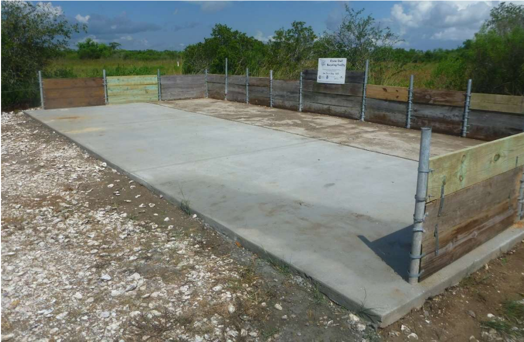
Figure 17. Cement pad at TX City Curing Site.
