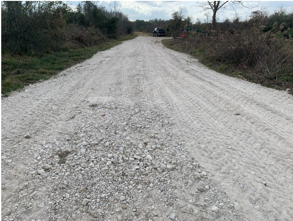
Access road maintenance
