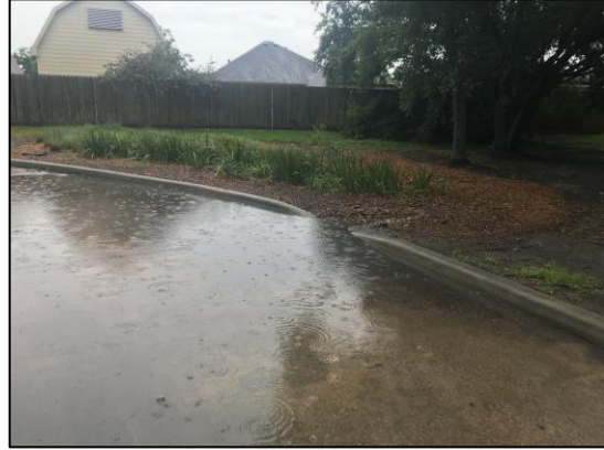
Water flowing from the parking lot through a curb cut into a rain garden, one of the GI practices in action during the field day
