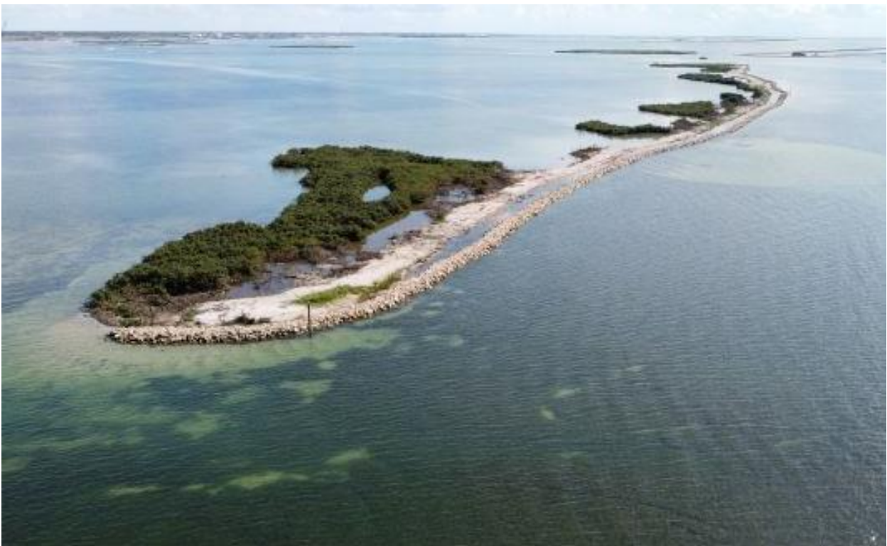
Figure 10. South Dagger Island Breakwater - south to north - after construction (August 2020)
