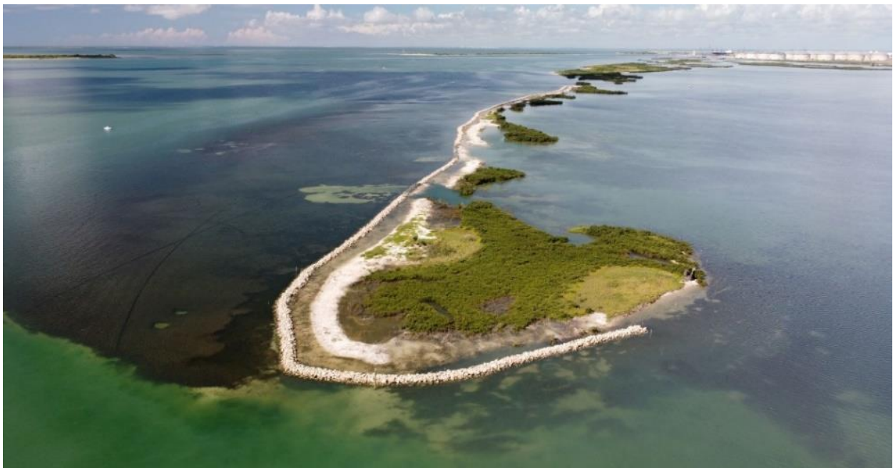
Figure 8. South Dagger Island breakwater - north to south - after construction (August 2020).
