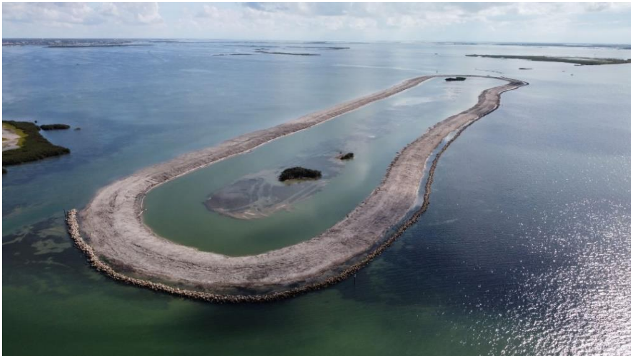
Figure 12. Breakwater and beneficial use site after construction (August 2020).
