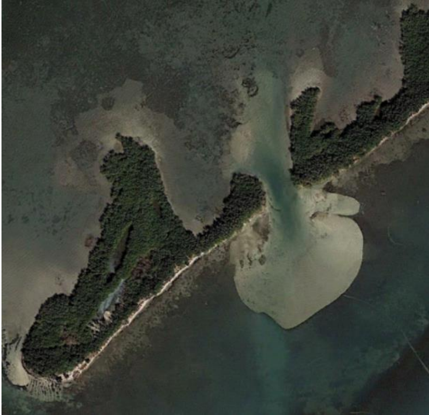
Figure 9. South Dagger Island breakwater - south to north - before construction (January 2020).
