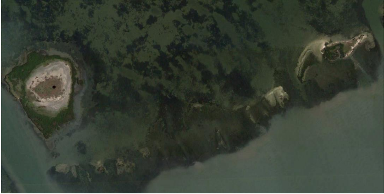
Figure 11. Breakwater and beneficial use site before construction (2017).
