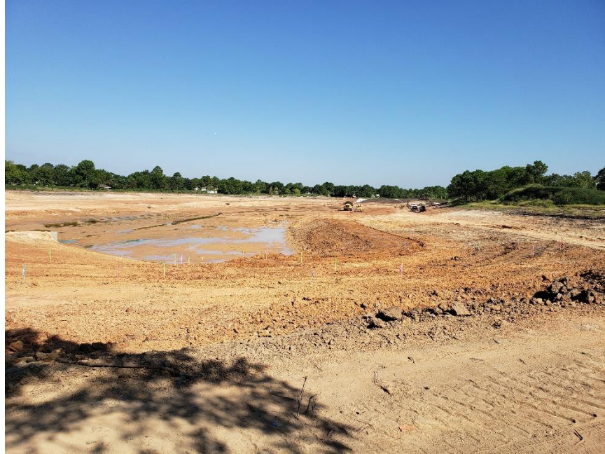
Photograph 5. During construction photograph taken July 2020.
