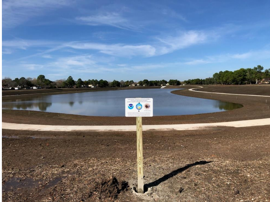
Photograph 19. Permanent sign at South entrance of Phase 3A.
