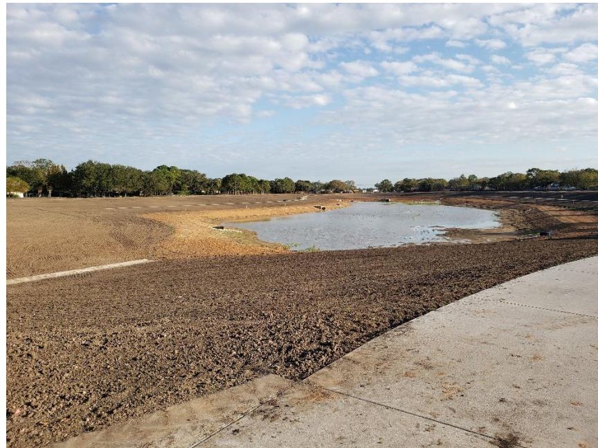
Photograph 6. During construction photograph taken November 2020.
