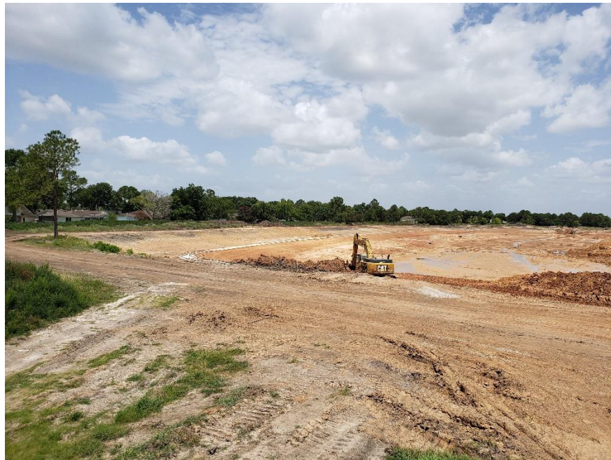
Photograph 4. During construction photograph taken July 2020.
