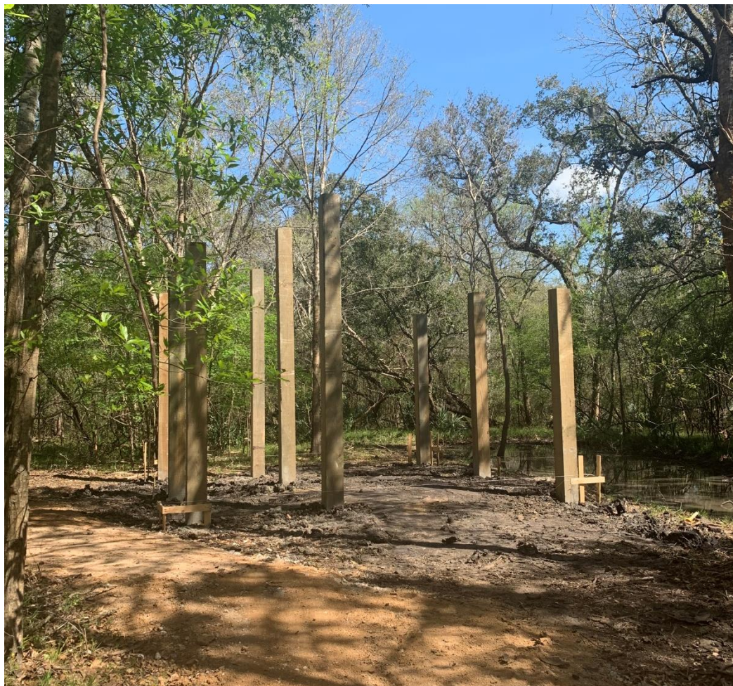
Pilings for Observation Deck
