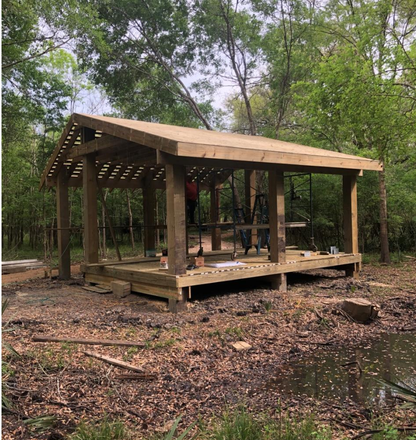
Construction of Observation Deck
