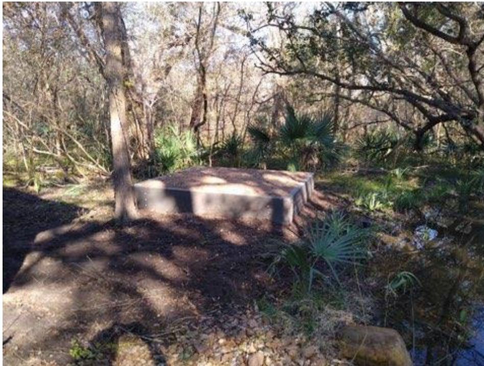
Concrete pad for Rain Water Harvesting System
