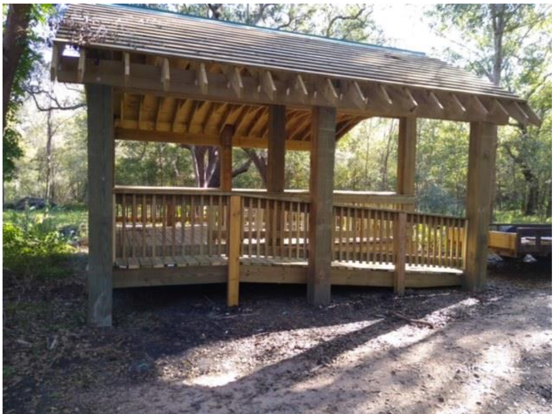
ADA Ramp Built for access to Observation Deck
