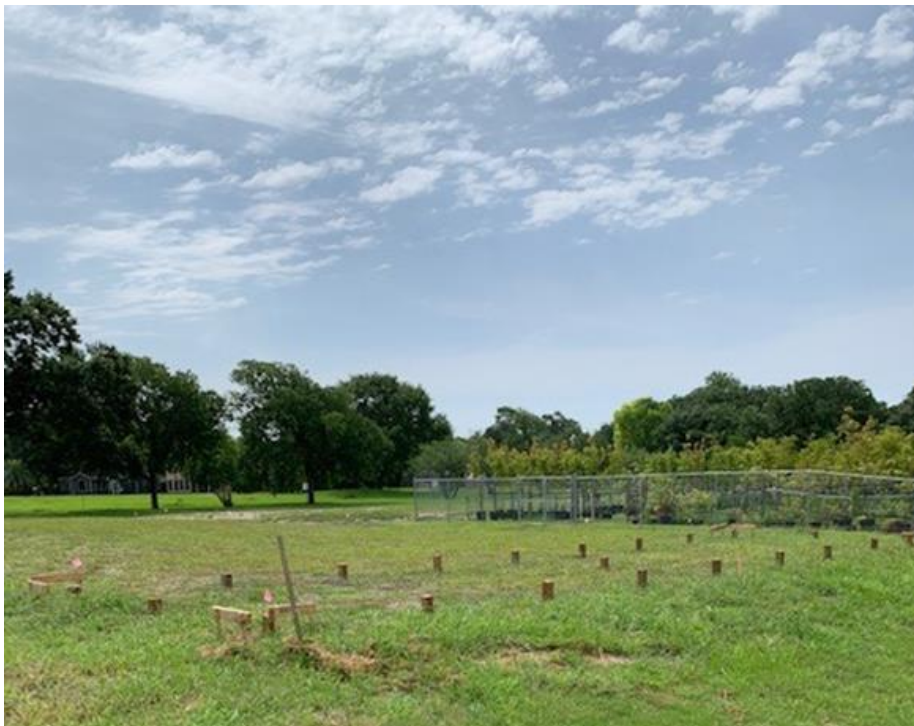
Figure 21: Initial framing of the on grade nursery tanks.
