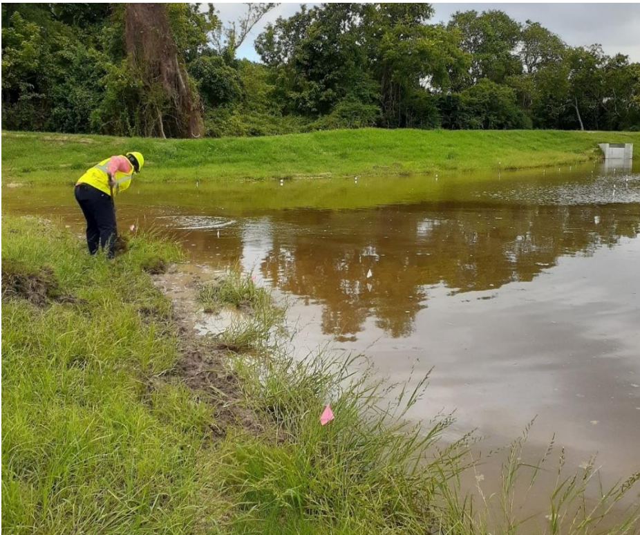
Figure 16: Coastal Bermuda grass sod around waterline of Stormwater basin.
