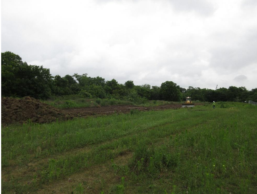
Figure 5: Harvey Construction beginning excavation 05/07/2019.
