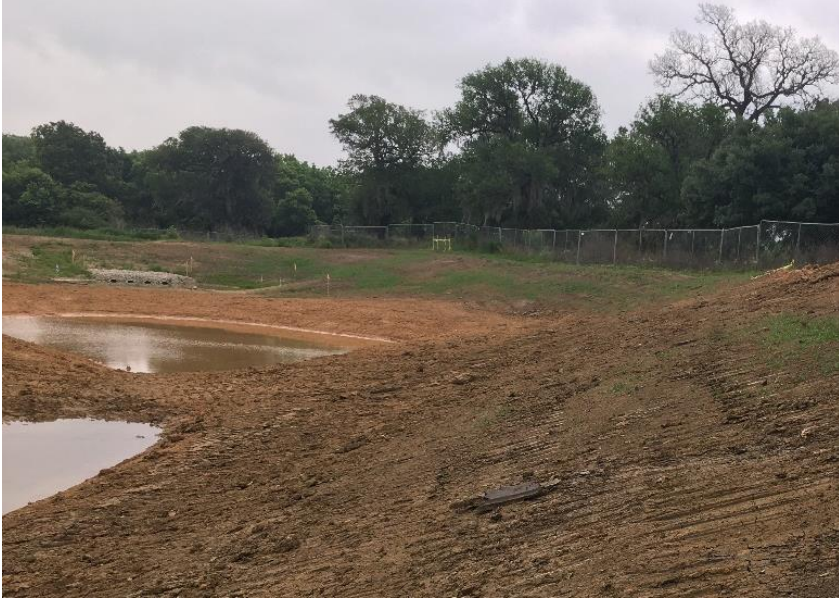
Figure 11: Culvert installed underneath the land bridge connecting basin 2 and 3.
