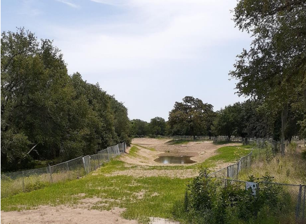
Figure 9: Final as built grading of the Stormwater Wetlands 06/10/2020.
