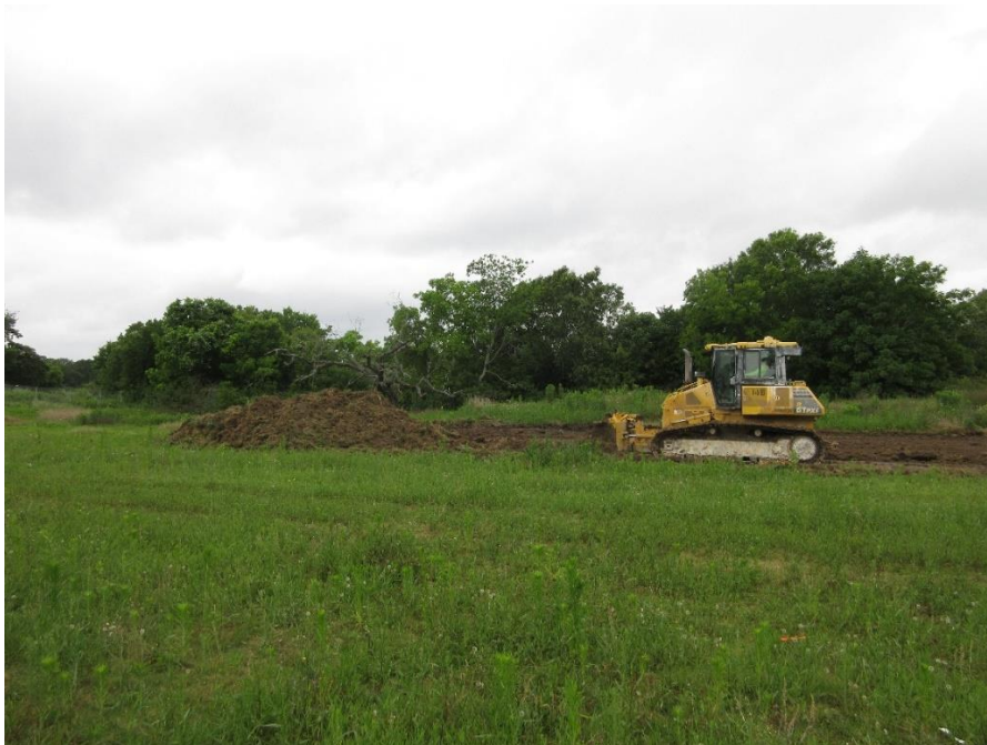
Figure 6: Harvey Construction beginning excavation 05/07/2019.
