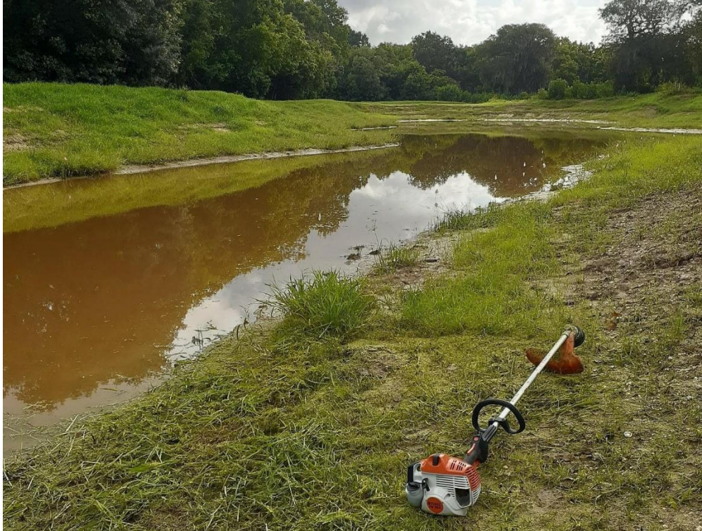
Figure 17: Coastal Bermuda grass sod around waterline of Stormwater basin.
