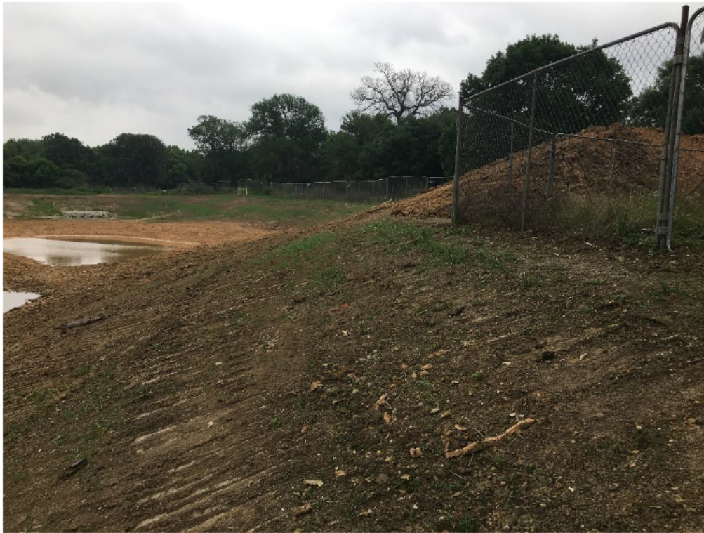
Figure 8: Final as built grading of the Stormwater Wetlands 04/22/2020.
