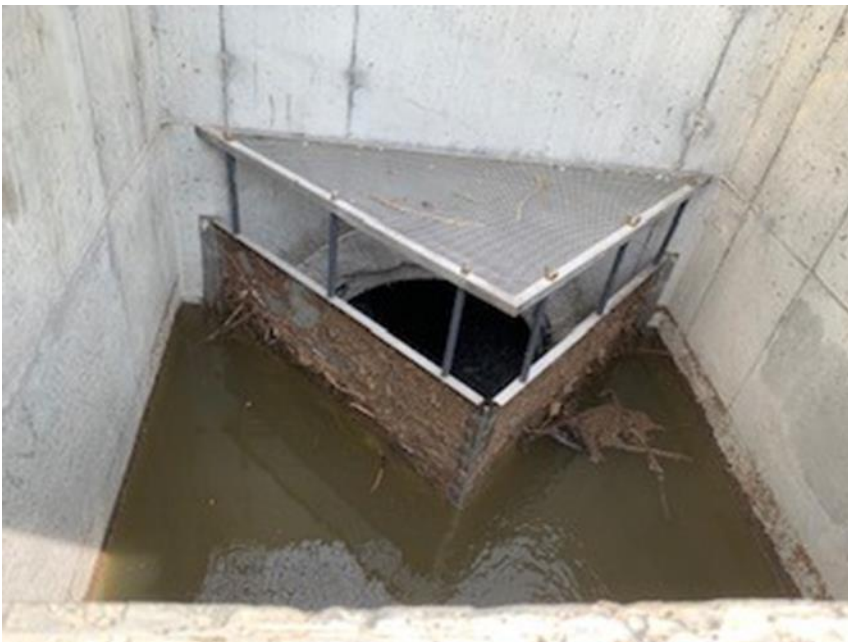
Figure 14: Cleaning grate at the outfall structure.
