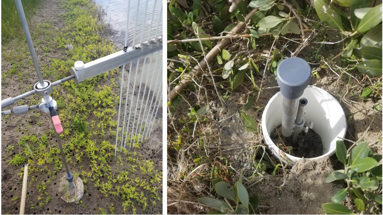
Figure 3a (left) the removable arm sitting on the collar (held steady by pink clamp), with the collar attached to the permanent receiver. 2b (right) the permanent receiver attached to the uppermost steel rod shown before cement is added to fill the hole. Picture on the left shows the pvc core after the receiver is cemented in. The photograph of the arm was taken at our Padre Island National Seashore site, and the receiver (right) is from our Boggy Creek / Port O'Connor site.
