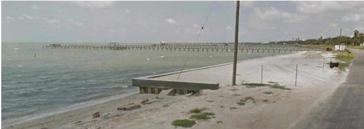
Figure 7. Google Street View Photo from 2018 showing a private sheetpile bulkhead and concrete cap along North Fulton Beach Road.
