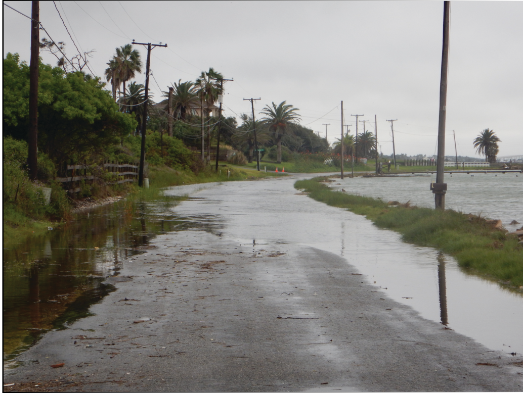
Fulton Beach Road, Facing North— September 26, 2020
