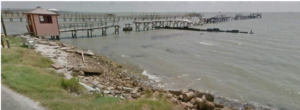
Figure 10. Google Street View Photo from 2018 showing privately leased timber piers and an offshore band on concrete rip rap along North Fulton Beach Road.
