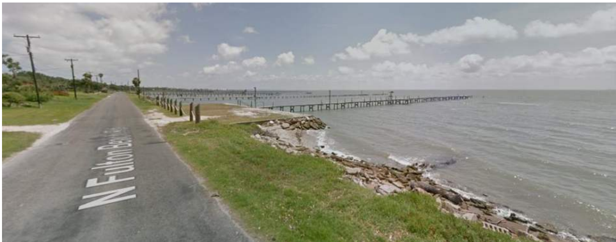
Figure 8. Google Street View Photo from 2018 showing a privately leased bulkhead and timber pier along North Fulton Beach Road.
