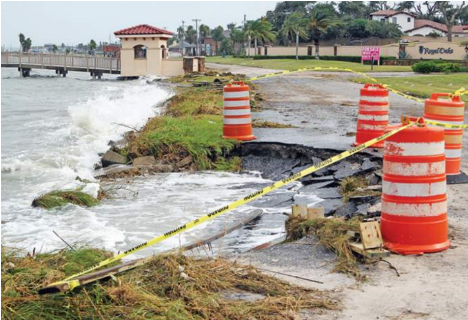
Figure 3. Damage at North Fulton Beach Road from Hurricane Hanna in July 2020 (Rockport Pilot, 2020).
