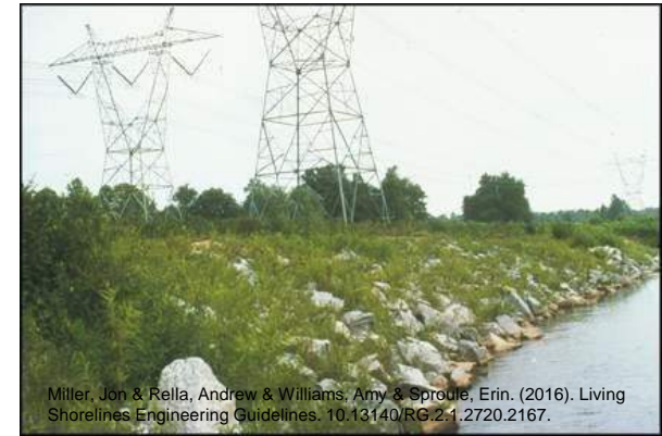
Figure A6. Example Joint Planting with Stone Revetment Design
