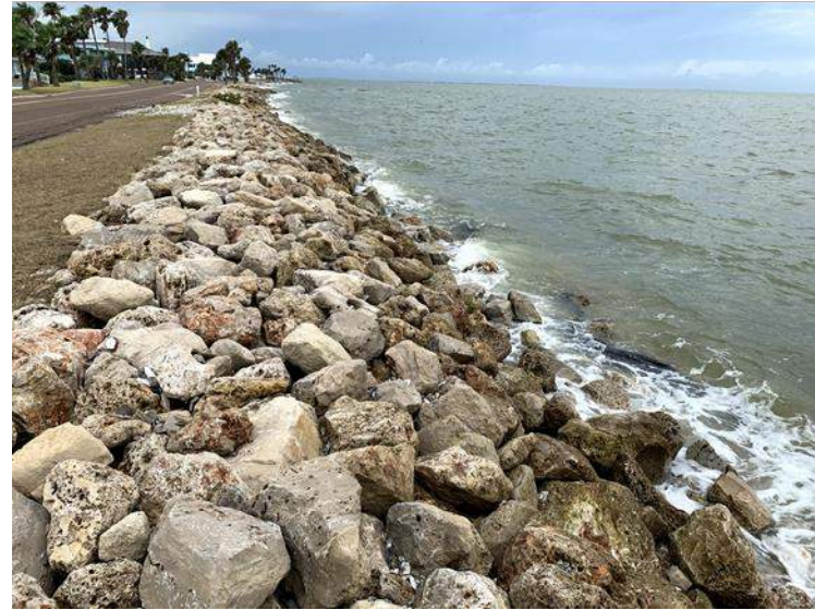
Figure A1. Stone Revetment Along Bayshore Drive Rockport, TX
