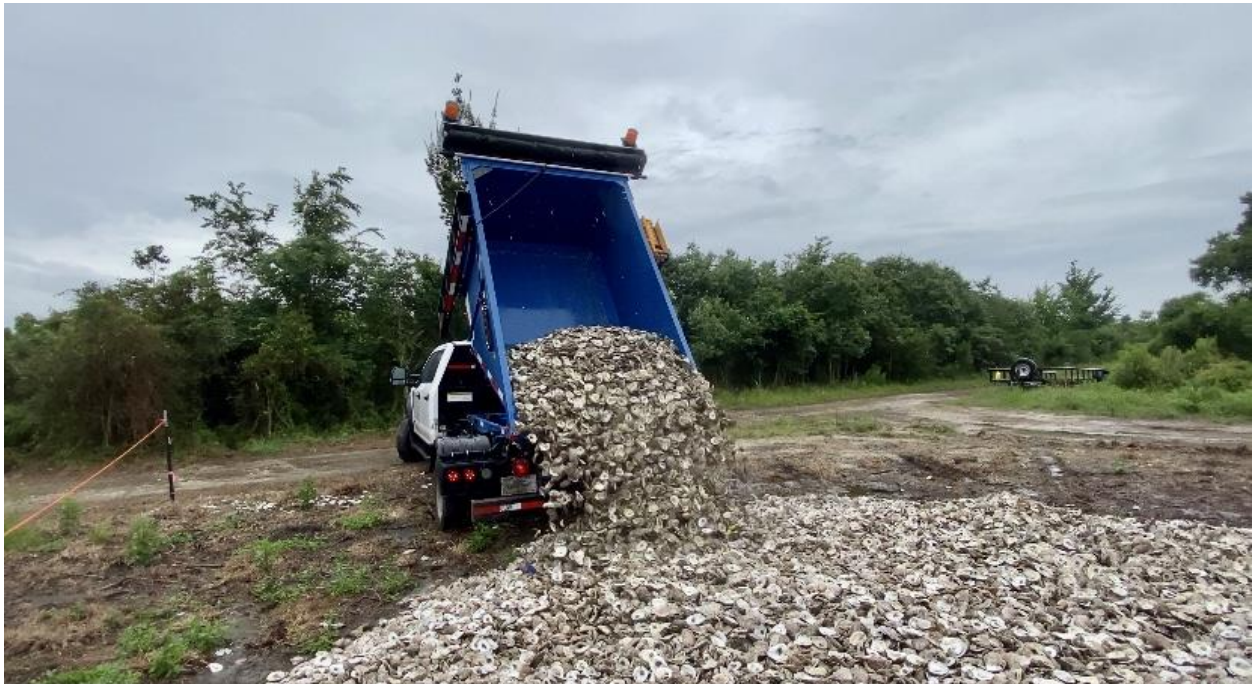
Figure 8. Recycled shell being delivered to the Red Bluff curing site with the new equipment.
