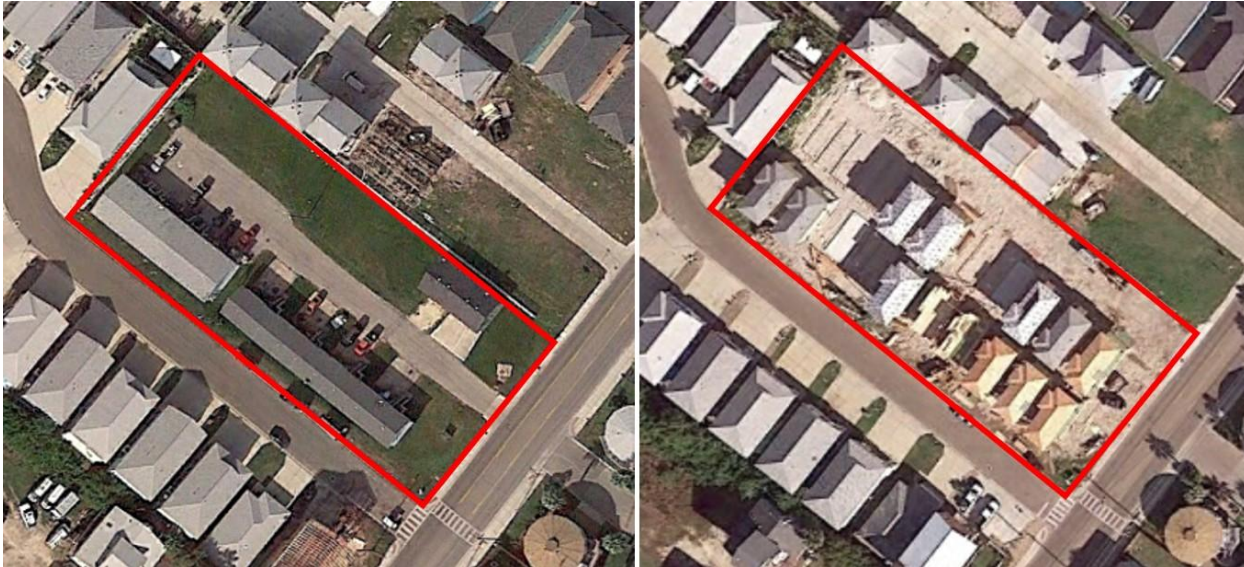
Due to hurricane damages, many lots in Port Aransas were sold and re-developed post-Harvey. This lot on Eleventh Street was converted from a small apartment unit with grass (left Jan. 2017) to 18 small vacation homes(right Jan. 2020; photo credit: Google Earth).
