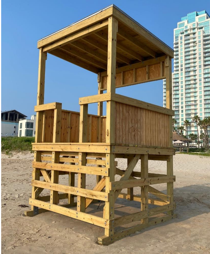
Figure 1. Initial Tower Construction
