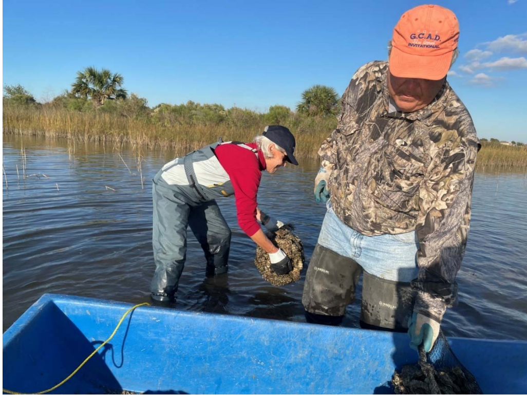
Figure 12. Volunteers placing oysters and recycled shell onto Sweetwater Lake Oyster Shell Breakwater (Fall 2021)
