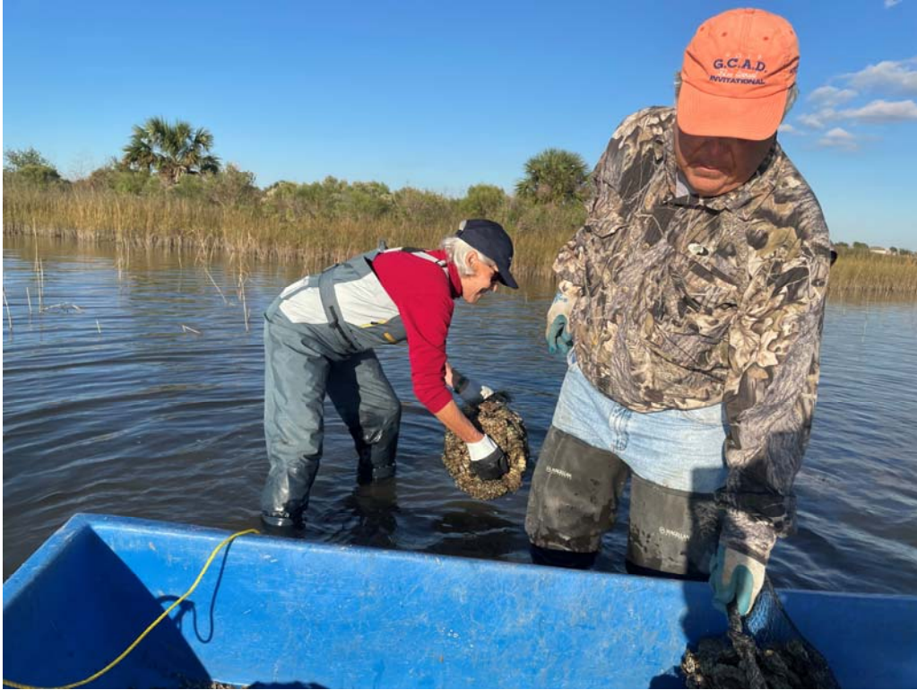
Figure 12. Volunteers placing oysters and recycled shell onto Sweetwater Lake Oyster Shell Breakwater (Fall 2021)
