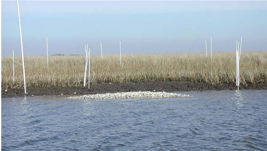
Figure 1. Cultched shoreline created at Sister Lake, Louisiana, showing intertidal oyster reef ( 25 \times 1.0 \times 0.7 m). Each reef was created with 17.5 \text{ m}^3 of shucked oyster shell.
