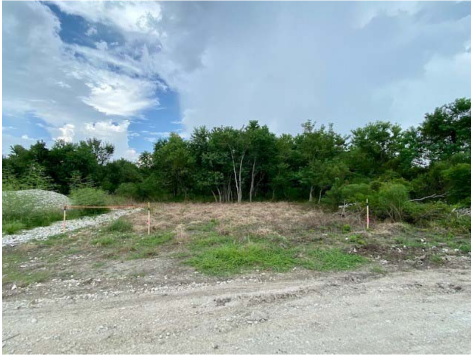
Figure 5. Installed t-posts, rope, and stakes with pile letter for shell piles D and M at Red Bluff curing site
