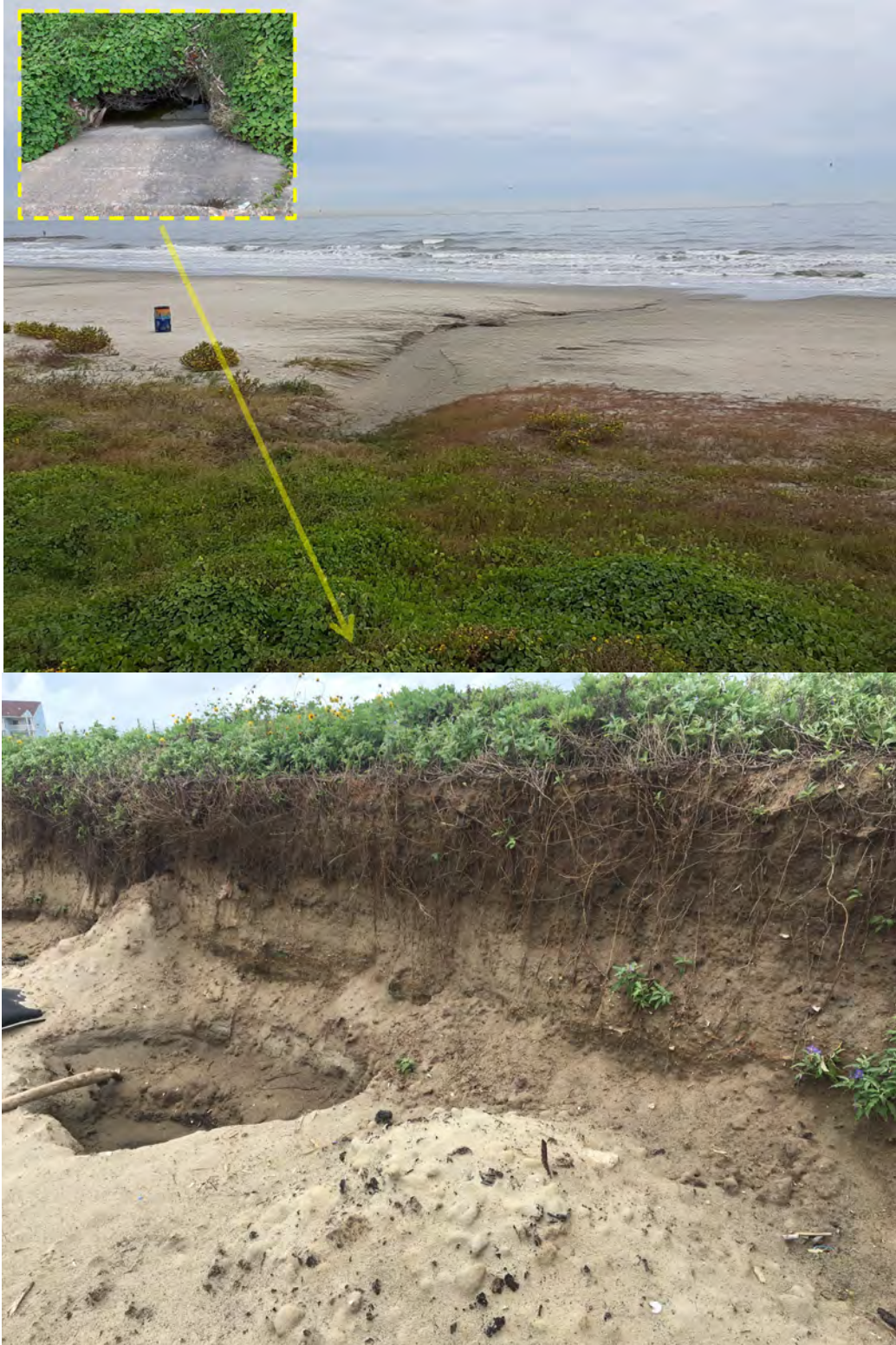
Figure 3. Photos of a runoff scour channel at the seaside toe of the Galveston Seawall (top) and a runoff scour hole at the base of the dune scarp at the Central Beach site. Photos by Youn-Kyung Song (top, date: 03-22/2021) and Jacob Garret (bottom, date: 07-08-2021).
