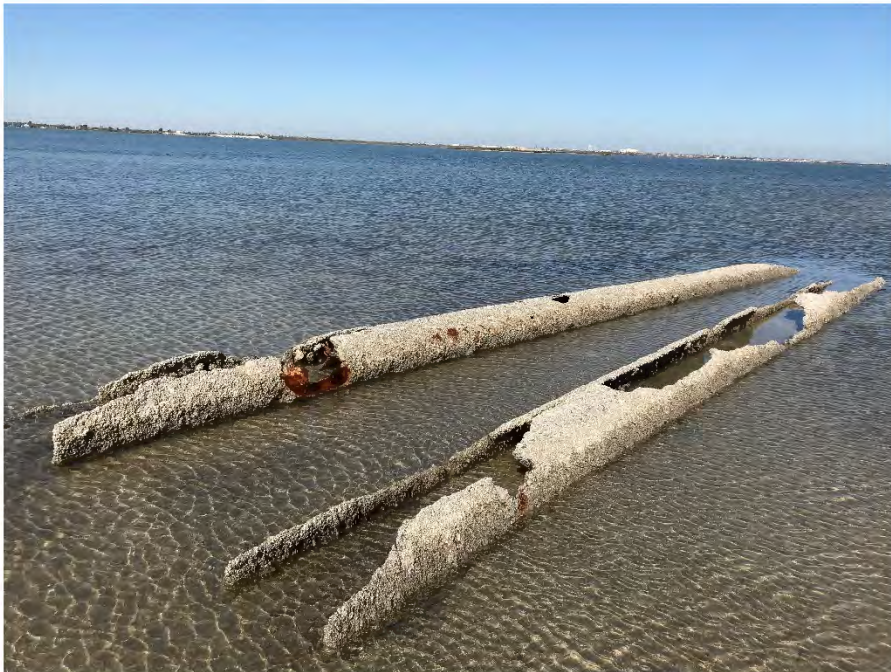
Photo 2 – Submerged debris observed between T1 and T2 located north of Tern Rookery Island and facing north.
