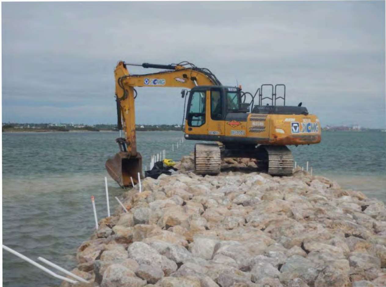
Figure 15. End-on breakwater construction
