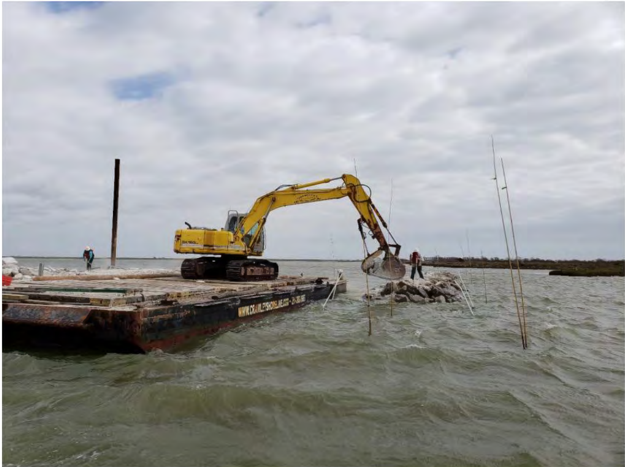
Figure 14. Breakwater construction by light loaded barges
