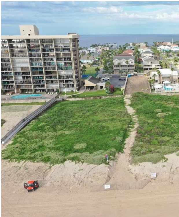
Figure 4. Sloping and sand placement
