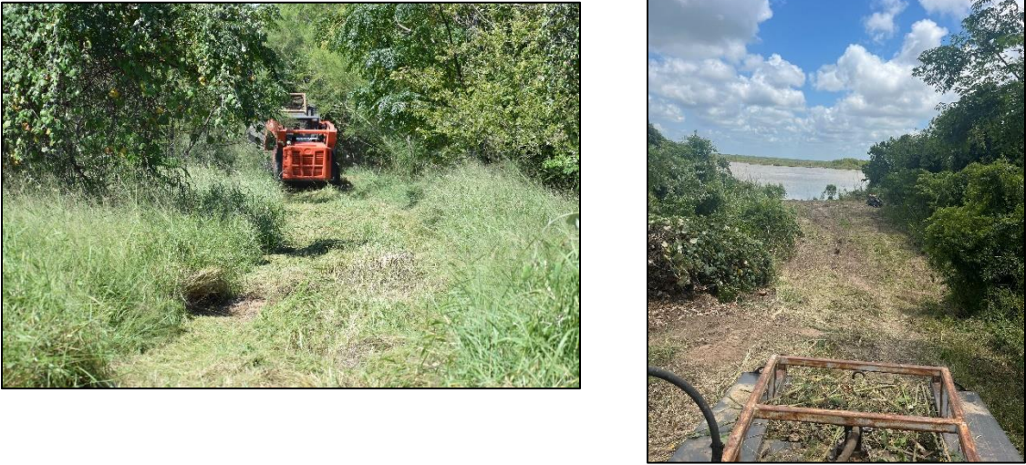
Figure 16 Initial trail clearing.
