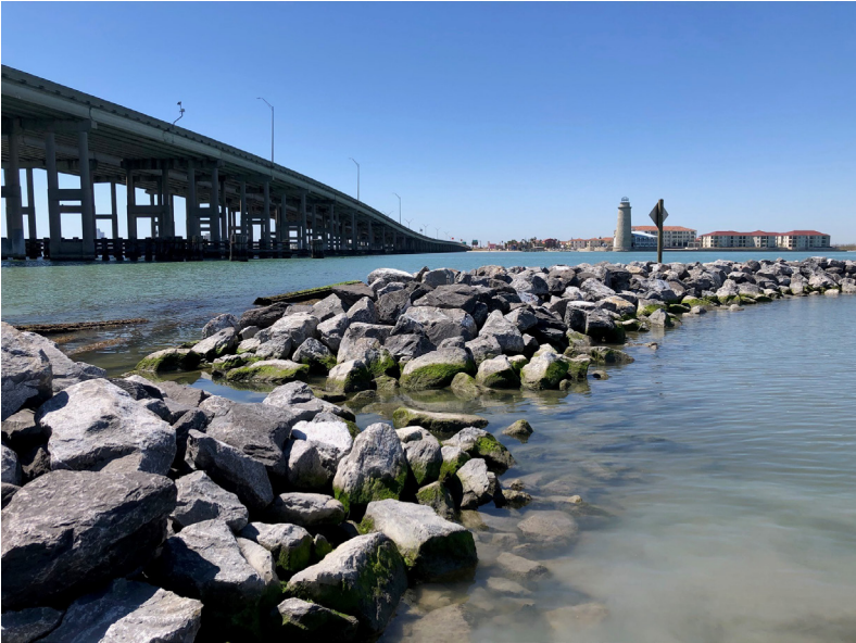
Existing rubble mound breakwater (photo credit: Ducks Unlimited)
