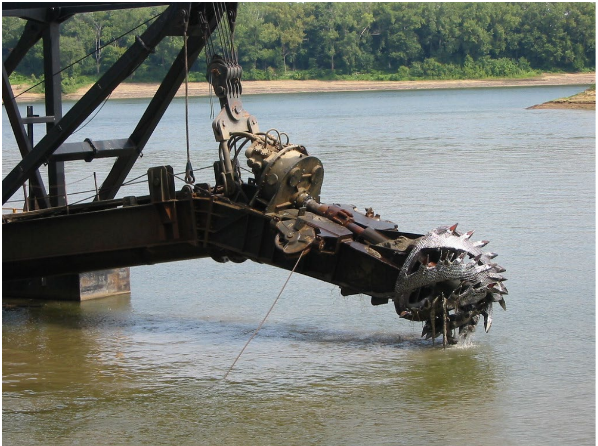
Photograph 2 Representative Hydraulic Dredging
