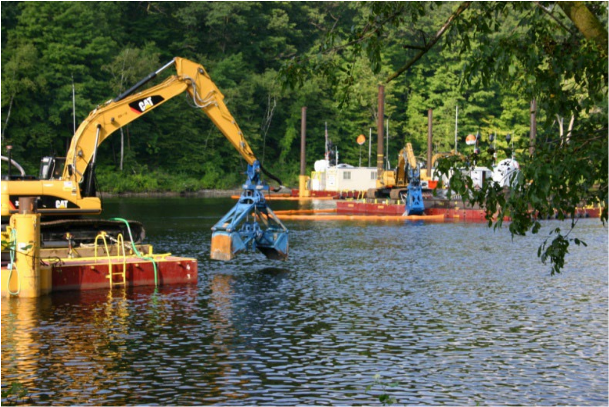
Photograph 1 Representative Mechanical Dredging
