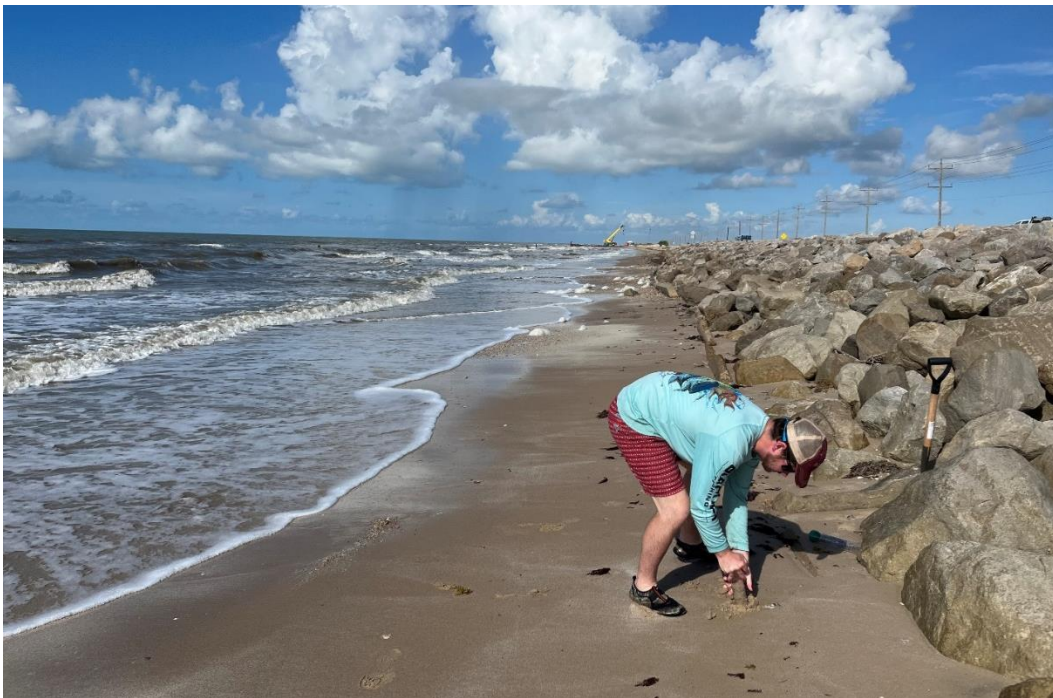
Figure 27. Riprap Revetment at Transect 2 in Bolivar Peninsula East
