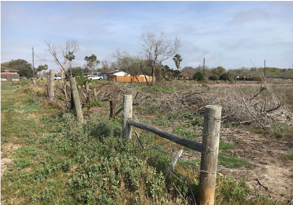
Photo 10. Redhead Pond fence line Section 1 – “After” chainsaw cutting.
