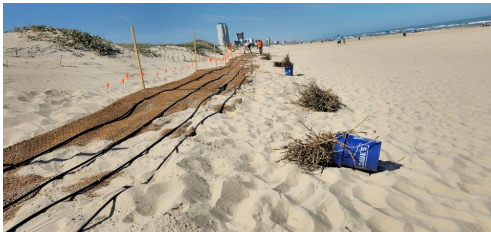
Figure 6.1: Installation of fiber mat and drip irrigation on the foredune (February 24, 2024).
