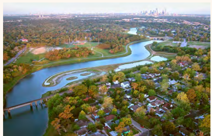
Figure 3: Photo of completed stormwater wetland at Mason Park adjacent to Brays Bayou in Houston, Texas. Photo credited to Harris County Flood Control District Project Brays.
