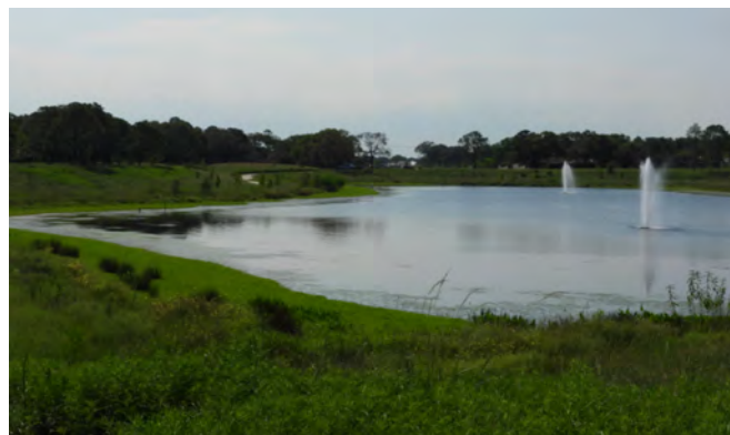
Figure 8: Aerator fountains in Phase 3A of Exploration Green. Photograph provided by Jason Miles.
