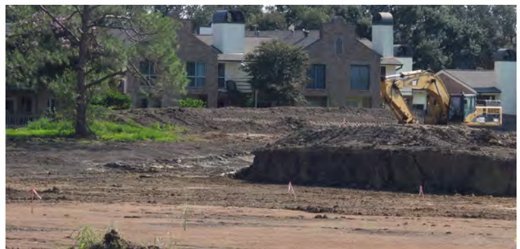
Figure 19: Photo depicts construction at Exploration Green note the grade stakes in the foreground. Photo courtesy of Jason Miles.
