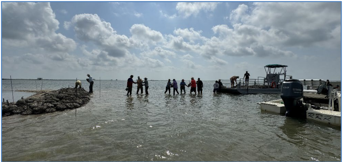
Photo 6: Volunteers unloading shell bags from barge and placing them on the staked-out reef footprint.
