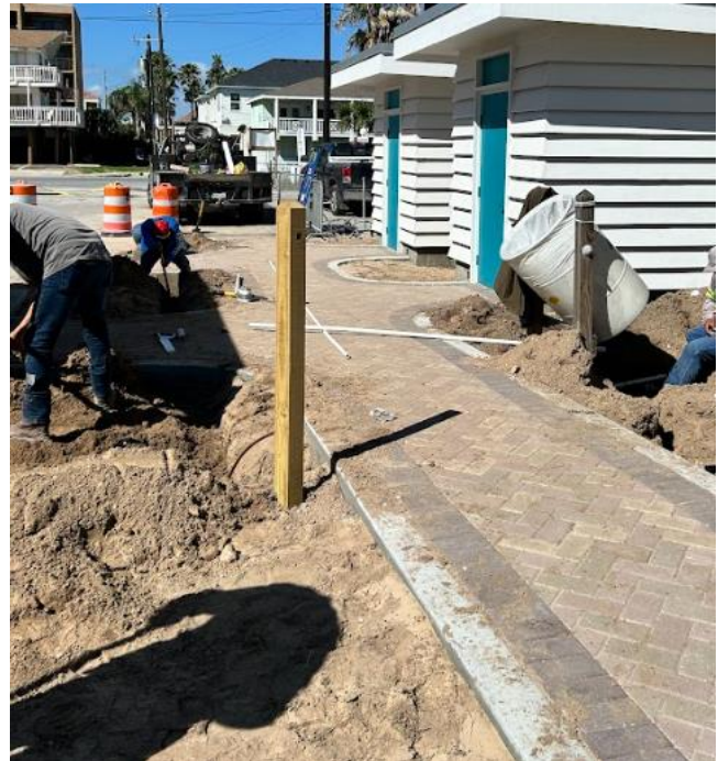
Figure 6. Irrigation Installation (Above)
