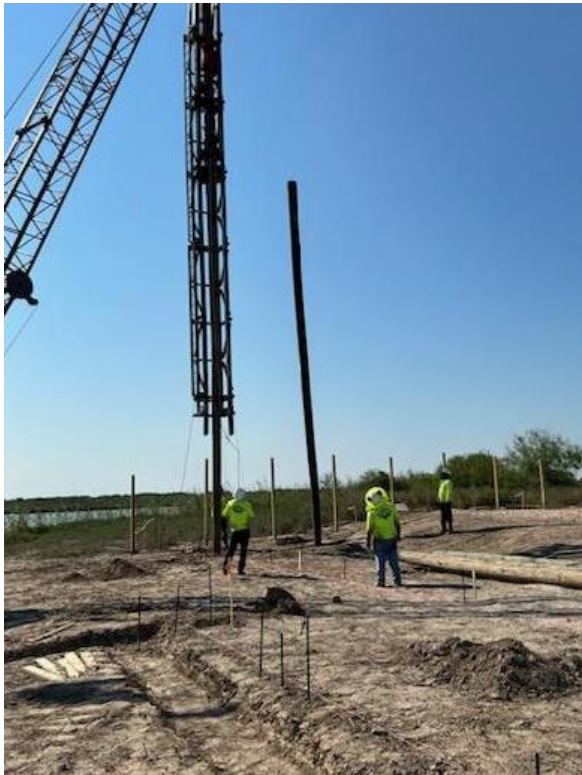
Figure 4. Foundation Pilings
