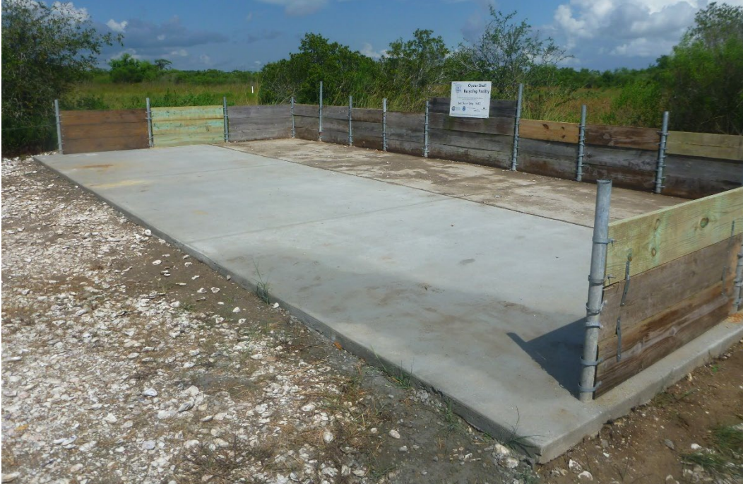
Figure 19. Cement pad at TX City Curing Site.
