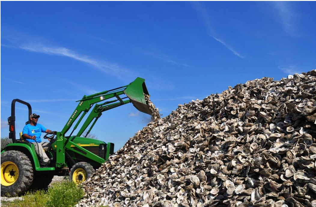
Figure 6. Consolidating a cured shell pile (Phase 3)
