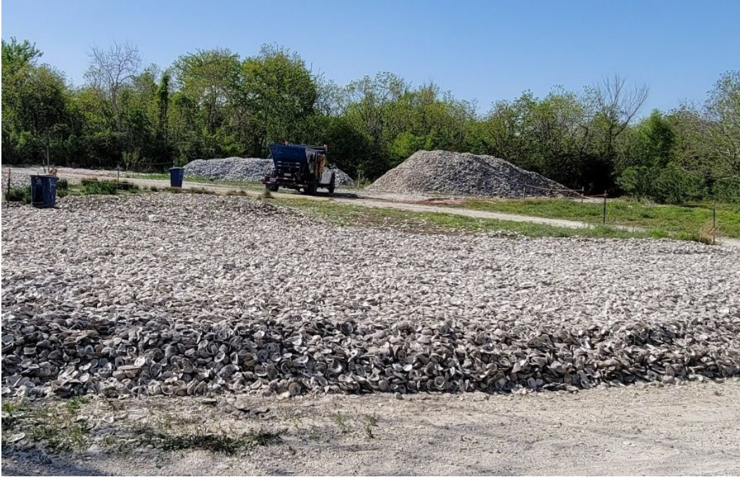
Figure 13. Fully cured shell in the background and partially cured shell that was just rotated in the foreground at Red Bluff curing site.
