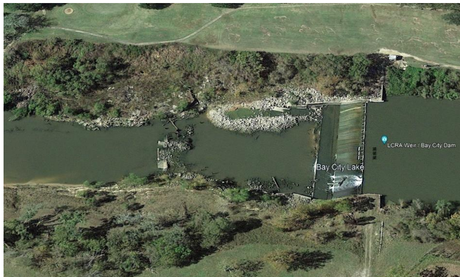
Figure 20 LCRA dam south of Bay City (Source: Google Earth)
