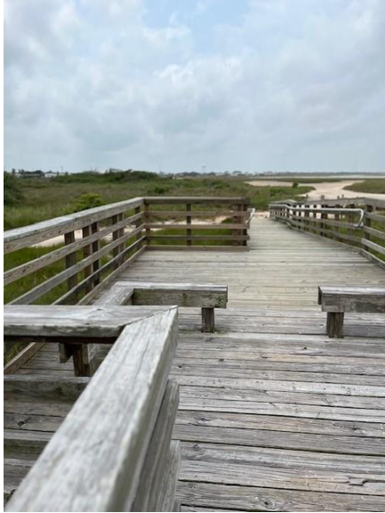
Boardwalk – Before Construction
