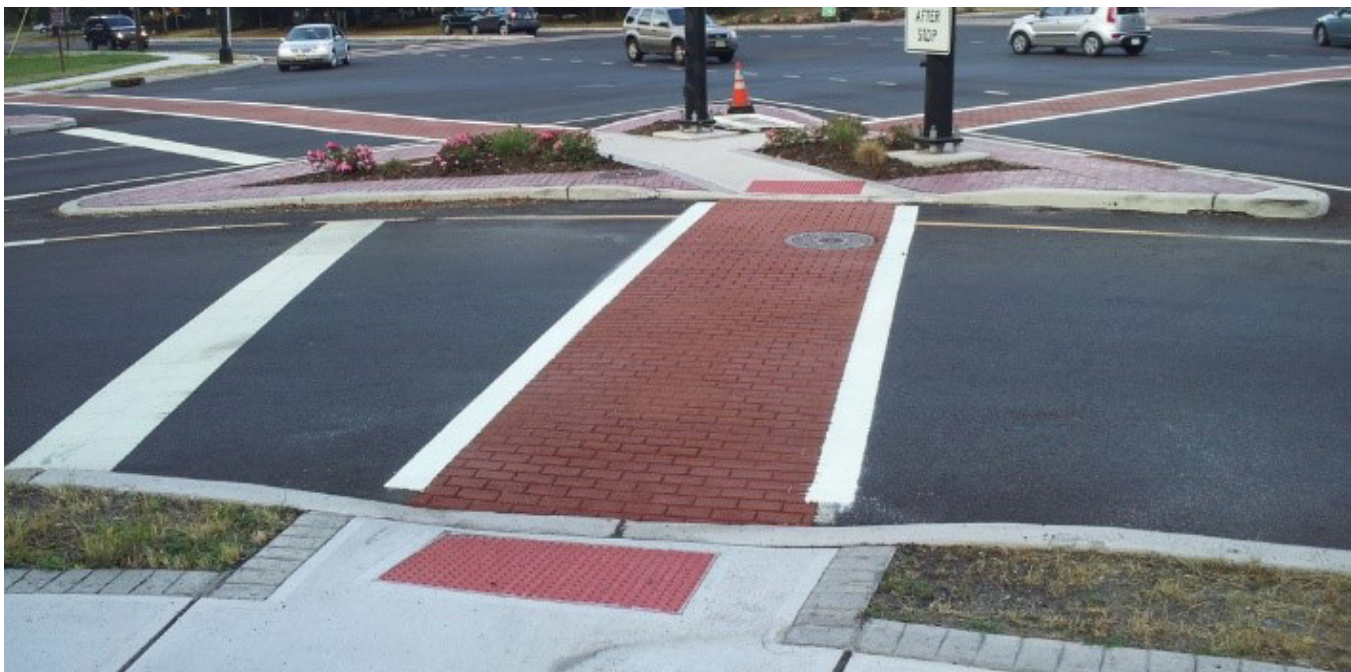
Figure 5-17: Pedestrian crossing constructed with pervious pavers.
