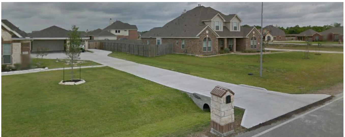
Figure 4-1: Picture of a Typical Swale in a Residential Neighborhood in Chambers County, Texas. (Photo courtesy of Google Earth)
