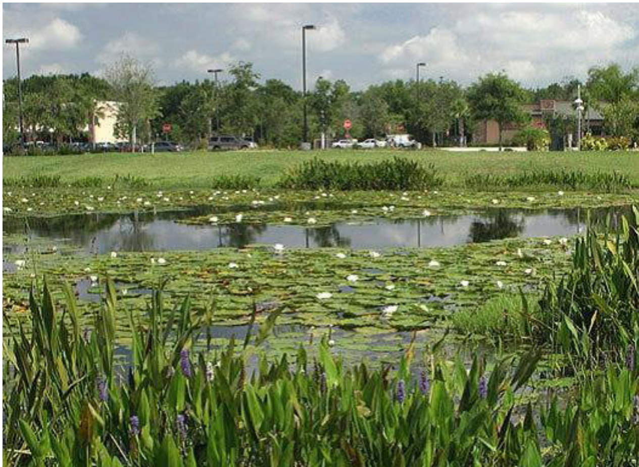
Figure 4-8: Enhanced Detention Wet Pond. (Photo courtesy of Houston Galveston Area Council)
