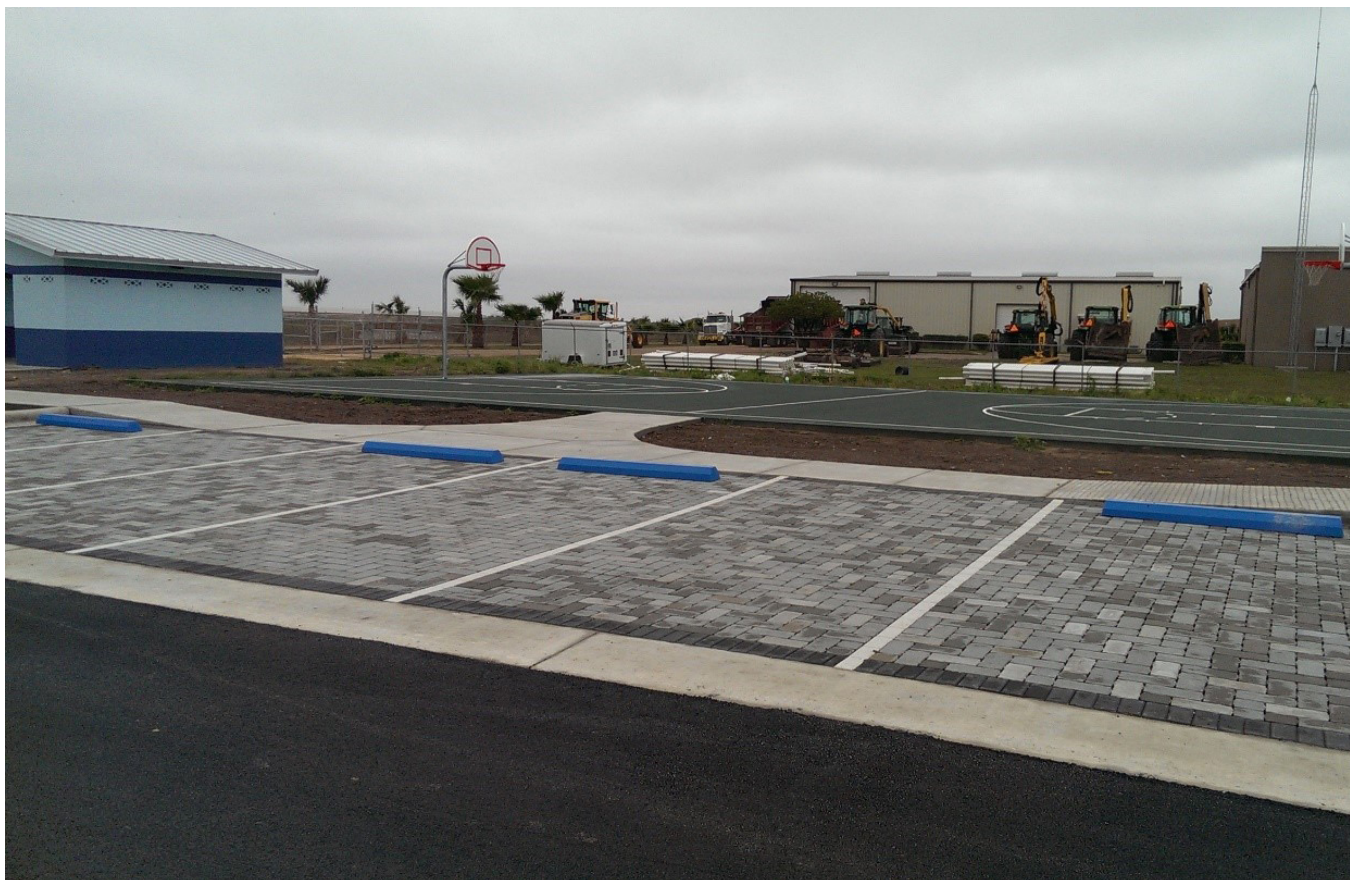
Figure 4-5: Permeable pavers in parking stall of Cascade Park parking lot in Cameron County, Texas. (Photo courtesy of Danica Adams)
