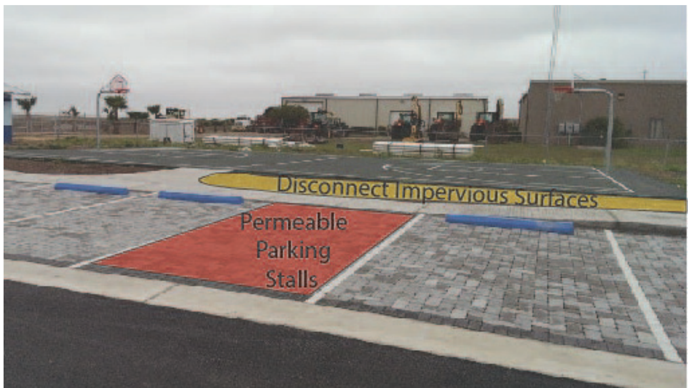
Figure 5-13: Permeable Interlocking Concrete Pavers with regular asphalt driving lane in Cascade Park parking lot, Cameron County, Texas.
