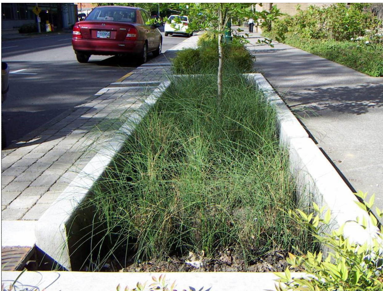
Figure 5-14: Bioretention serves as a buffer between the sidewalk and street. (Photo courtesy of State of Washington Transportation Improvement Board)
