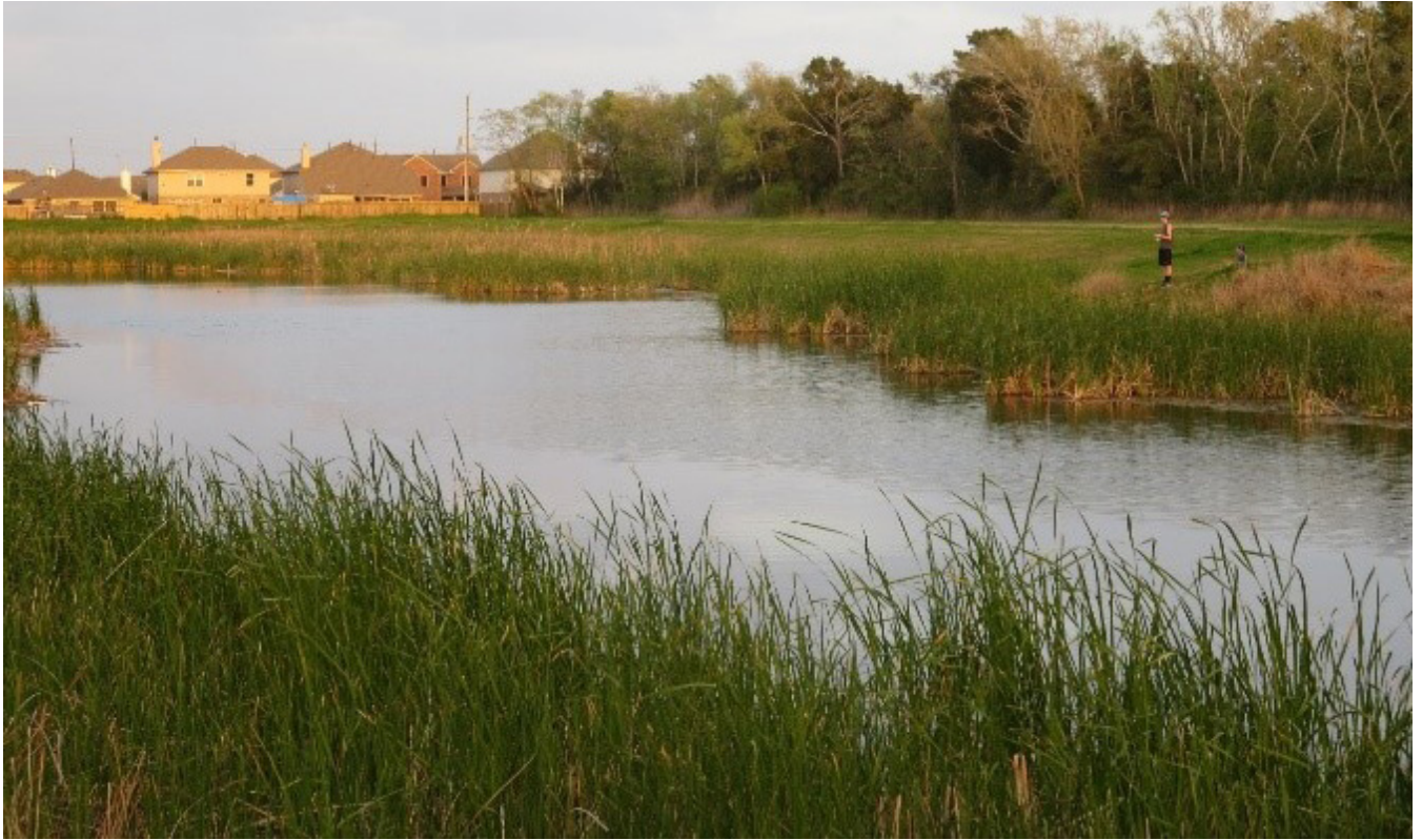
Figure 5-2: Enhanced detention wet pond is an amenity in a subdivision in Chambers County, Texas.
