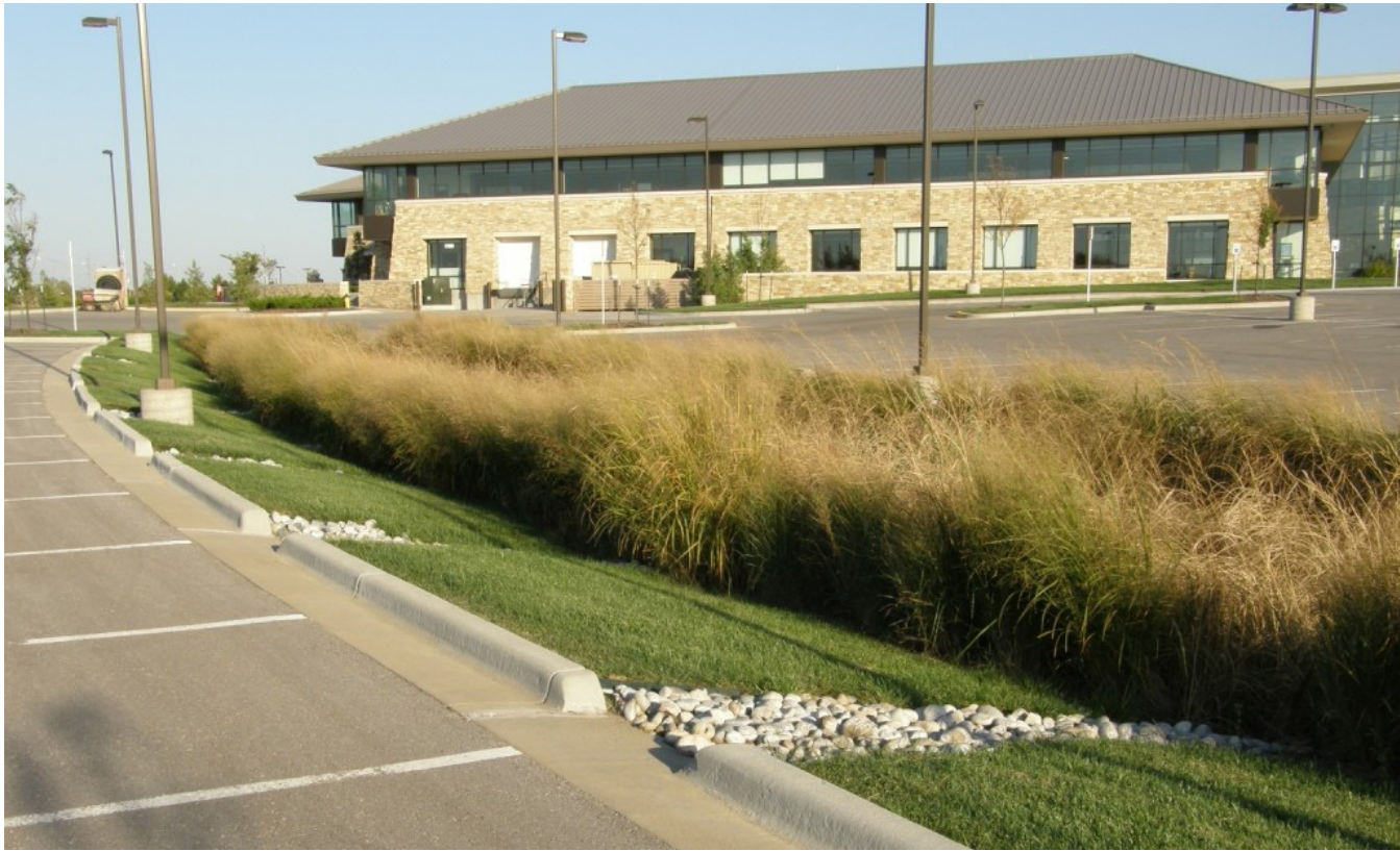
Figure 4-11: Picture of a Bioretention Facility. (Photo courtesy of David Dods)
