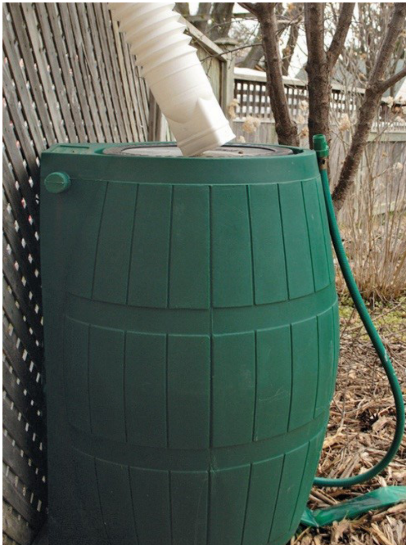
Figure 2-5: Residential rain barrel. (Photo courtesy of TCEQ)
