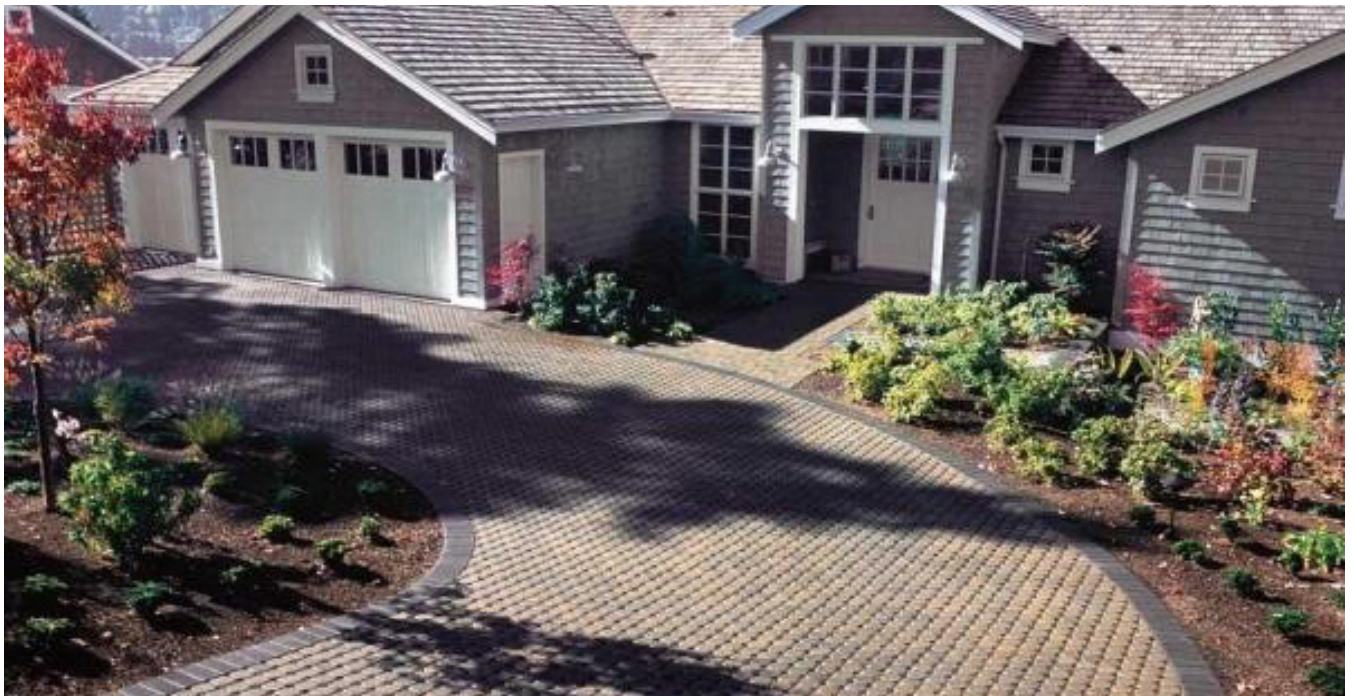
Figure 5-7: Driveway constructed of permeable pavers. (Photo courtesy of Mutual Materials)
