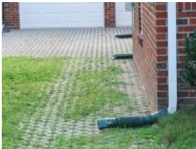
Figure 3-5: Downspouts directed to permeable pavement on driveway. (Photo courtesy of Montgomery County, Maryland)
