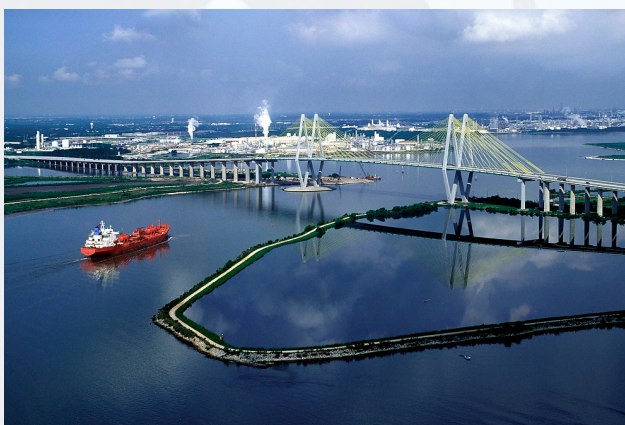
Fred Hartman Bridge Photo By: Jim Olive
