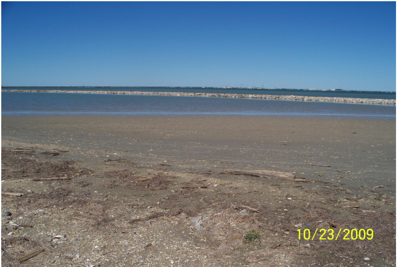
Photo Station 5. Post-construction. Mid and eastern sections of completed breakwater.
