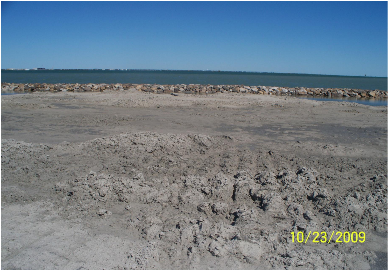
Photo Station 3. Post-construction. View north toward Ship Channel and Redfish Bay, Texas with completed breakwater and shoreline nourishment.
