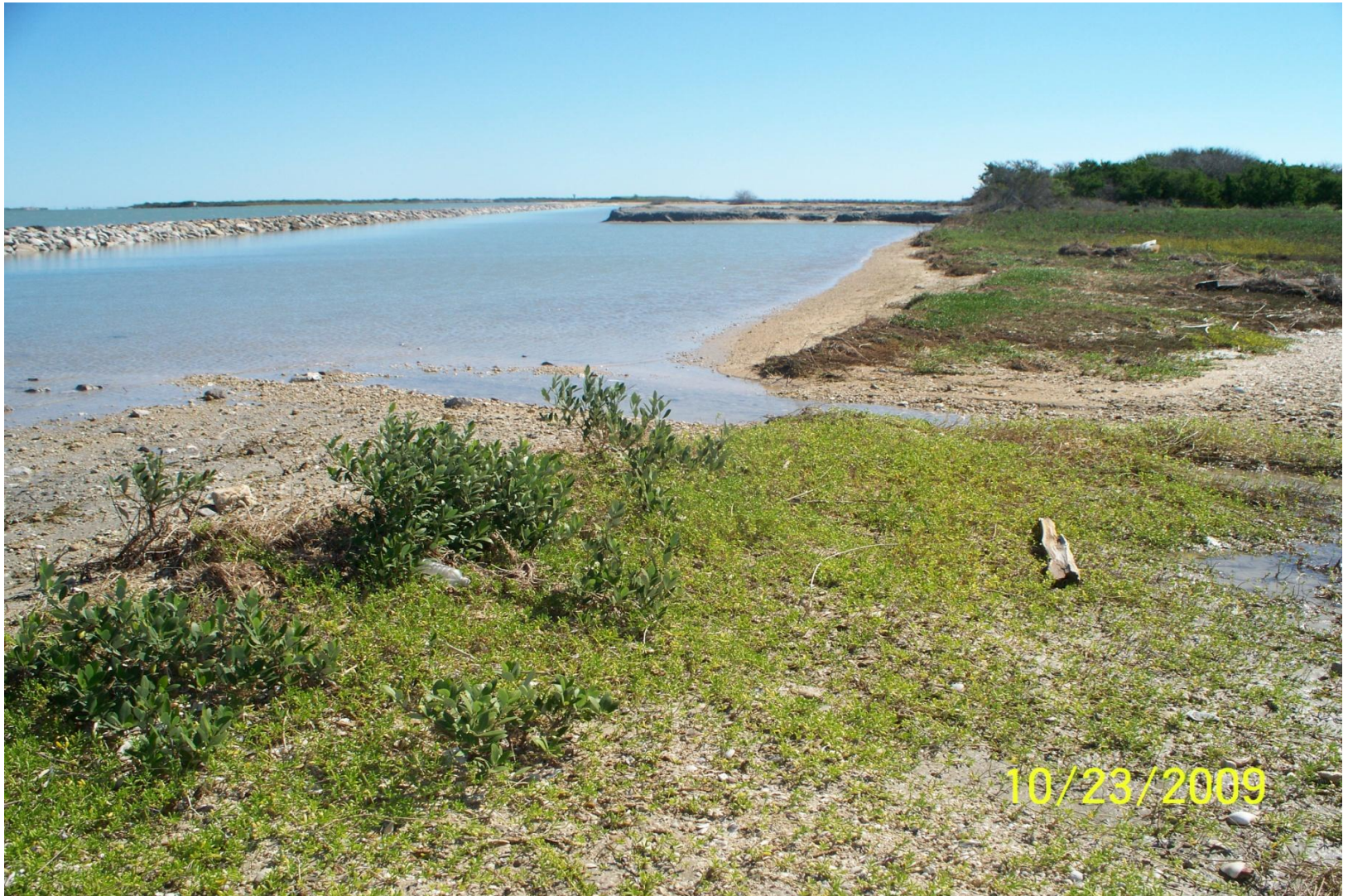
Photo Station 2. Post-construction . Note erosion between July 2009 photo and breakwater completion. Shoreline nourishment in mid distance .
