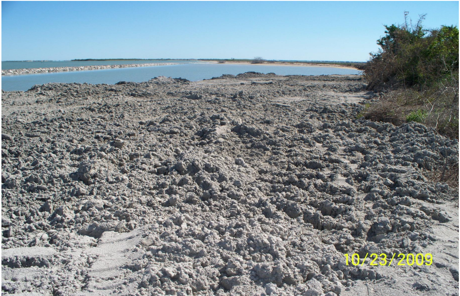
Photo Station 3. Post -construction. Shoreline nourishment and breakwater. Note erosion between pre-construction and completion of project.
