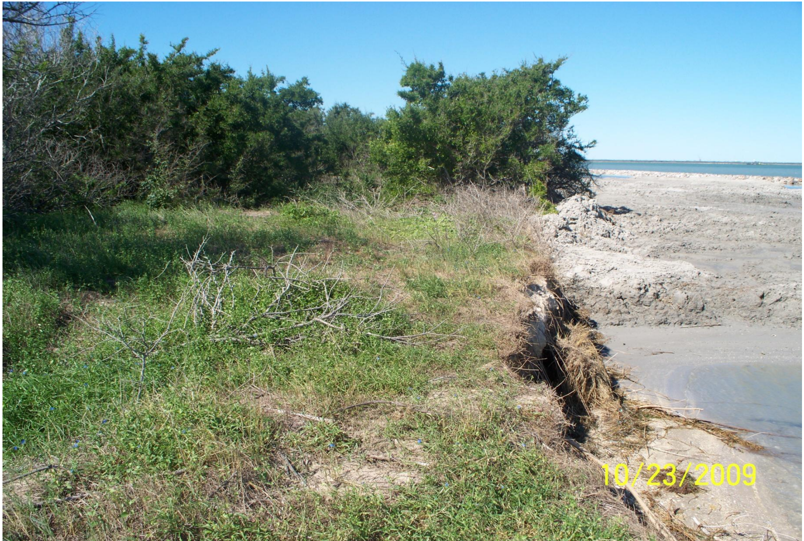
Photo Station 4. Post-construction. View west with shoreline nourishment .
