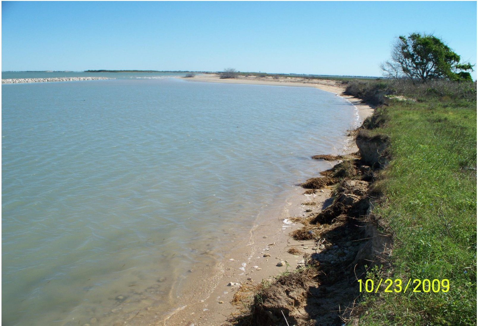
Photo Station 4. Post-construction. East portion of completed breakwater.
