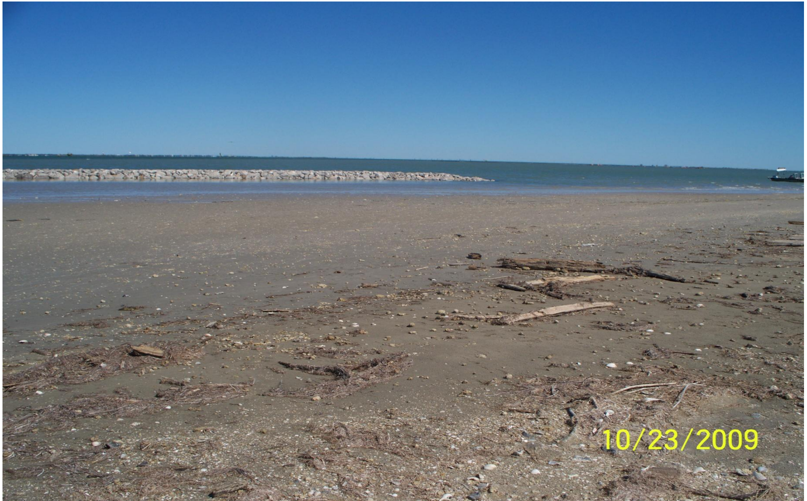
Photo Station 5. Post-construction. East end of and completed breakwater, 1 of 2.
