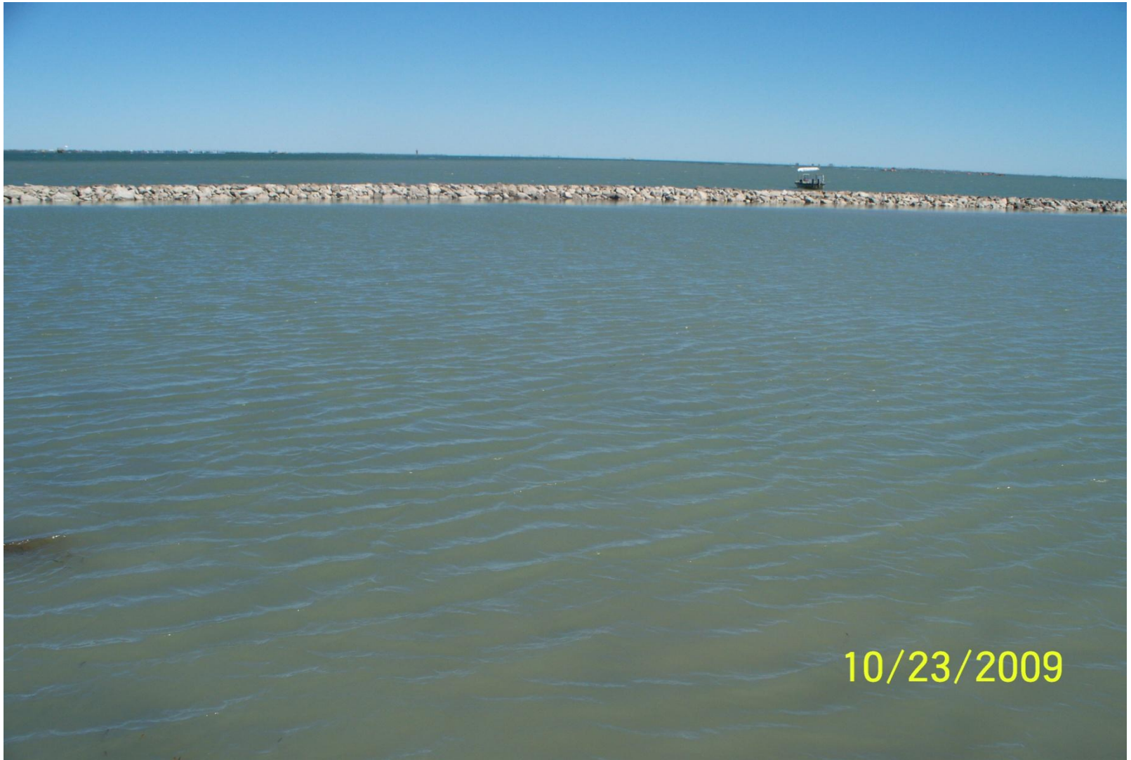
Photo Station 4. Post-construction. Completed breakwater.
