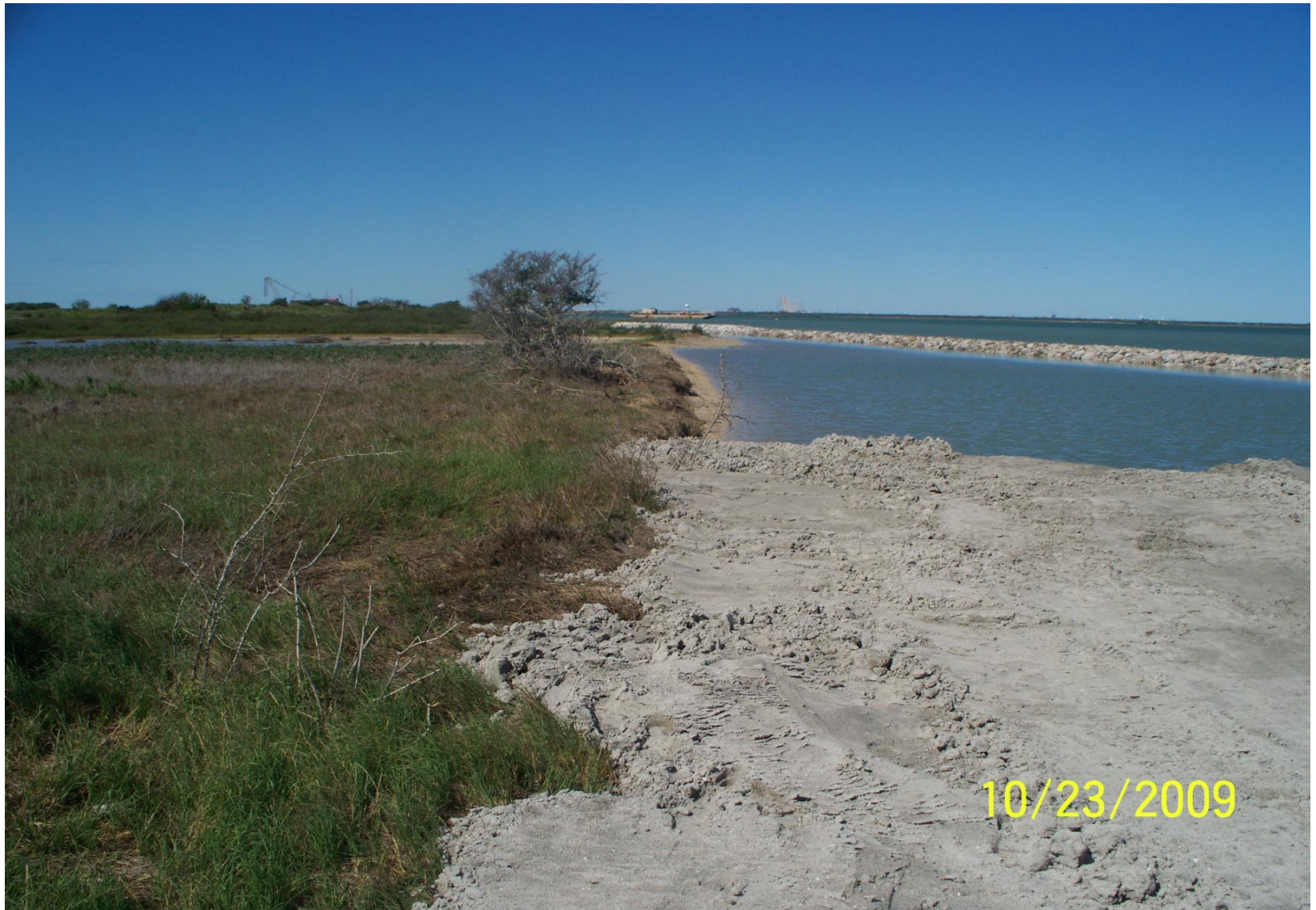
Photo Station 3. Post-construction . Note erosion between July 2009 and project completion. Shoreline nourishment in foreground.
