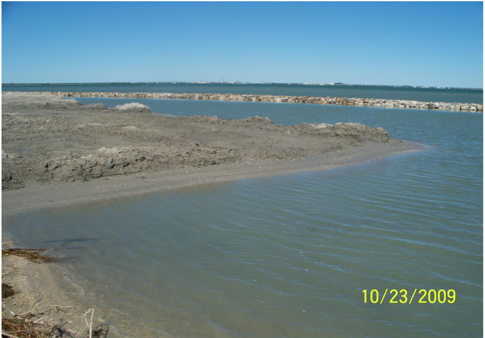
Photo Station 4. Post-construction. East portion of shoreline nourishment and completed breakwater.
