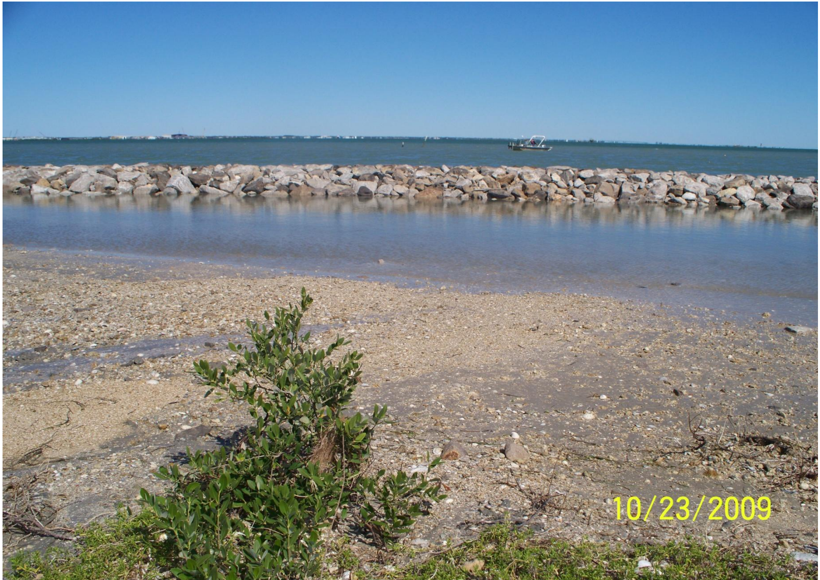
Photo Station 2. Post-construction . Note erosion up to mangrove between pre-construction photo and breakwater completion.
