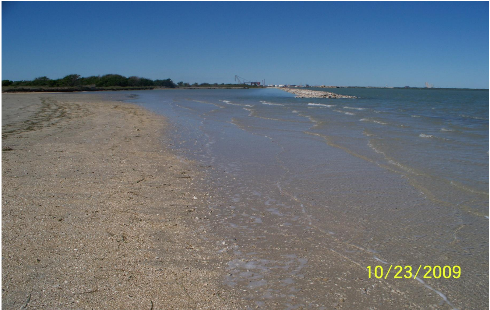
Miscellaneous Post Construction photo of far east end radial head looking westward behind completed breakwater, 10/23/2009.
