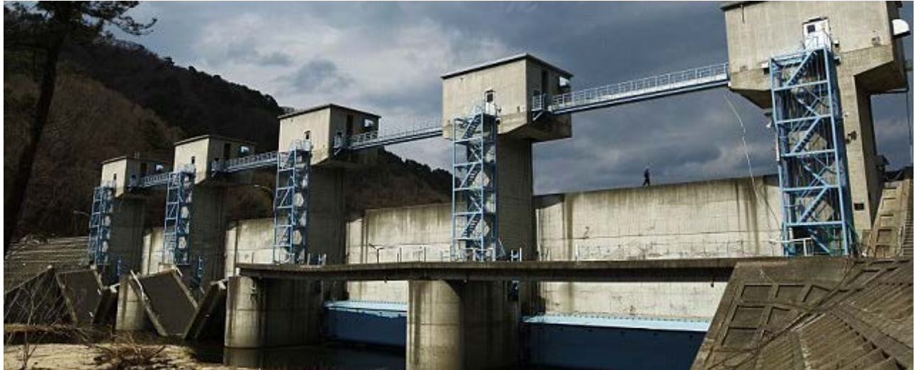
Figure 43 - Fudai Flood Gate
