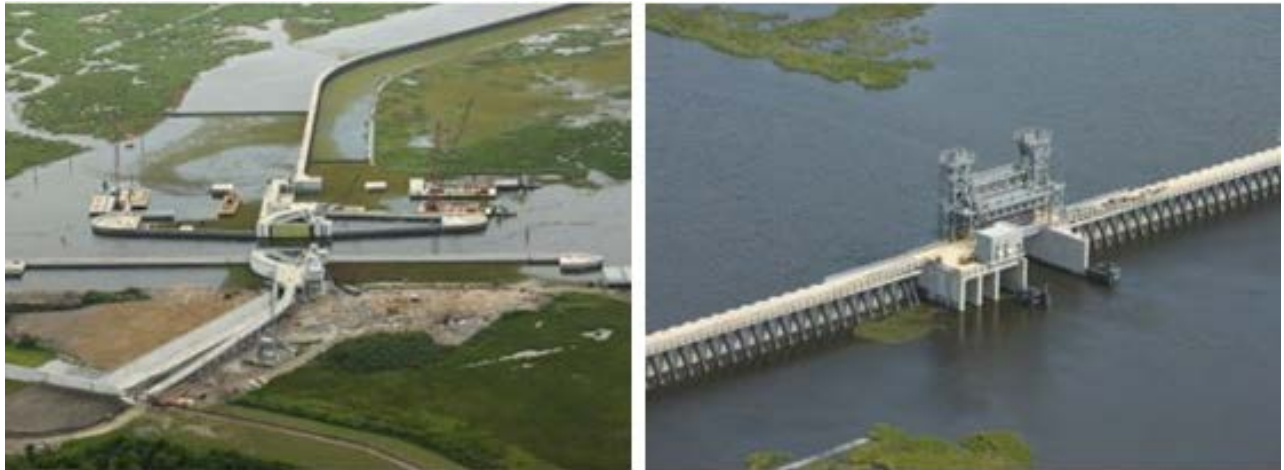
Figure 55 - (a) Sector Gate & Barge Gate, (b) Bayou Bienvenue Vertical Lift Gate
