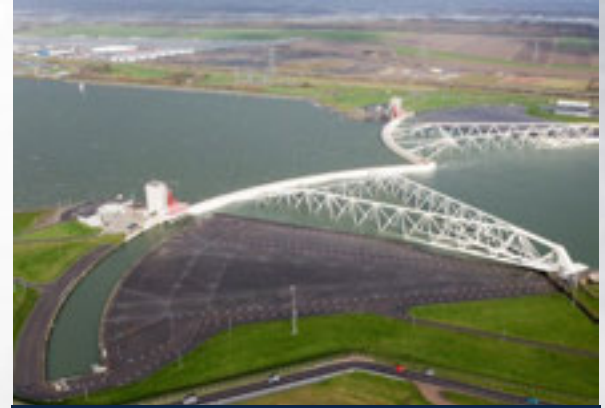
Storm Surge Barrier, Maeslantkering, Netherlands
