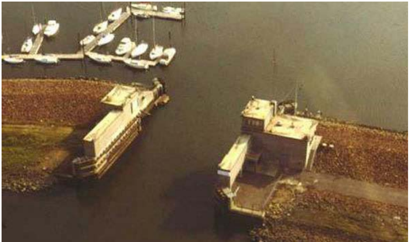
Figure 57 - Stamford Hurricane Barrier
