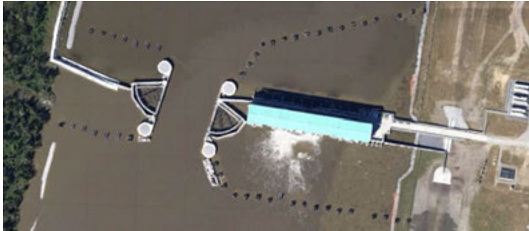
Figure 58 - GIWW West Closure Complex
