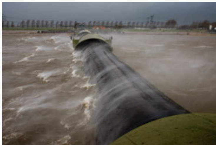
Figure 37 -Inflatable Rubber Dam
