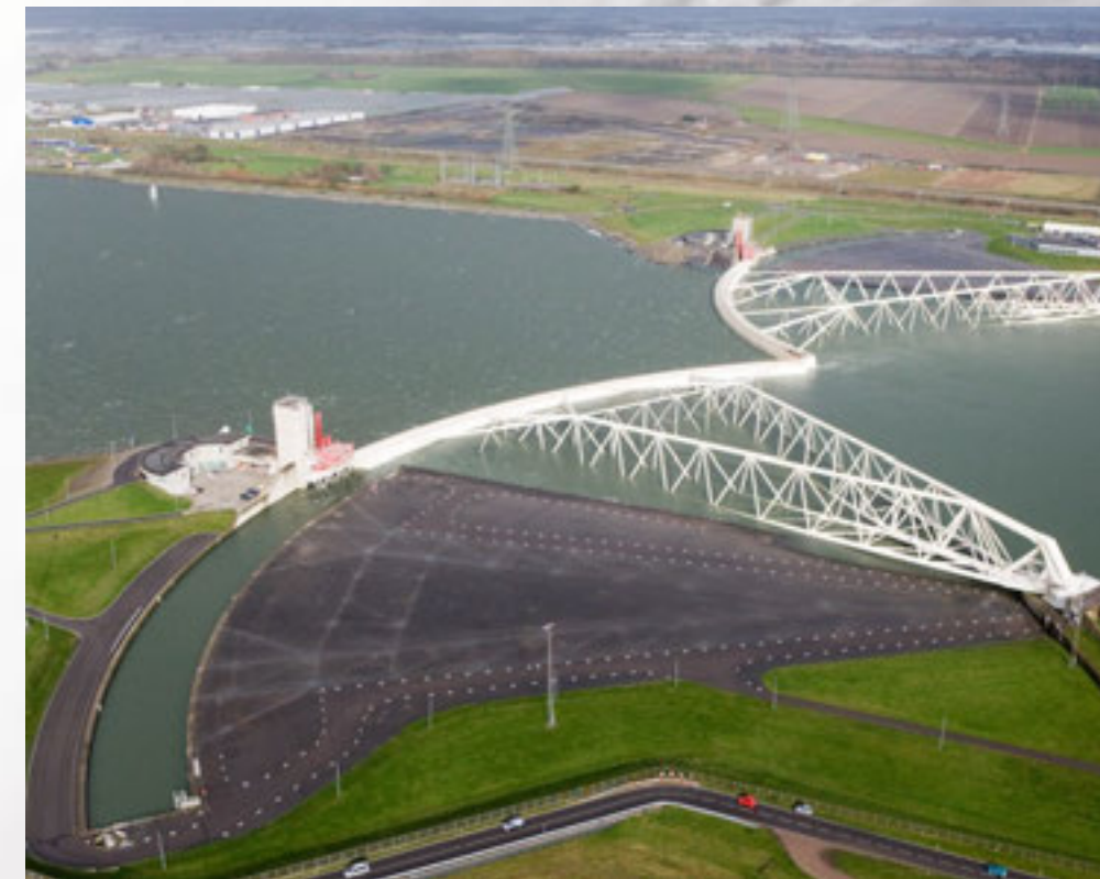
Storm Surge Barrier, Maeslantkering, Netherlands
