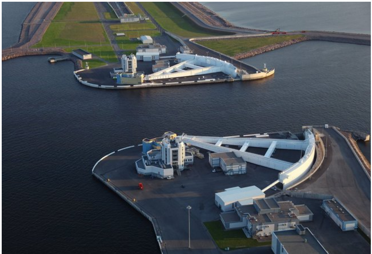
Figure 49 - St. Petersburg Dam
