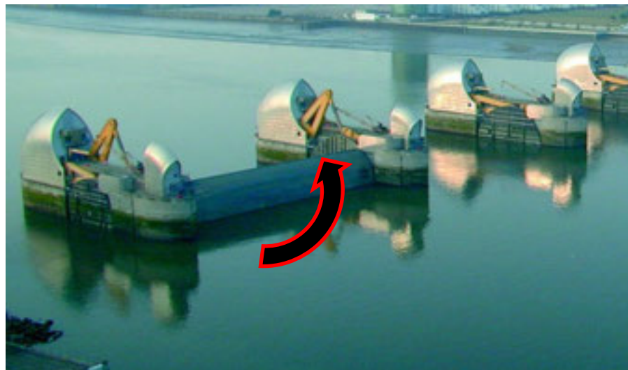
Figure 33 - Vertical Rotating Gate
