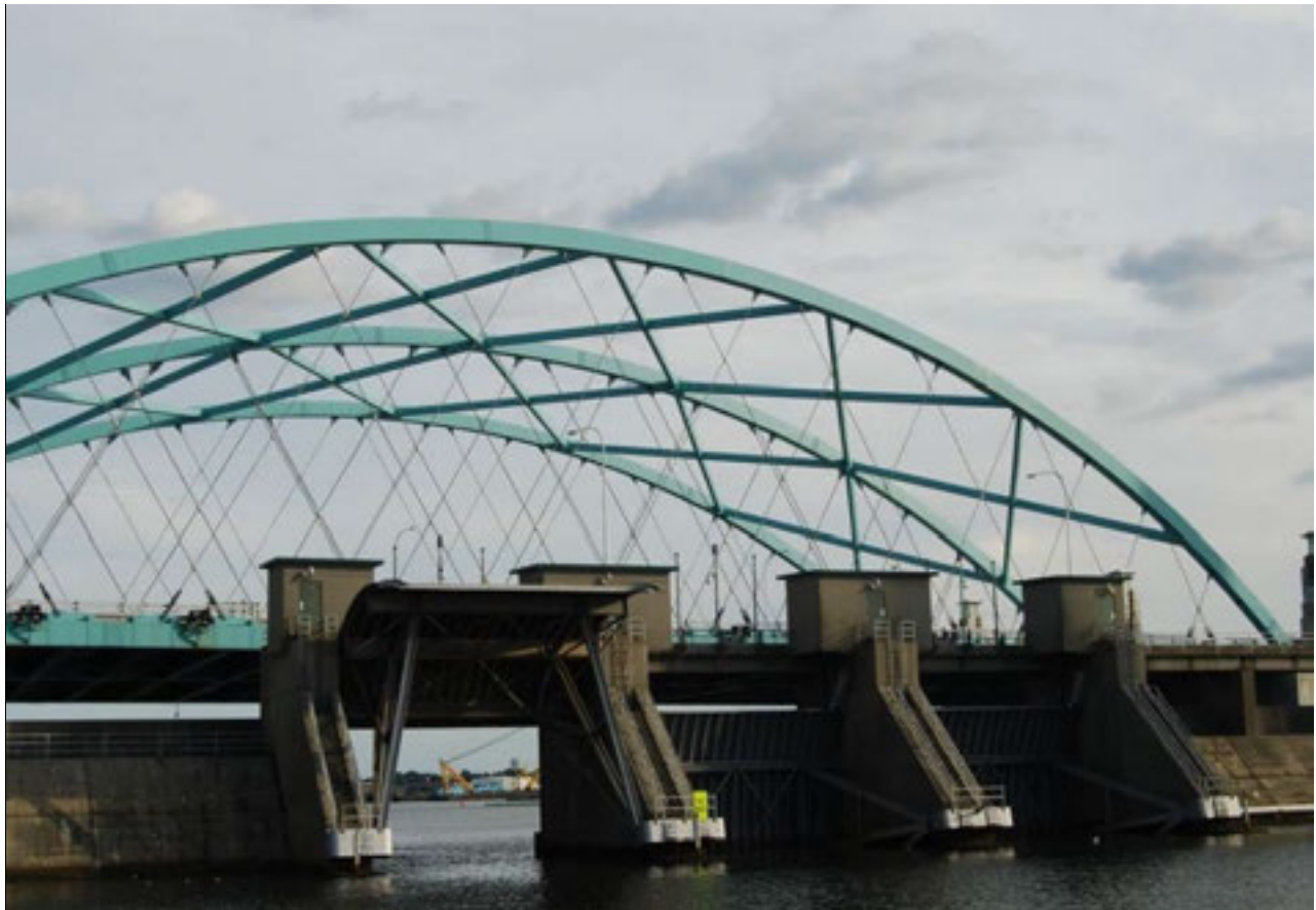
Figure 56 - Foxpoint Hurricane Barrier
