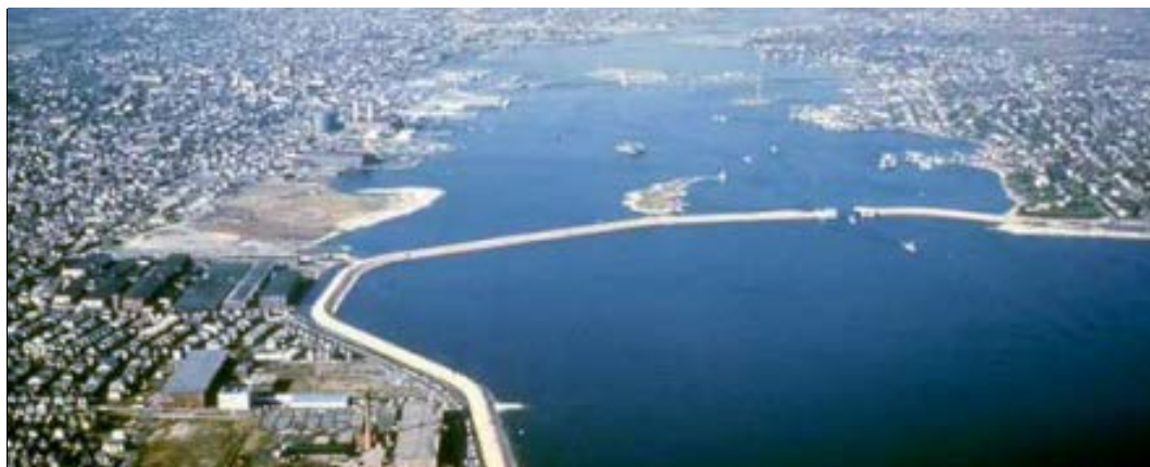
Figure 59 - New Bedford Hurricane Protection Barrier
