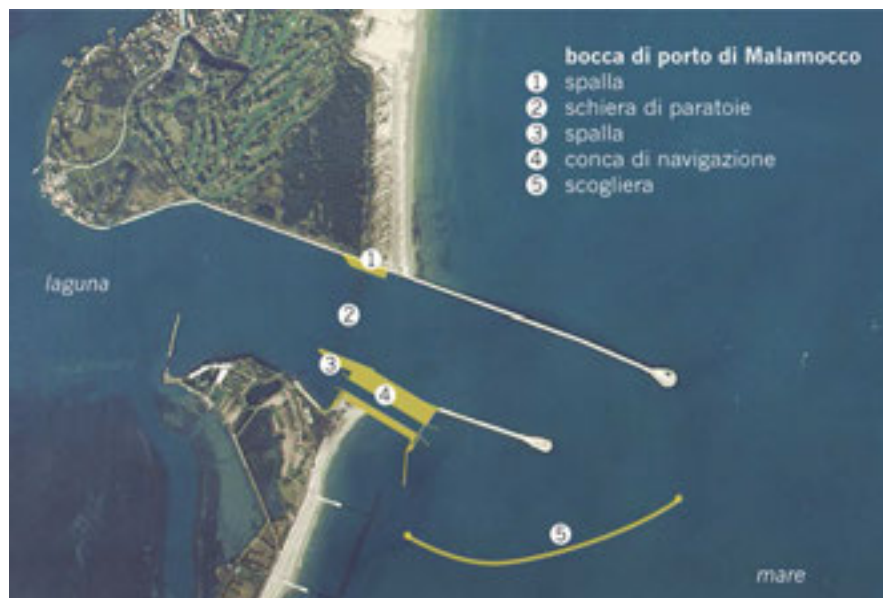
Figure 51 - Malamocco Inlet Barrier
