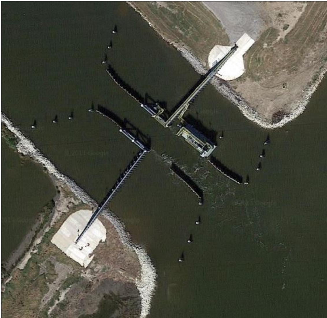
Figure 60 - Bush Canal Floodgate
