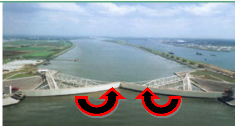
Figure 34 - Floating Sector Gate
