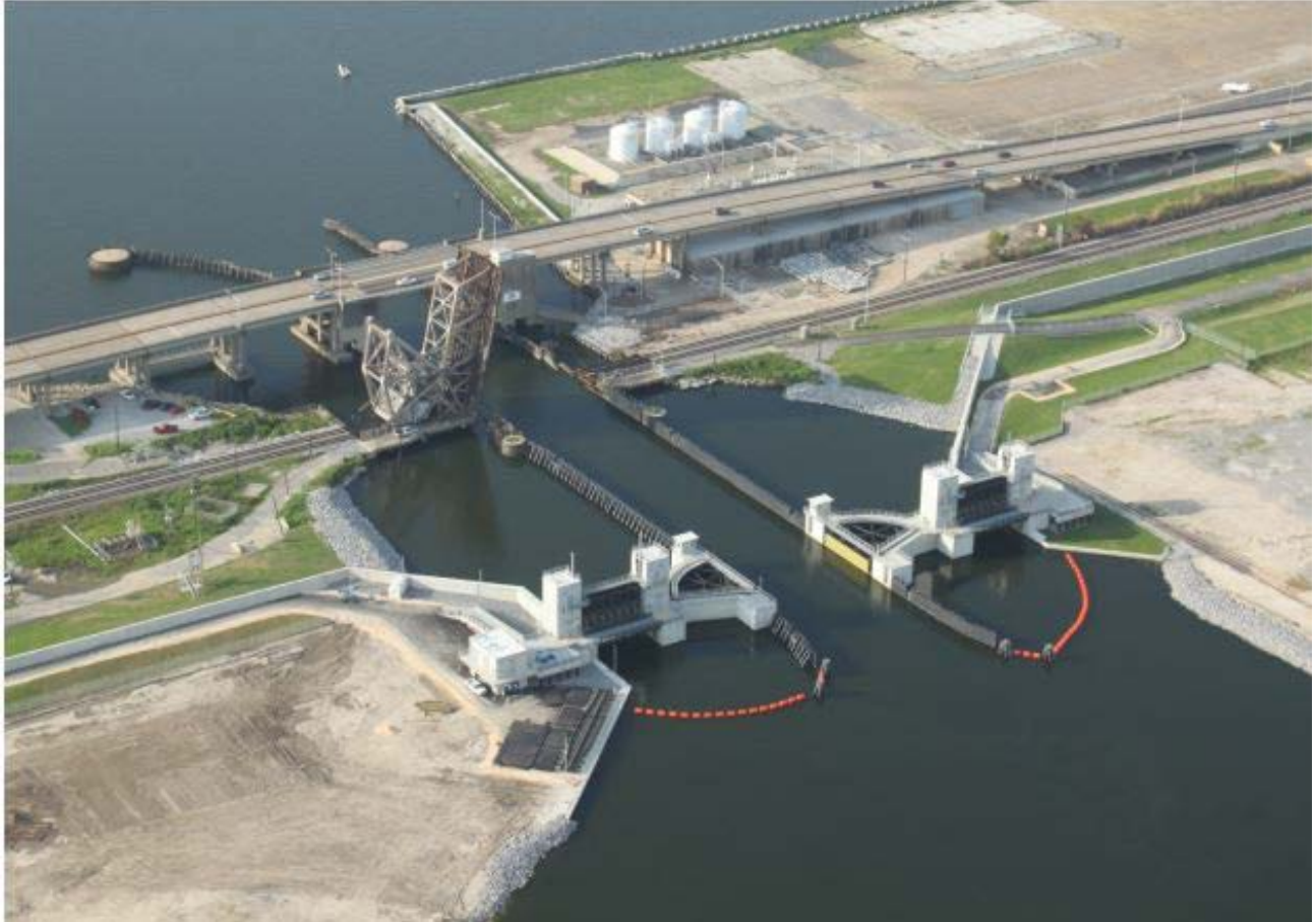
Figure 54 - Seabrook Floodgate Complex
