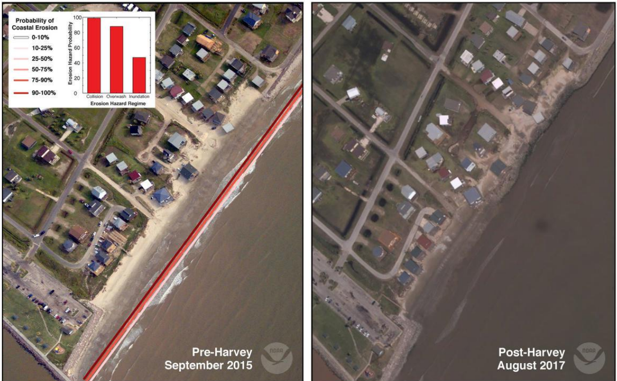
Figure 9-38: Surfside Beach Pre- and Post-Harvey
